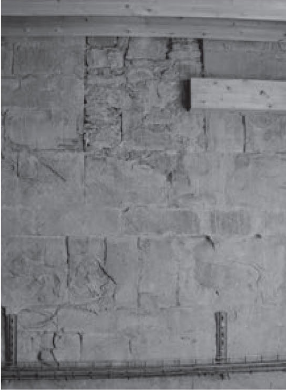
Fig. 7. Jaca Cathedral, window over the modern vault of the north aisle (photo author)
