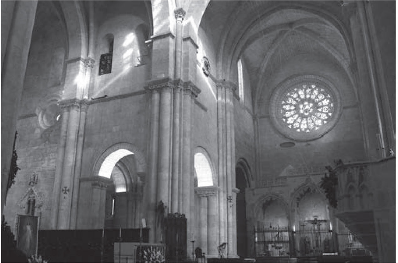
Fig. 7. South transept and southern lateral apse, with double columns on each pillar, c. 1175–90 (photo Marta SERRANO COLL)
