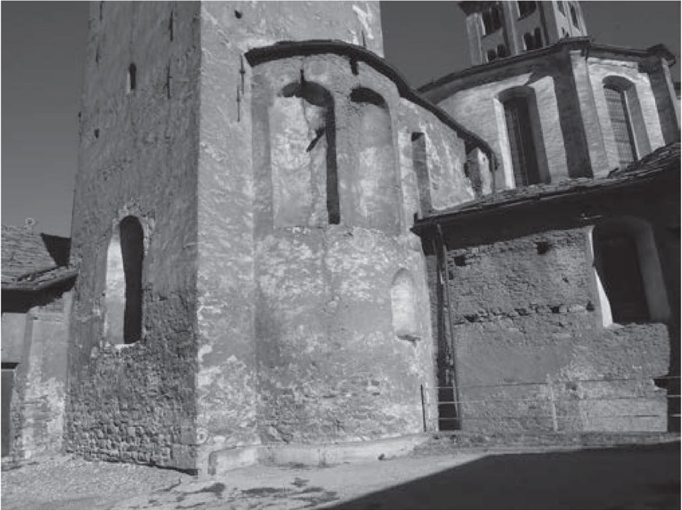
Fig. 6. Aosta Cathedral, the elevated chapel of the southern bell tower, seen from the exterior (photo Renato PERINETTI)
