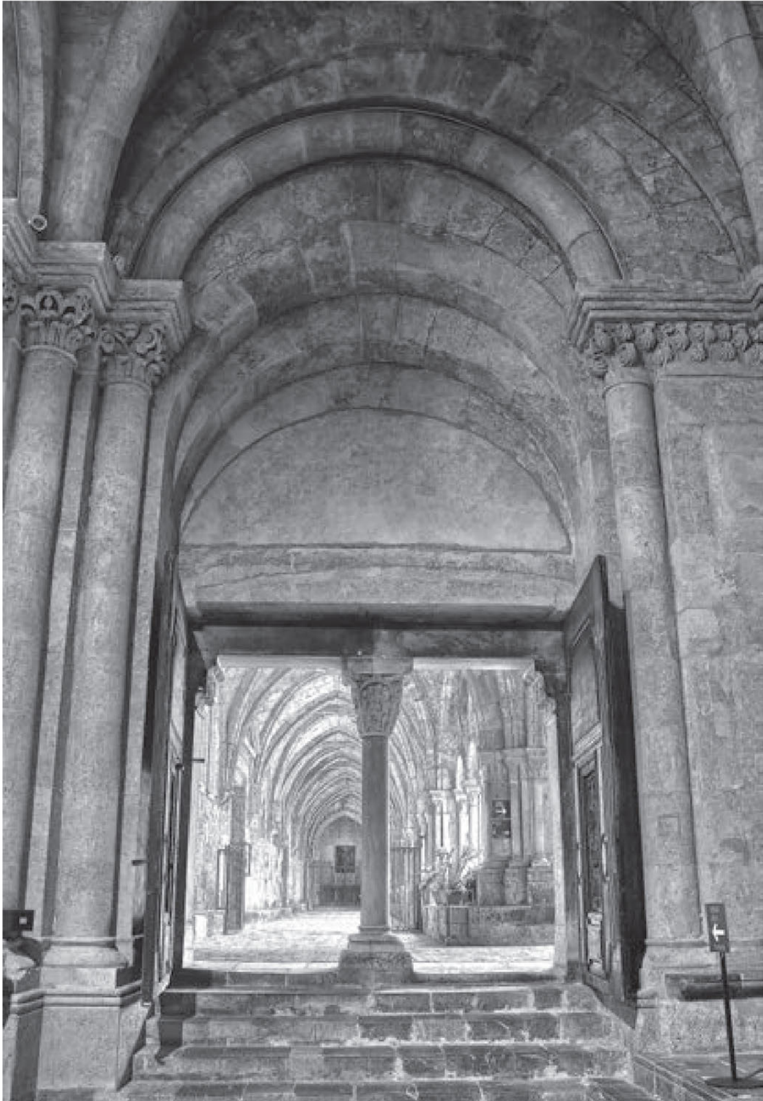
Fig. 2b. Monumental marble doorway connecting the church and cloister, c. 1175: exterior view (photo Roberto CHAVERRI BERGUÉ & Elena ARANDA VÁZQUEZ)
