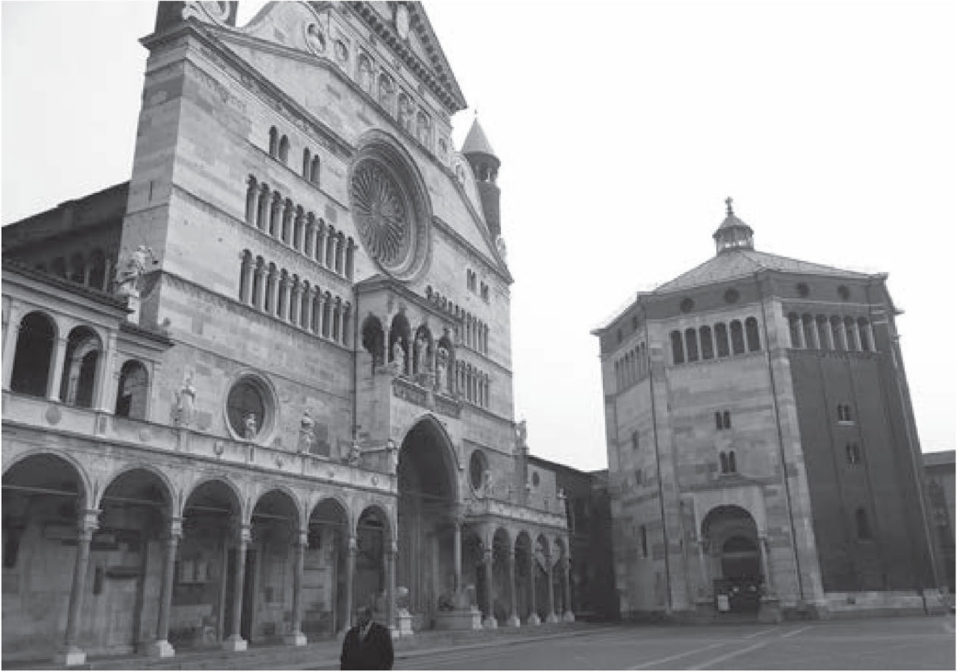
Fig. 5. Cremona Cathedral, view of the façade and baptistery (photo author)
