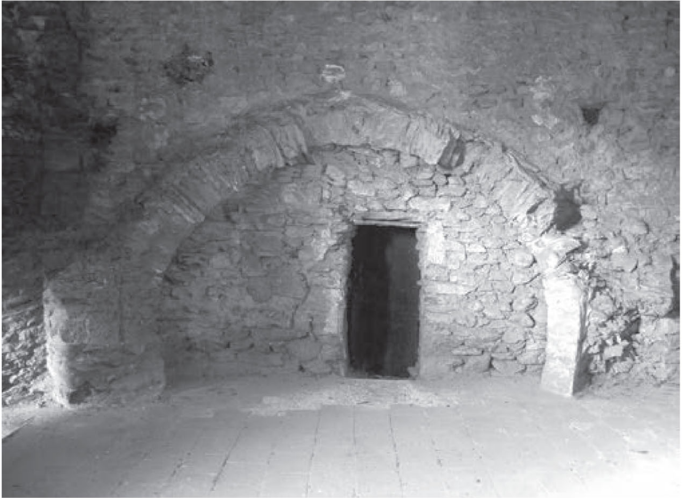
Fig. 5. Aosta Cathedral, remains of the elevated chapel in the northern bell tower (photo Mauro CORTELAZZO)
