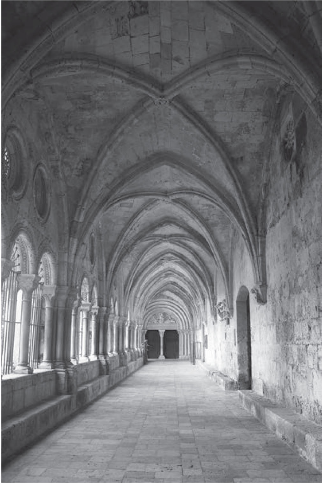
Fig. 9. Walkway in the cloister, with corner and intermediate pillars (c. 1190–95) and ribbed vaults on corbels (c. 1215) (photo MARTA SERRANO COLL)
