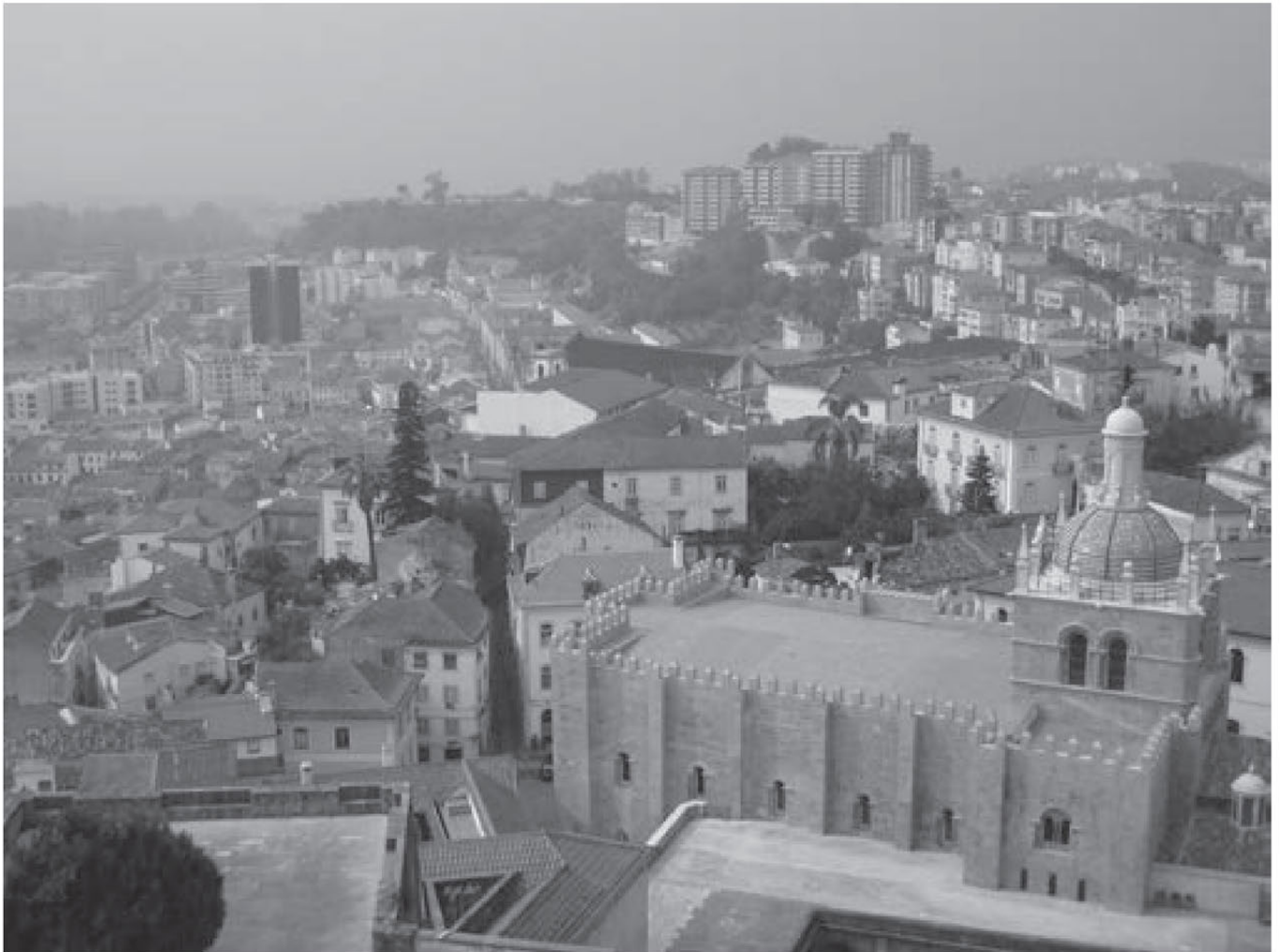
Fig. 2. Coimbra Cathedral, exterior view (photo Wikimedia commons)
