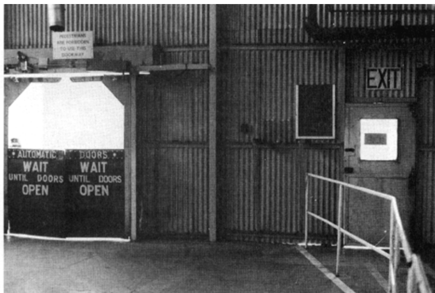
Figure 3.17 Separation of truck and pedestrian gangways
