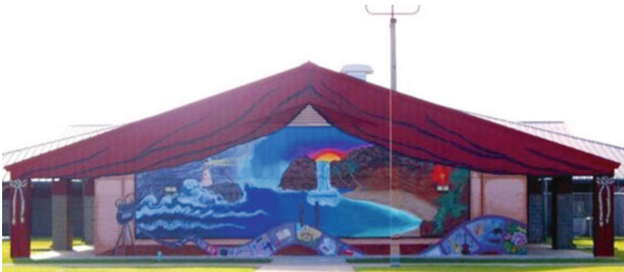
Fig. 5.8 Beacon of Hope: mural completed by female prison inmates on a building at the Gadsden Correctional Institution (GCI)
