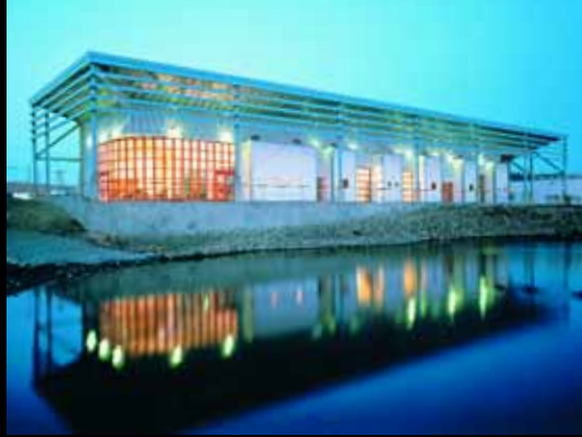
MARINE TECHNOLOGY FACILITY, SEATTLE CENTRAL COMMUNITY COLLEGE, SEATTLE, WASHINGTON 1987
