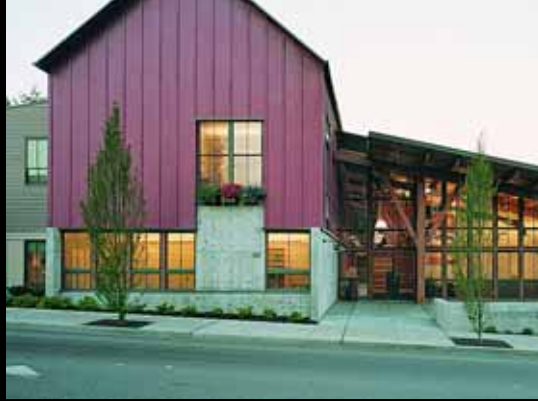
BAINBRIDGE ISLAND CITY HALL, BAINBRIDGE ISLAND, WASHINGTON, 2000
