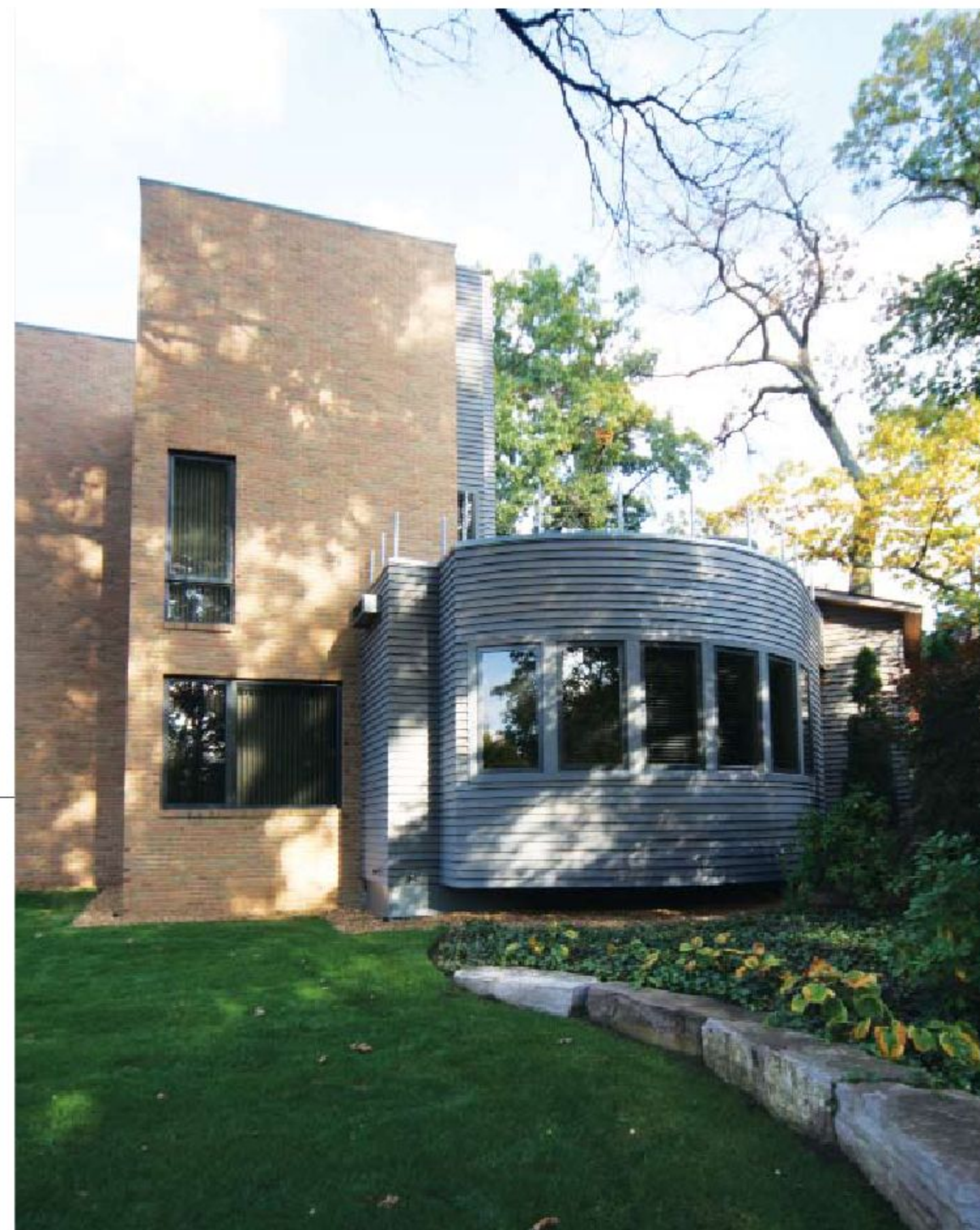
ABOVE: The one-story, curved cedar siding element comprises an office-study with a continuous ribbon of windows. Photograph by Robert Saarinen Swanson
