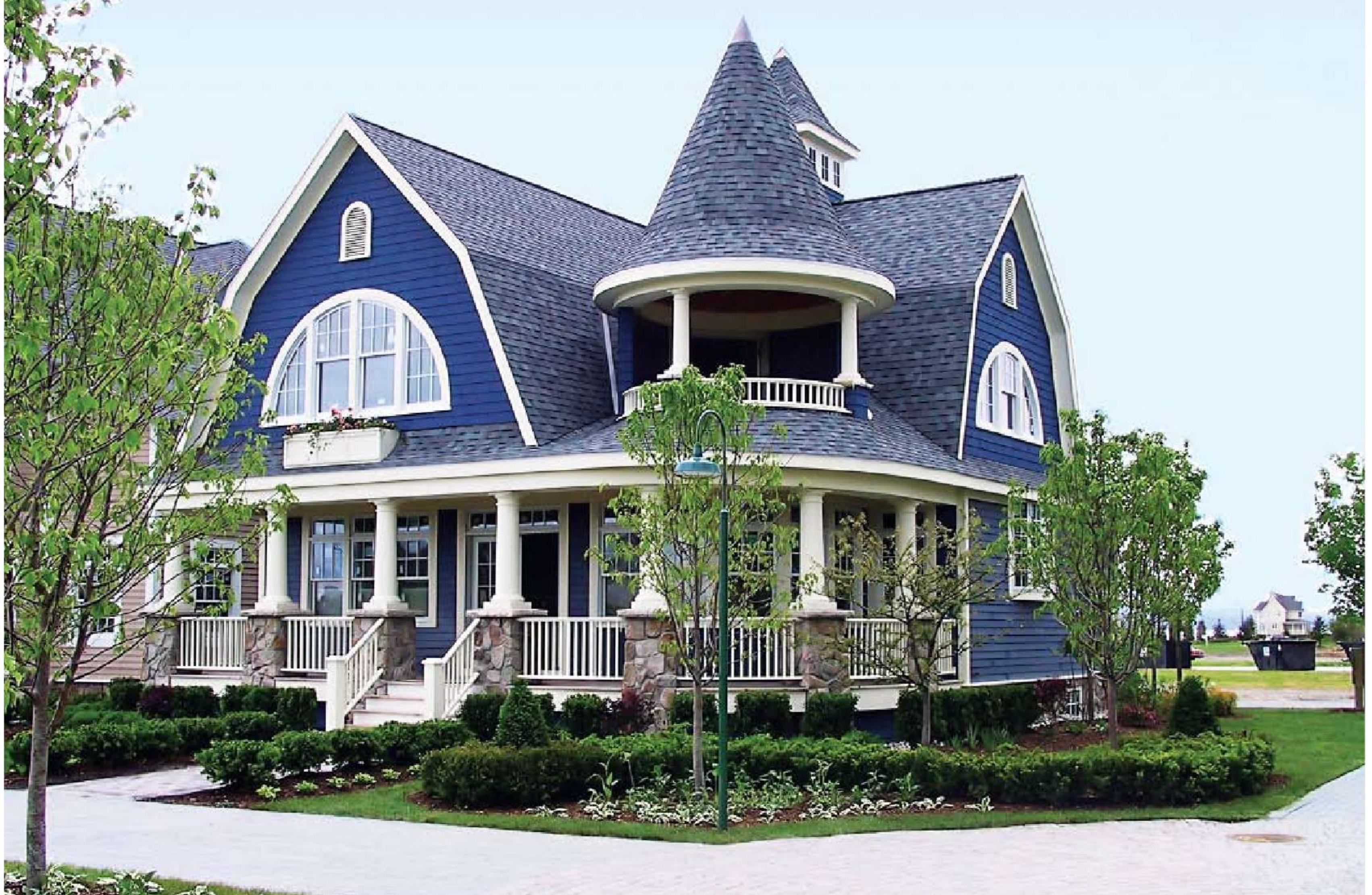
ABOVE: This quaint Victorian graces the village in Bay Harbor near Petoskey. Photograph by N.J. White
