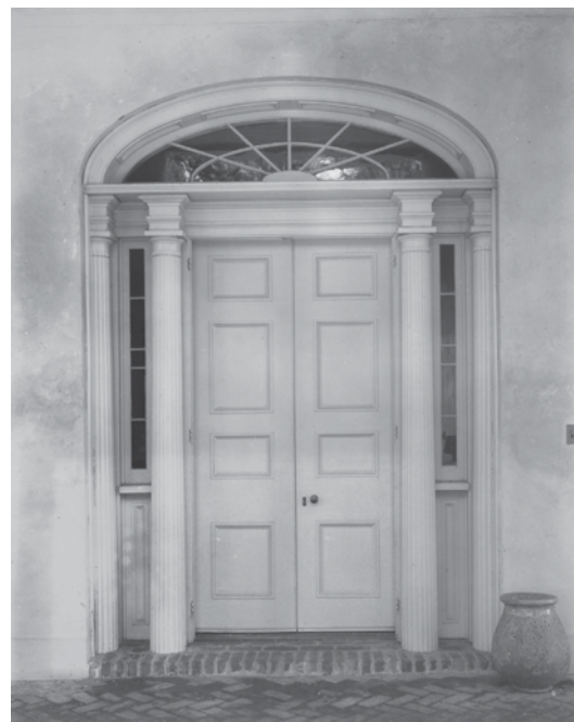
Oak Alley Plantation (front doorway with columns, side-lights, and a fanlight transom), vintage gelatin silver print, Louisiana State Museum, 1956.087.083b
