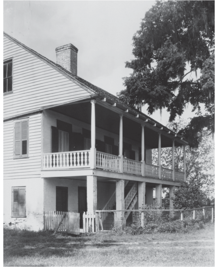
Pleasant View Plantation (three-quarter view including gallery and staircase), gelatin silver print, Louisiana State Museum, 1956.087.212
