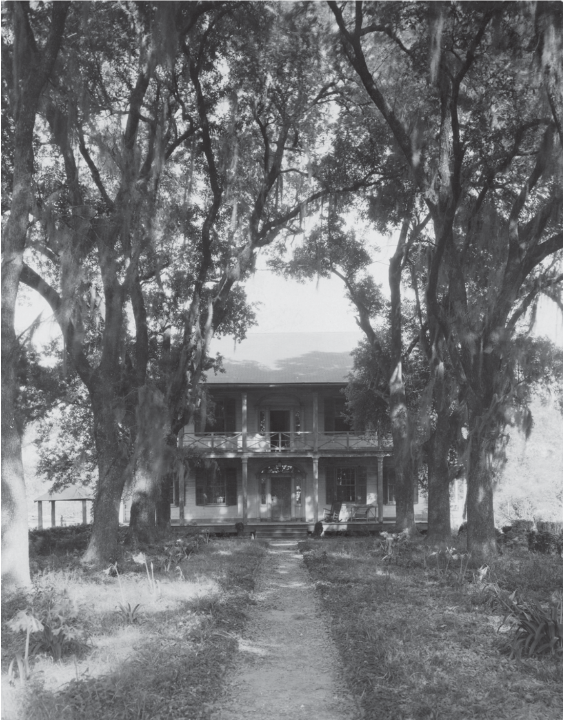
Waverly Plantation (front elevation from a distance), vintage gelatin silver print, Louisiana State Museum, 1956.087.121b
