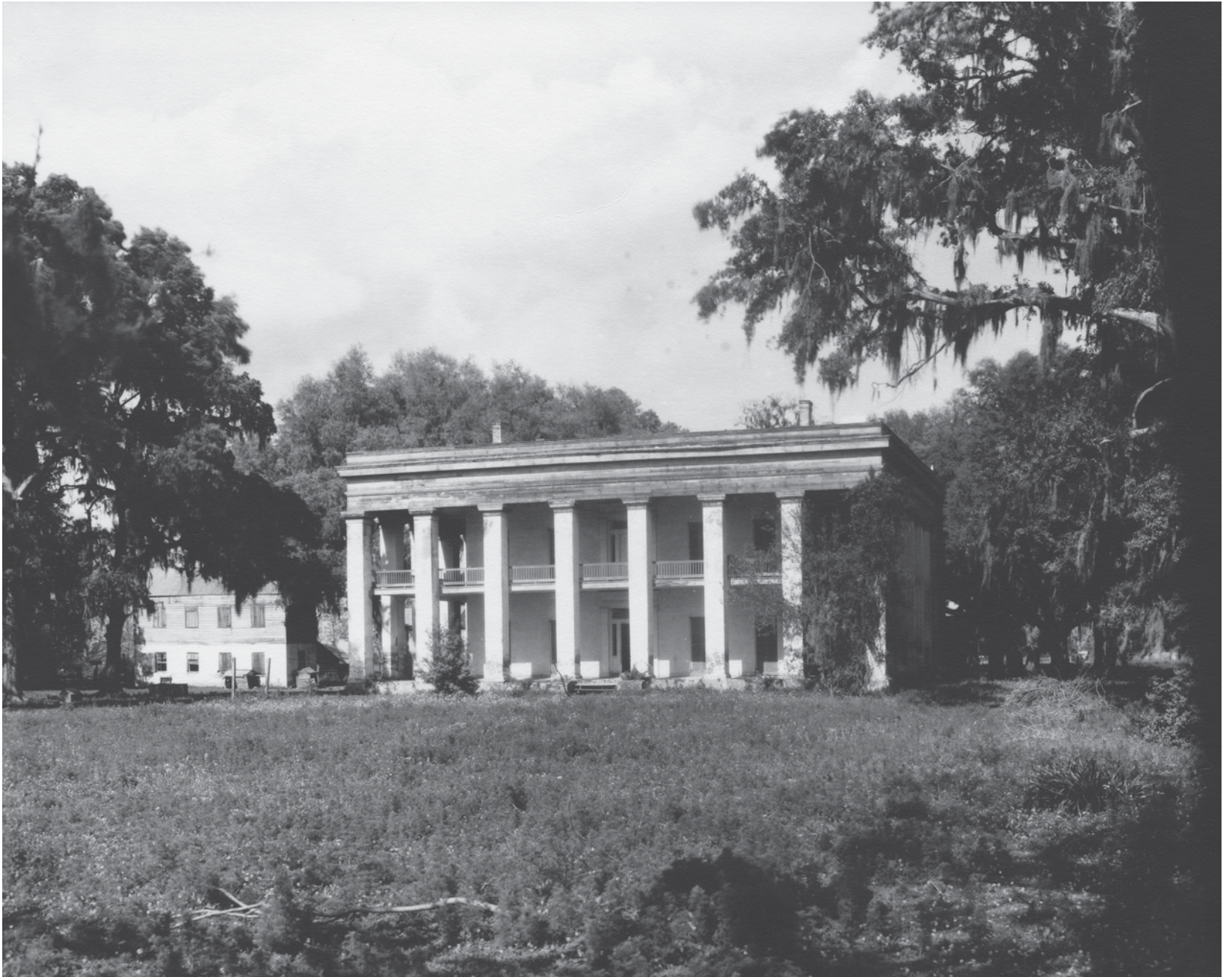
Ashland/Belle Helene Plantation (front elevation from a distance), gelatin silver print, Louisiana State Museum, 1956.087.262
