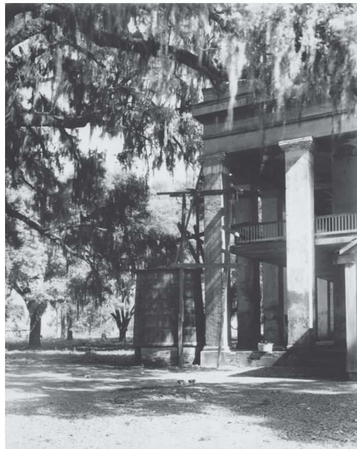
Ashland/Belle Helene Plantation (detail of side gallery, featuring Doric columns, pediment, and entablature), gelatin silver print, Louisiana State Museum, 1956.087.264
