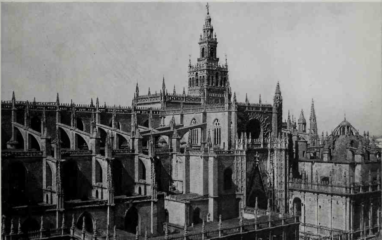
177 Seville Cathedral (c.1401-1521) is the largest church in Christendom, and unlike any other. Here, from the south, one sees the flat-roofed nave and aisles with their triple flying buttresses, and the ornate transept-front. The bell-tower beyond is an Islamic minaret, heightened in the 16th century
