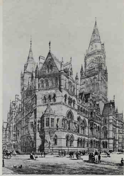
361 Town Hall, Manchester (1869): Alfred Waterhouse adapted the current Gothic style to the elaborate requirements of new commercial and civic buildings with great ingenuity. The massive Gothic skyline of the Town Hall did not prevent it being – in its own day – an extremely efficient building
