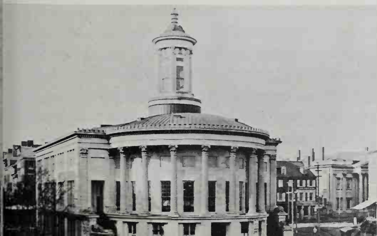
344 Merchants' Exchange, Philadelphia (1832-4), designed by the city's Greek Revival architect, William Strickland. An elegant Corinthian Order rounds the corner, below a cupola reminiscent of the Choragic Monument of Lysicrates at Athens
