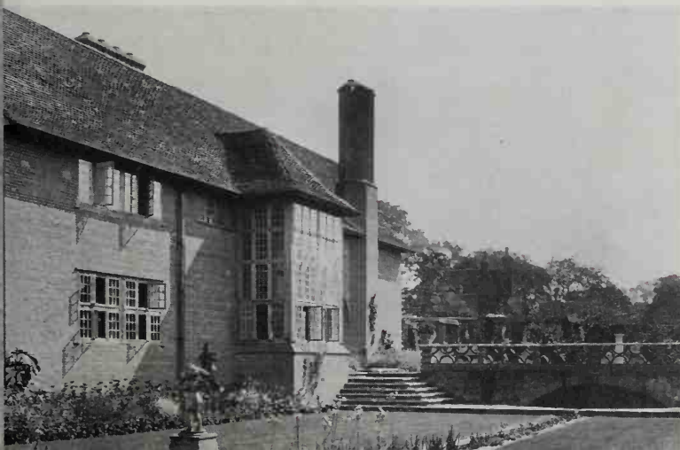
373 Deanery Garden, Sonning (1901), one of the most serene of Lutyens's earlier houses. This is the architectural fruit of Morris's revival of craftsmanship, with its impeccably handled brickwork and wooden window-mullions, and also the perfect marriage of house and garden
