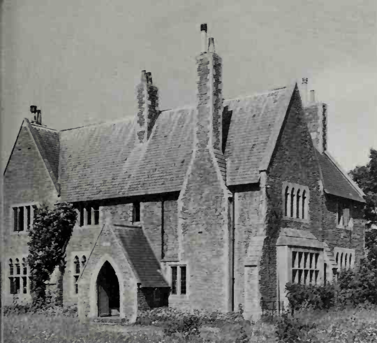
368 The Vicarage, Coalpitheath (1844-5). In spite of Butterfield's elaborate and polychromatic churches, a house such as this shows that he was far ahead of Webb in his appreciation of the traditional and craftsmanlike English house. Like medieval buildings, it is planned from the inside out: the irregular exterior expresses the plan, rather than dictating it
