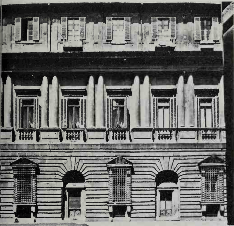
208, 209 The Palazzo Vidoni-Caffarelli in Rome (c.1515), by Raphael, shows the palace design invented by Bramante in the 'House of Raphael': a heavily rusticated ground storey, below a 'piano nobile' with windows set between paired columns. The High Renaissance achievement is clearly seen if one compares this richly sculptural façade with the first palace design to make use of the orders, Alberti's Palazzo Rucellai in Florence (below), of 1446-51
