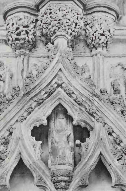
163 Detail of wall-arcading in Ely Cathedral Lady Chapel (1321-49). The ripple of oak leaves, the double ogee curves of the arches, and the way in which these 'nod' forward allowing a shaft to pass, as it were, behind them, makes this a triumph of the Decorated style
