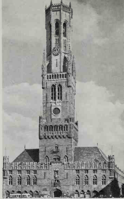
134 The Cloth Hall at Bruges, with its overwhelming tower raised in 1482, expresses the secular, mercantile wealth of one of the most prosperous towns of medieval Europe
