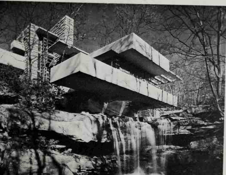
399 Kaufmann House, Bear Run (1936). This probably came nearest, of everything Wright built, to true 'organic architecture'. It makes a full use of concrete, but the broad cantilevered balconies are there also as a foil to the delicate tracery of the birch forest
