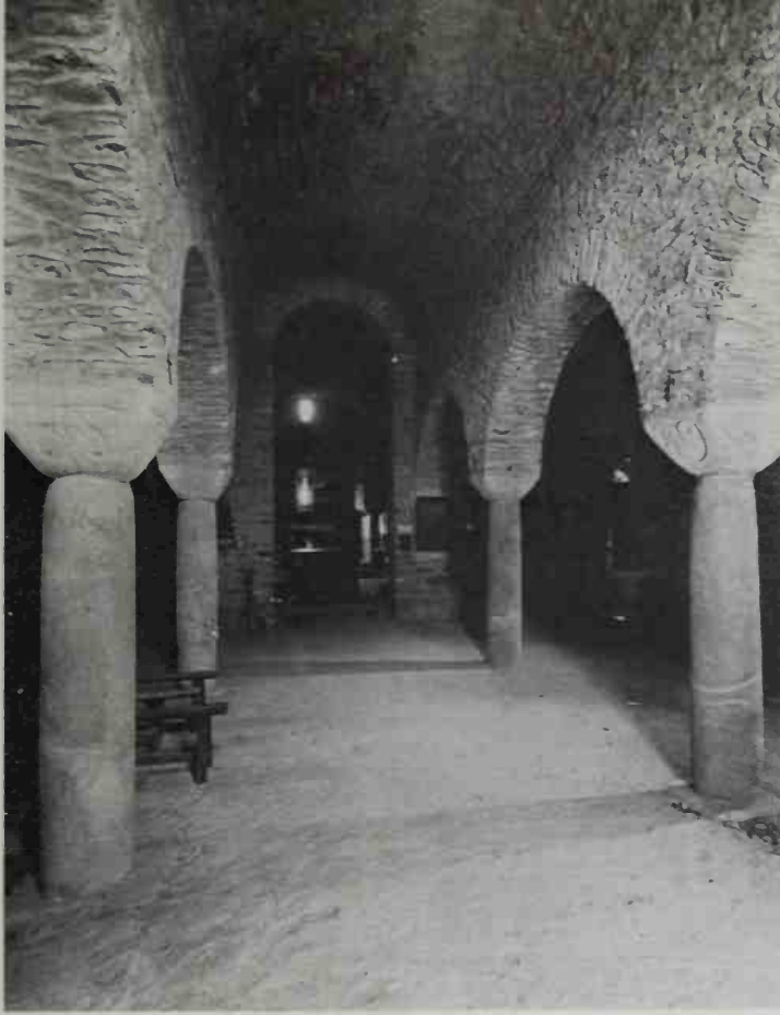
111 The interior of St-Martin-du-Canigou is remarkable for its date in having long tunnel vaults which rest only on a central arch and on eight columns with rough capitals. There is neither gallery nor clerestory
