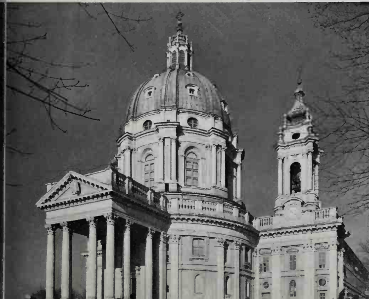
311 Superga, Turin (1717–31). Juvarra takes an eclectic collection of elements and makes them into a completely original composition. A central-space church is set into one end of a convent quadrangle, and rises in a dome almost as big as itself (compare the design of walls and dome with St Peter's, Ill. 206). The wilfully large – almost independent – portico is balanced by the convent wings, crowned with towers (cp. Ill. 245)
