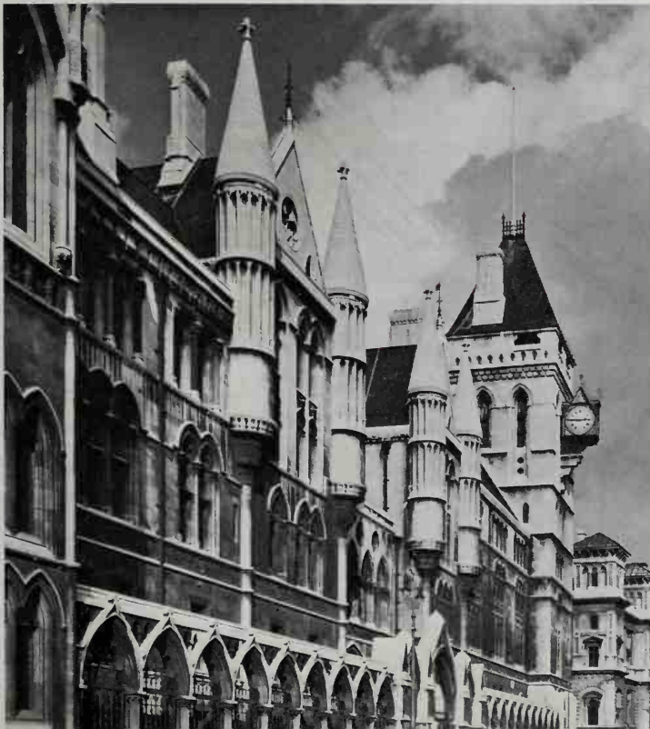
362 In the Royal Courts of Justice, London (designed 1866), G.E. Street showed his genius for grouping and for breaking up a long façade without loss of unity. The street-level arcade ties the composition together
