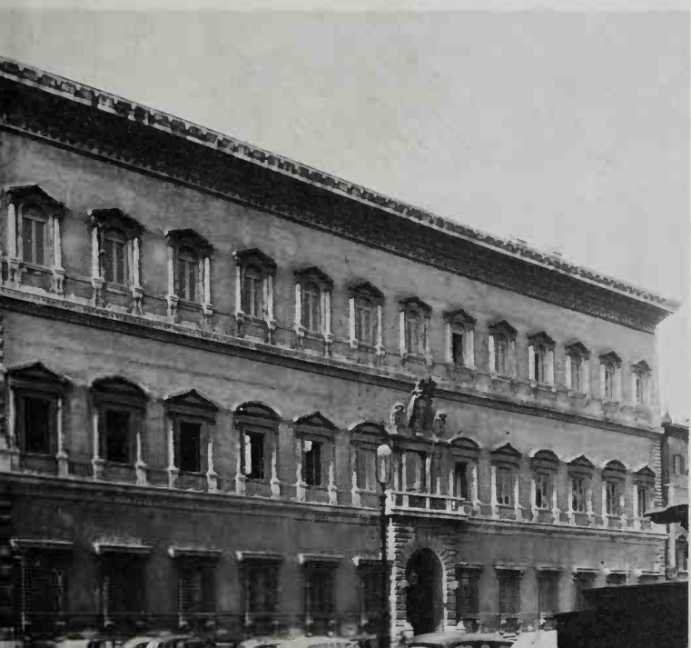
212, 214 Palazzo Farnese, Rome (1534–40), designed by Antonio da Sangallo and completed – with the window over the doorway (opposite, below), and the upper storey where window-frames rest on twin consoles – by Michelangelo. Smaller parts, such as the balcony and cartouches, build up to tell the eye how large the building really is
