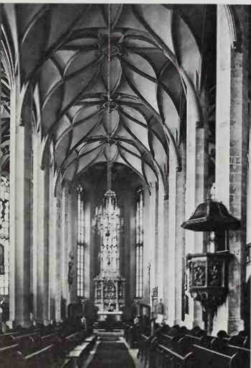
95, 96 Romanesque achievement and Gothic virtuosity: above, Ste-Foy at Conques (begun c.1050; see also p. 113) with high tunnel-vaulted nave, and crossing covered by a lantern on squinches; below, St Anne, Annaberg (begun 1499; see also p. 154) – the functional stone vault transformed into a fantastic pattern of ribs
