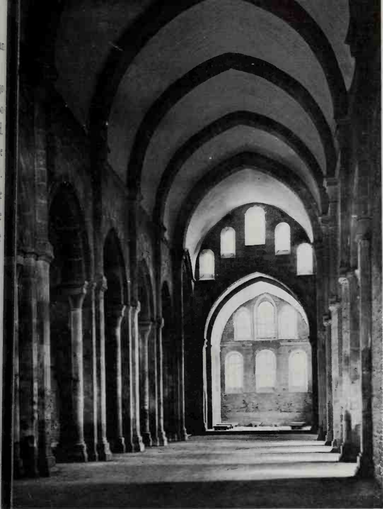
122 Fontenay (1139-47), the Cistercian ideal. The piers are articulated, but there is no sculpture and the east end is austerely square. The arcade is slightly pointed, and wall-shafts carry the transverse arches of a pointed tunnel vault
