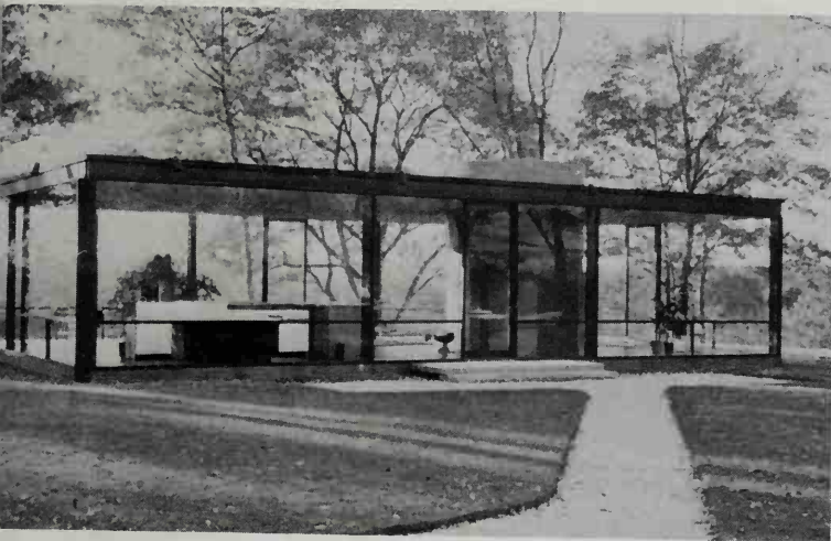
426 Philip Johnson House, New Canaan (1949). This is the Miesian approach to the purest use of glass and steel: a glass box for living in, justified by its setting in lake and woodland
