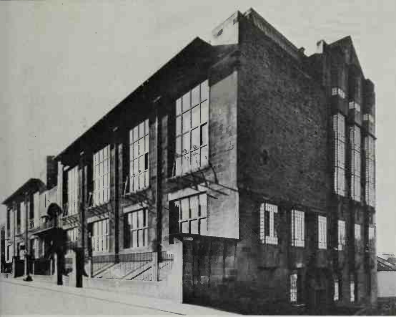
390 Glasgow School of Art. Mackintosh built the first section, on the left, in 1897-9. It has minor touches of Art Nouveau decoration, but its big studio windows are frankly functional. The later section of 1907-9, on the right, makes a more dramatic use of form: the library's long iron-framed windows set in plain stone tower up from the steep street
