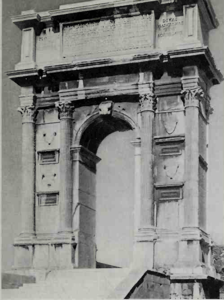
50 The Arch of Trajan at Ancona (AD 113) was purely decorative and ceremonial, standing in isolation on the end of the quay. While simpler than the arches in Rome, it has the same features: a central opening with flanking features framed by columns, and an 'attic' stage above the cornice. The tripartite division of the triumphal arch gave architecture a new motif (see, e.g. Ills. 199, 201, 204)
