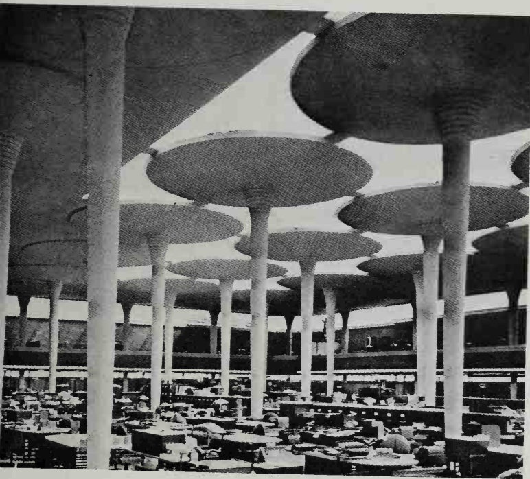
398 This large open office for S.C. Johnson and Son (Racine, 1936-9) was one of Wright's early masterpieces. The beautifully slender mushroom columns – built in defiance of the general opinion that they would never stand – support a most curiously contrived ceiling of glass tubes
