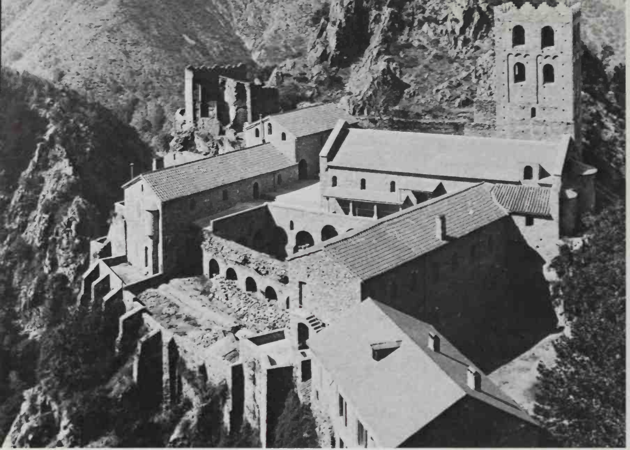
110 St-Martin-du-Canigou (1001–26), from the south: a noble piece of siting. The monastic buildings are compressed on a rocky spur around the low cloister; to the left is the refectory and to the right the dormitory, joined to the church, which stands between the cloister and the bell tower
