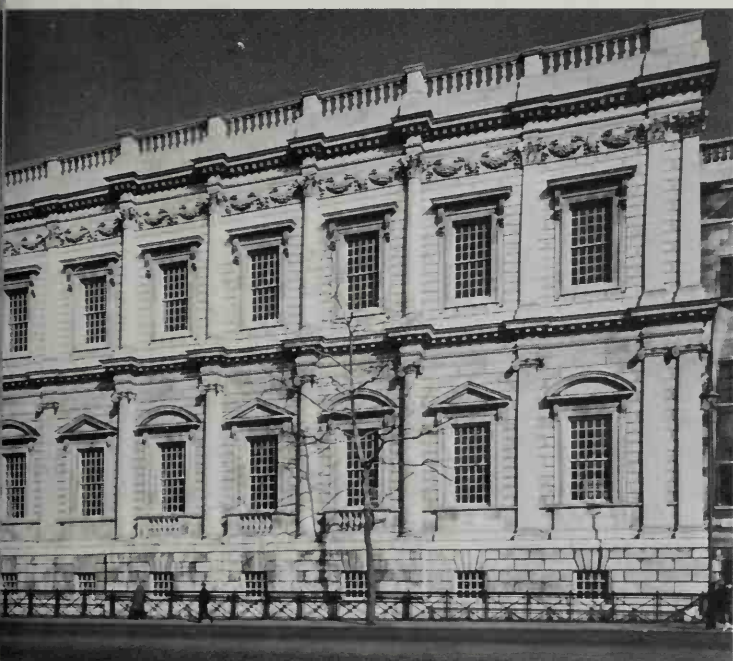
285 Banqueting House, Whitehall, London (1619–22), by Inigo Jones. The façade is articulated by columns in the centre and pilasters at the side, though the division into two tiers hardly reflects the single large room inside. It is a more elaborate and ornate composition than the Queen's House, but beautifully – and extremely carefully – proportioned
