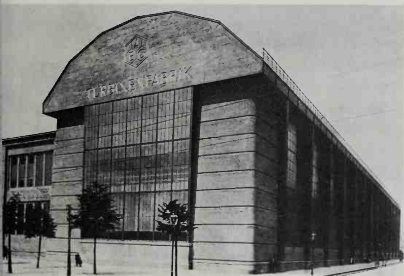
391 For his purely utilitarian Turbine Factory in Berlin (1908-9) Peter Behrens created a great expression of power. The sides consist only of iron and glass, while the corners are formed by massive pylons of poured concrete below a concrete 'pediment'
