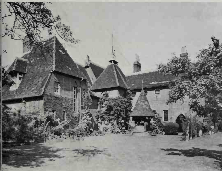
369 Philip Webb's Red House at Bexley Heath (1859-61), built for William Morris, shows a picturesque and romantic grouping of roof and chimneys around the focal point of a well-head. There is practically no ornament or stylistic detail; what there is comes equally from Gothic and from the 17th century
