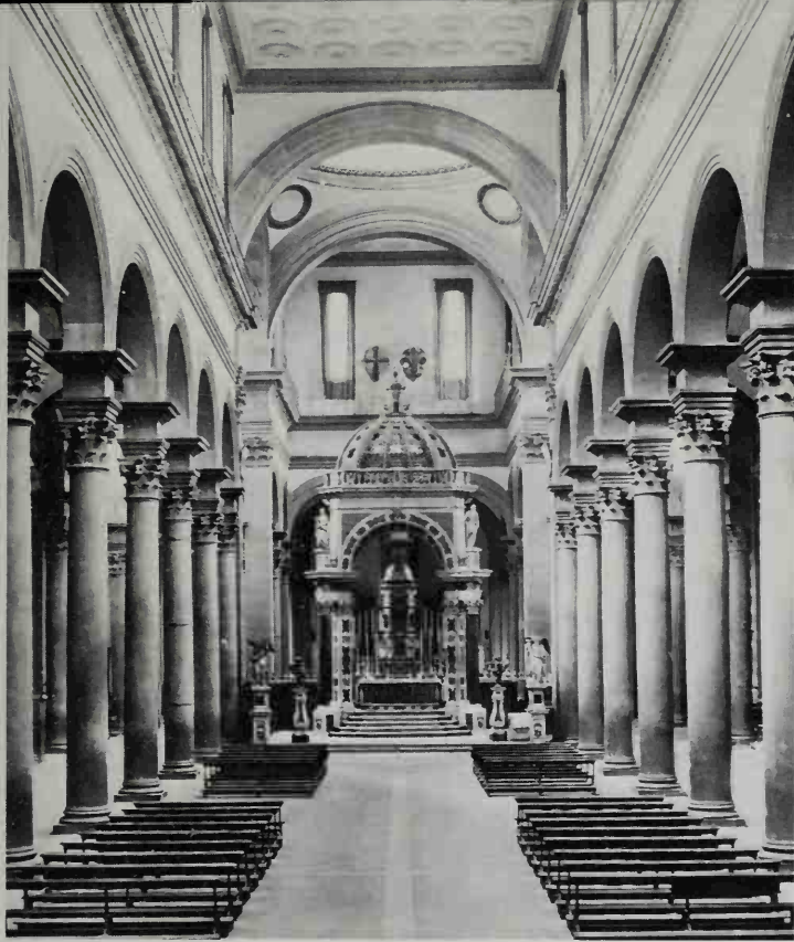
193 Sto Spirito, Florence (1436–82), by Brunelleschi. Nave and choir are covered by flat coffered ceilings, the crossing by a dome. The purist treatment of the arcade – with chunks of entablature above each capital – was scarcely seen again until the 18th century (Ill. 332)
