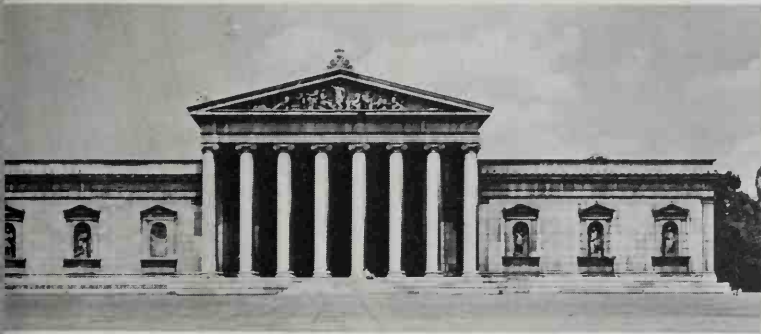
342 Glyptothek, Munich (1815-34). Leo von Klenze was, like Schinkel, an exponent of Romantic Classicism. This building, with central Grecian portico and side walls relieved by Renaissance aedicules – the three parts perhaps too nearly equal in width – was built to house the Duke of Bavaria's magnificent collection of antique sculpture
