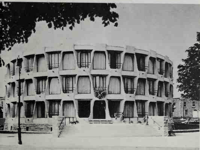
418 United States Embassy, Dublin (1963), by John M. Johansen. Another approach to building in concrete: the wall is built up of regular pre-cast sections. It rests, however, on a fortress-like, rusticated basement. The circular plan resolved the problem of an awkward site
