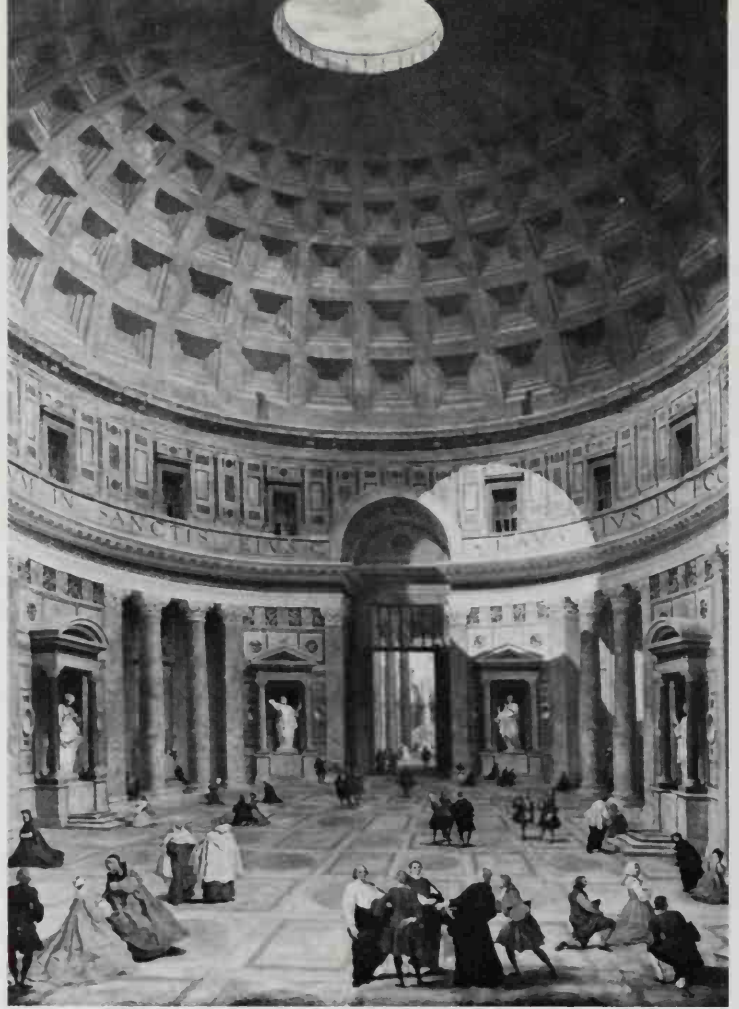
47 An 18th-century view of the Pantheon, showing its original marble panelling. Note the alternation of columned recesses and niches flanked by colonnettes. The interior is dramatically lit through the 'eye', giving a spotlight effect; surrounded by bronze stars in the coffers of the dome, this opening symbolized the sun at the centre of the universe
