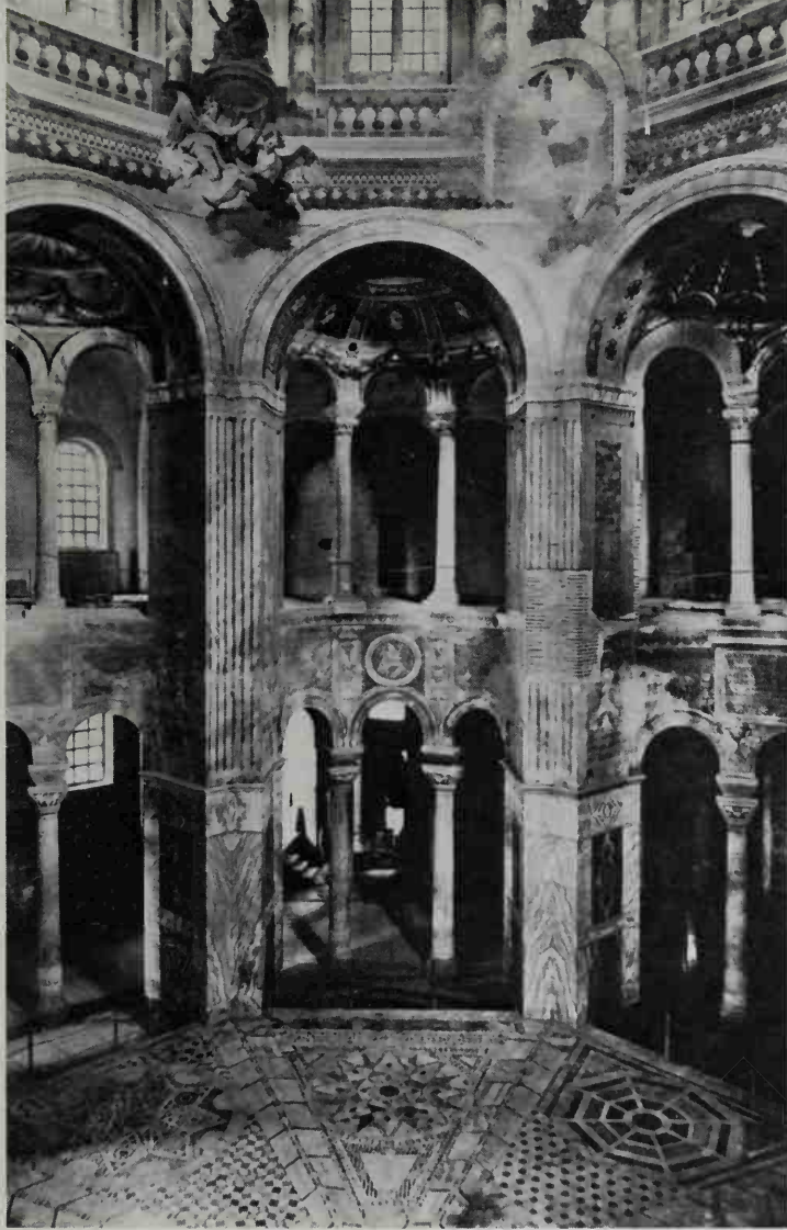
74, 75 Interior and plan of S. Vitale, Ravenna (547). Like SS. Sergius and Bacchus, the central domed area is octagonal. Here, however, the surrounding aisle is also octagonal, and the openings between it and the central area are all curved in plan. This produces a still subtler interpenetration of spaces
