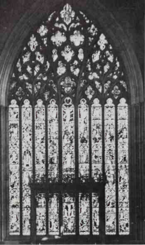
159 East window, Carlisle Cathedral (c.1290): the beginnings of Decorated
