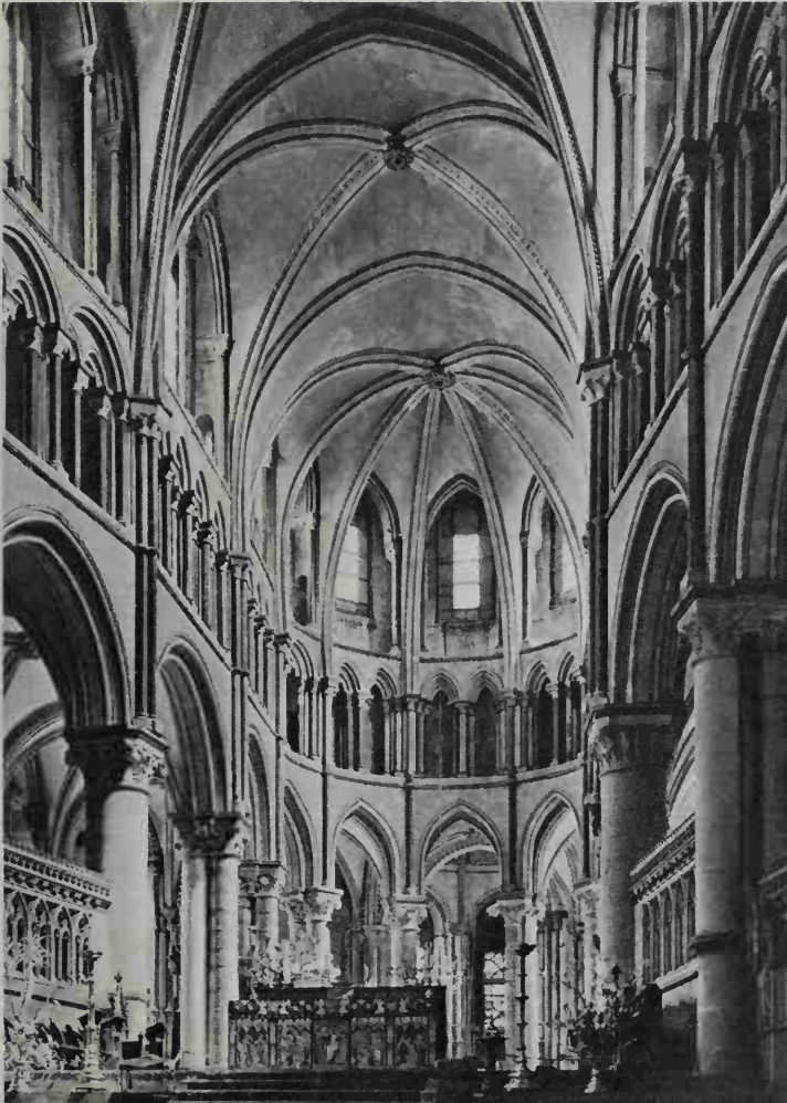
152 Canterbury Cathedral choir (begun 1175), by William of Sens and William the Englishman. The design retains some features of English Romanesque (low proportions, some round arches, zigzag ornament) combined with others from early French Gothic (crocket capitals, sexpartite vaults in the western bays, and coupled columns – a speciality of Sens). It was such combinations which, together with the use of Purbeck marble, were to characterize the development of English Gothic
