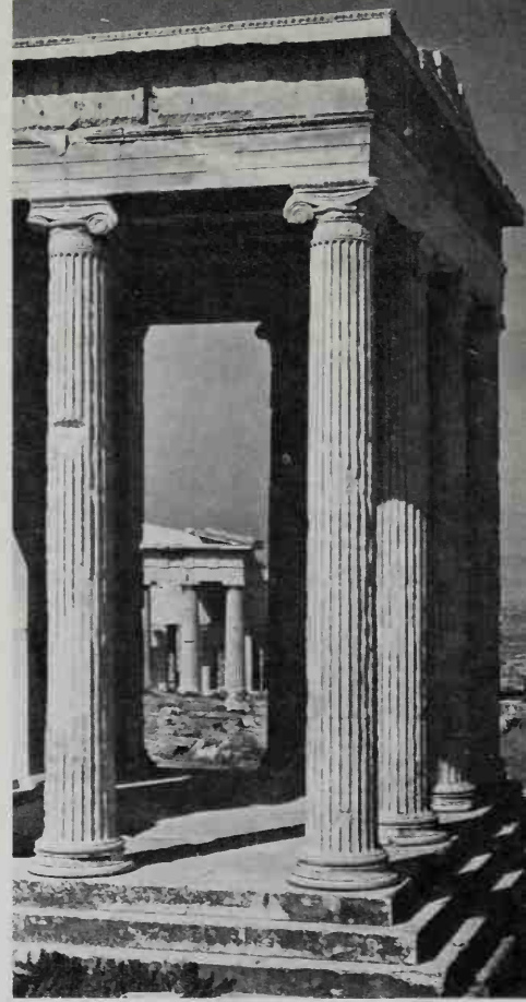
30 North porch of the Erechtheum (at the top in Ill. 28). Slender Ionic columns, 25 feet high, are unusually widely spaced, giving an airy effect. Above them in the frieze white marble figures were attached to a grey stone background
