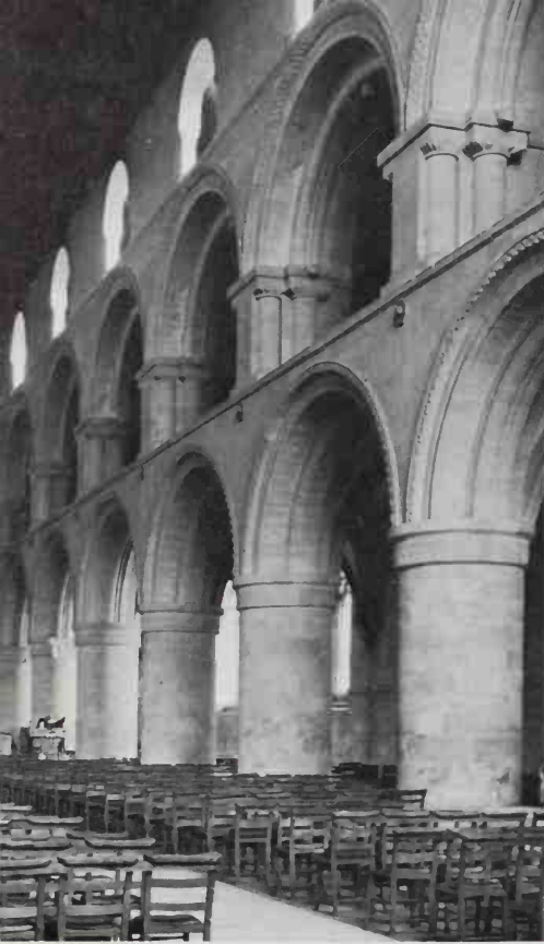
107 Southwell Minster nave (c.1130), a variation within the three-tier elevation. The triforium has arches as wide as those of the arcade below; it also has articulated piers, whereas those of the arcade are cylindrical
