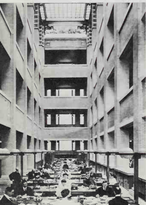
389 Frank Lloyd Wright built the open-plan Larkin Building at Buffalo, N.Y., early in his career (1904). The strong horizontal lines and plain brickwork, so superbly used in his later work, are already there
