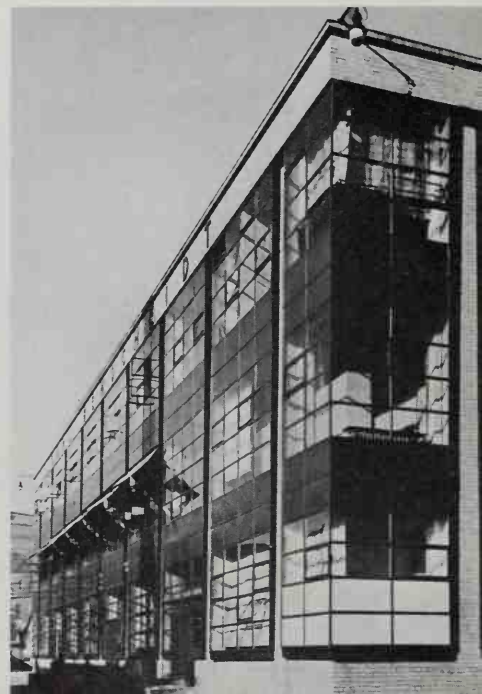
392 Fagus Factory, Alfeld (1911). Where Behrens had emphasized the corner, Gropius and Meyer abolished it, showing that steel and glass could achieve delicacy as well as strength
