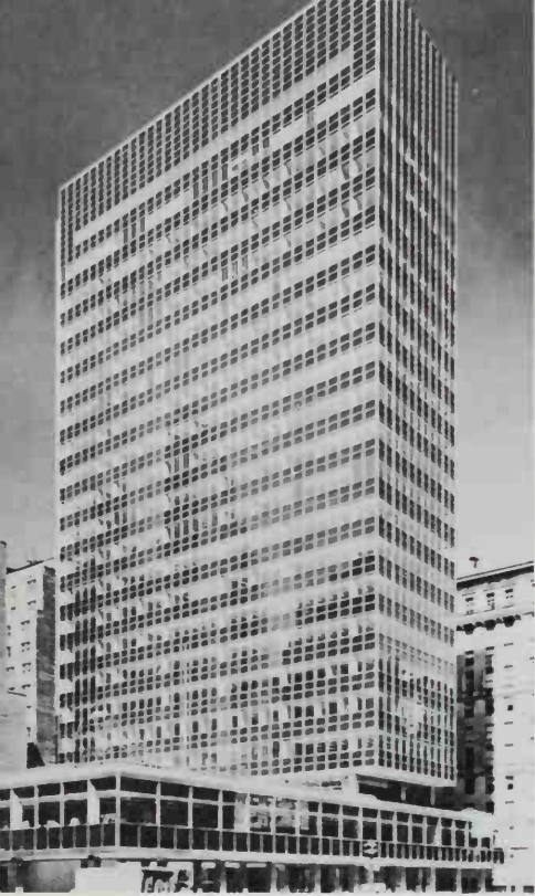
423 Lever Building, New York (1952), by Gordon Bunshaft of Skidmore, Owings and Merrill. A Mies-inspired and much-imitated combination of a curtain-walled office tower with a low podium (containing forecourt, restaurant and shops)
