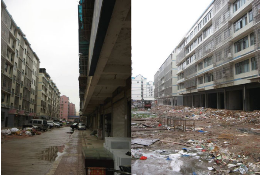
Fig. 3.4 Built environment of Sifangping community, March of 2010
