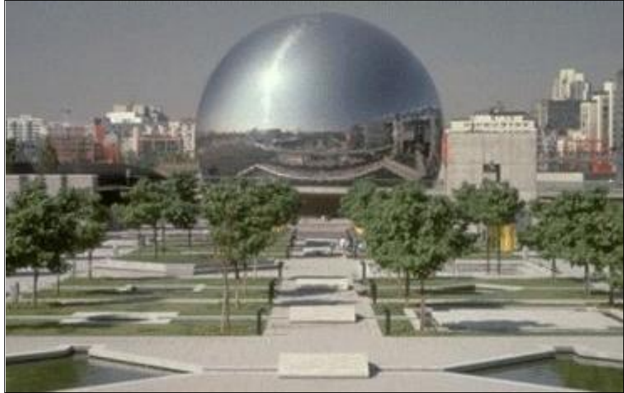
Figure 1 General view of La Geode
