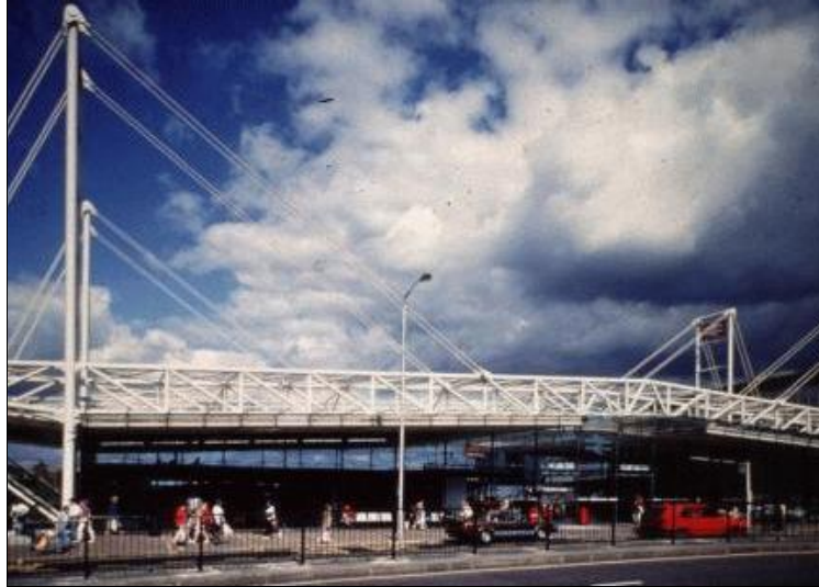
Figure 1 General view of the station
