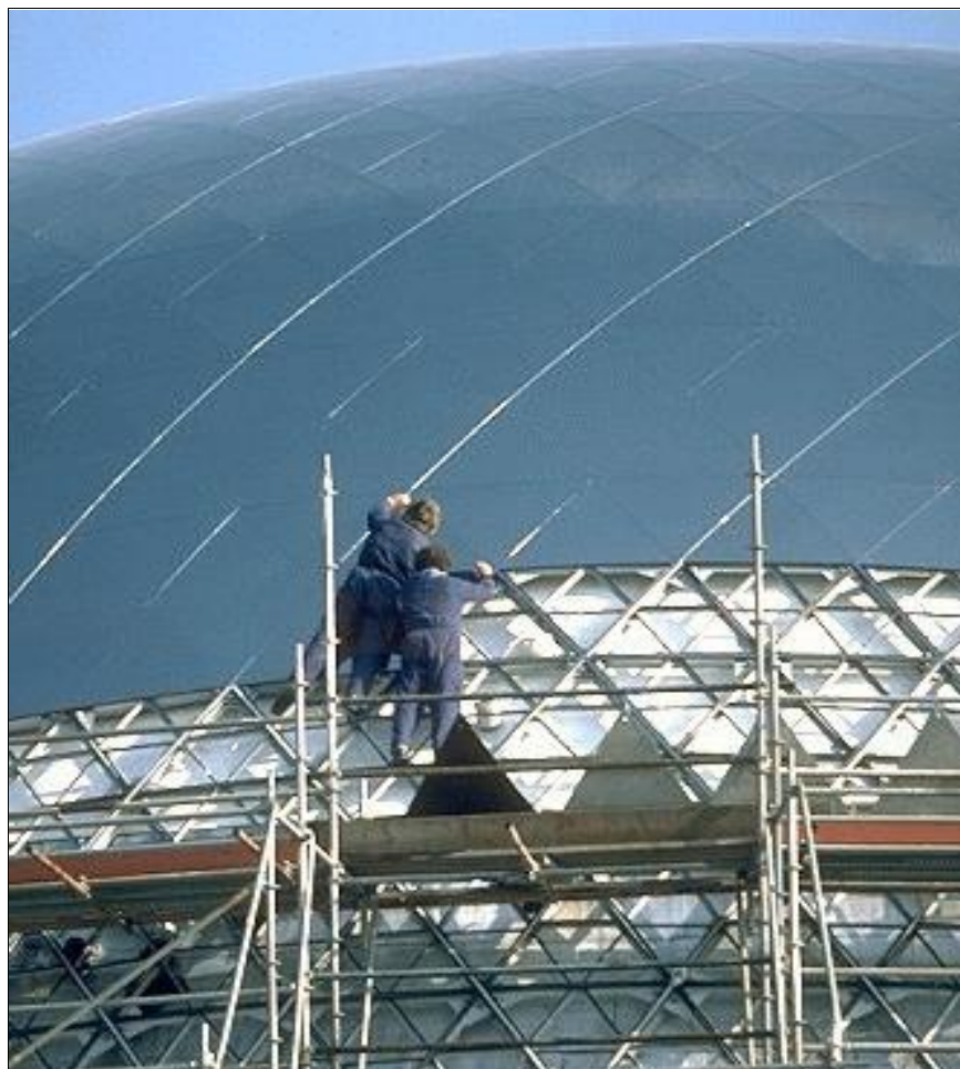
Figure 6 Erection of stainless steel skin
