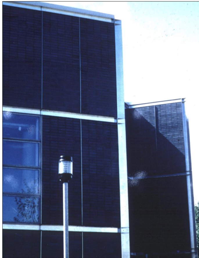
Figure 2 Exposed stainless steel channels support brick panels
