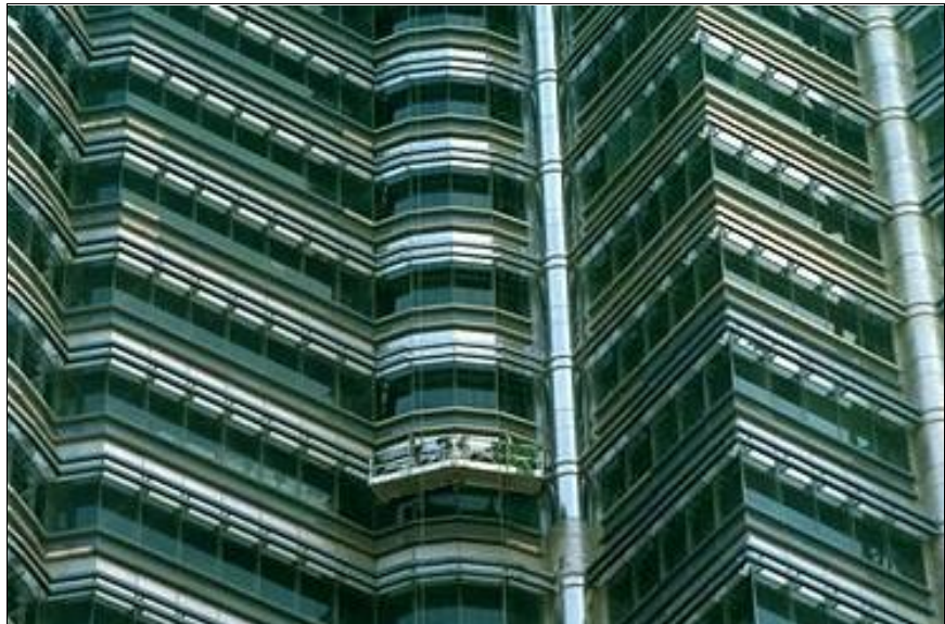
Figure 2 Cladding consists of ribbons of stainless steel and glass
