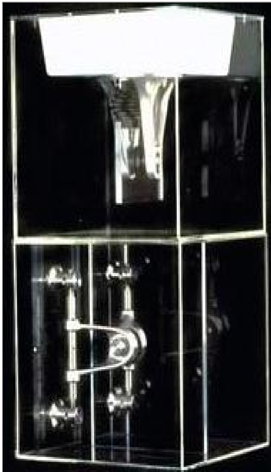
Figure 9 Glazing connection using stainless steel cast components
