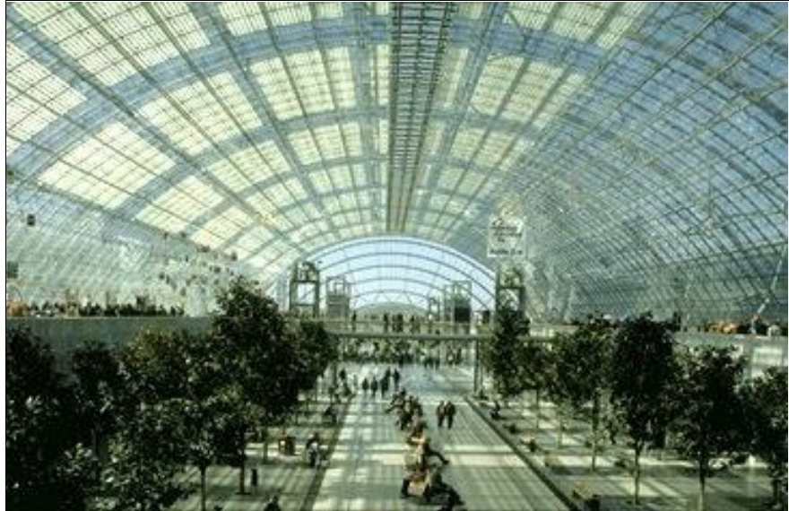
Figure 1 Internal view of the glass hall
