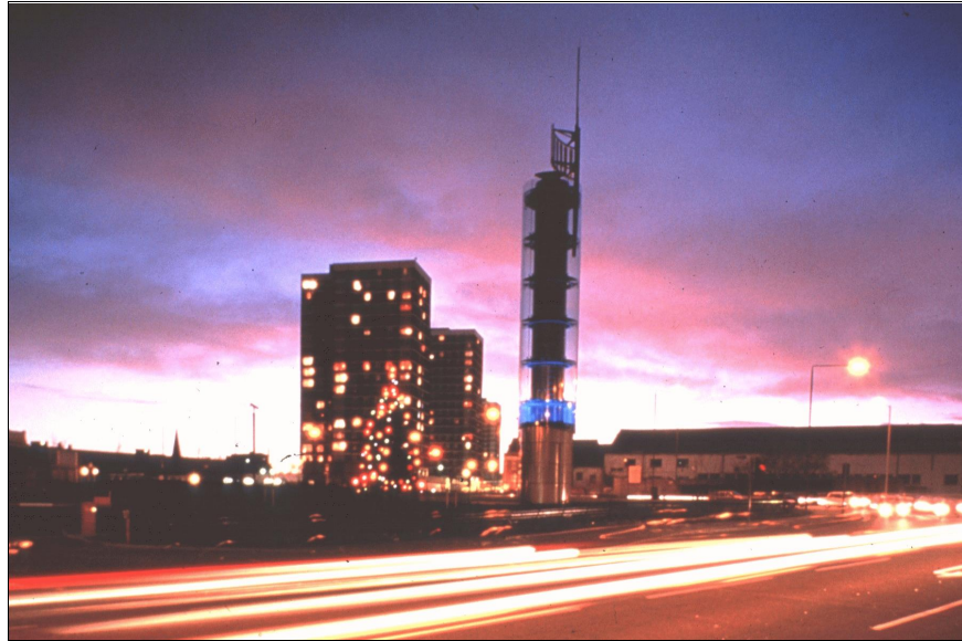
Figure 1 General view of the tower
