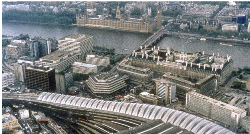
Figure 1 Waterloo International Terminal - aerial view
