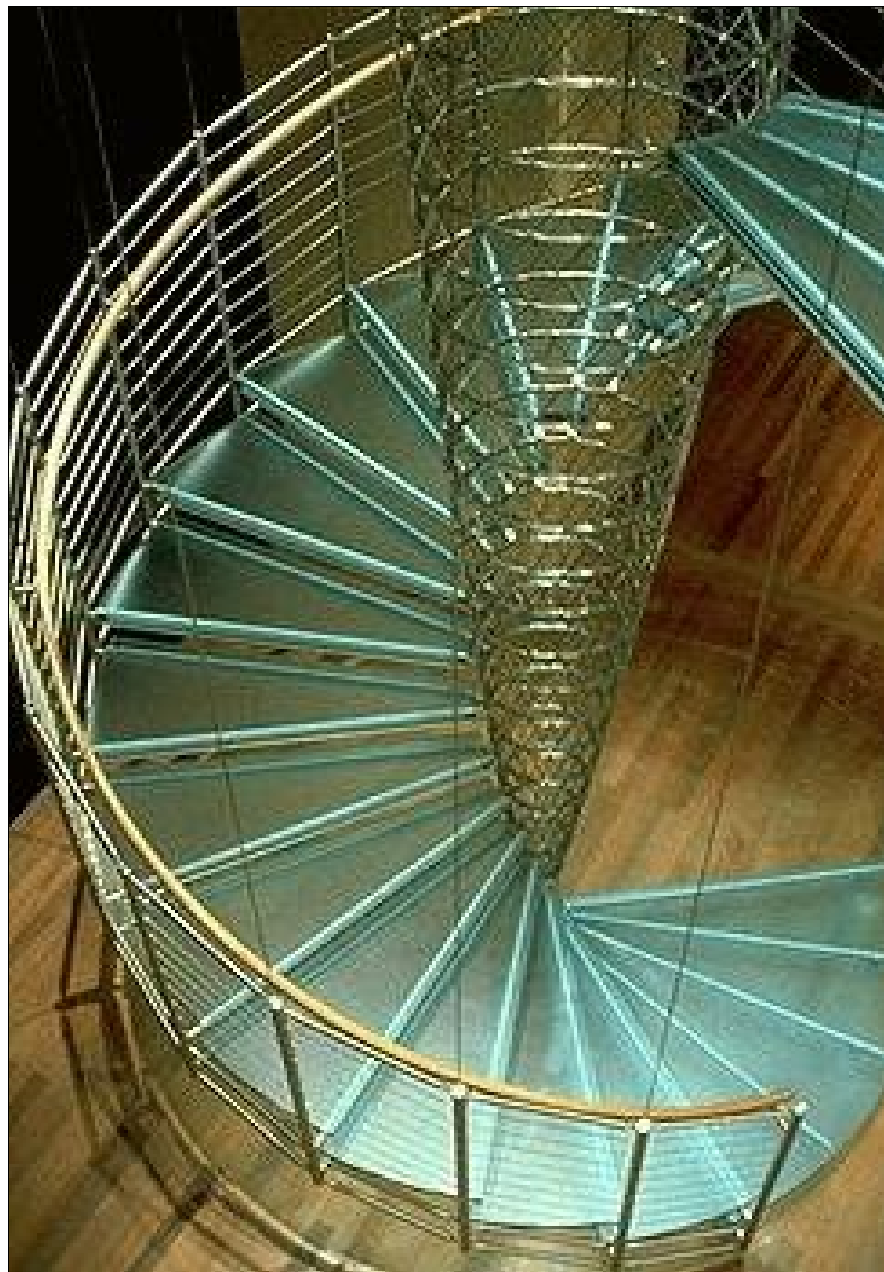
Figure 1 Translucent glass treads spiral round the slender cone of stainless steel mesh
