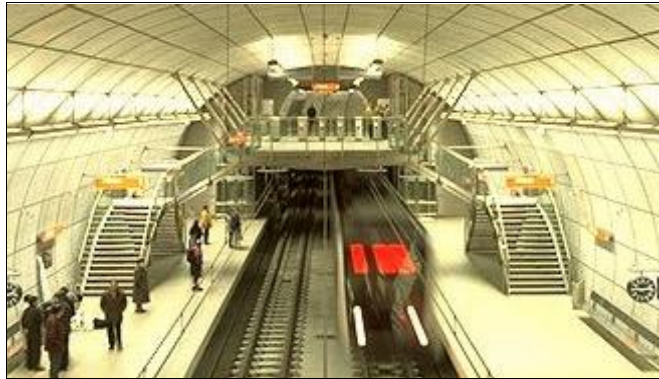
Figure 2 The mezzanine provides the link between the platform and the access tunnels
