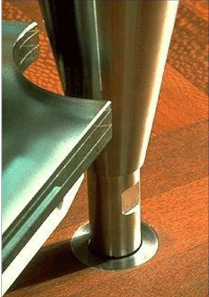
Figure 3 Stairs are aligned and tensioned with a single turnbuckle at the cone base
