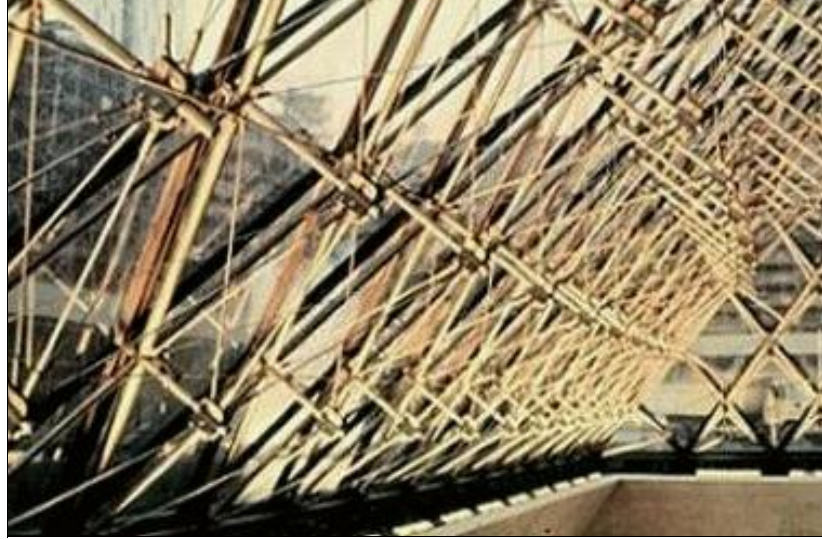
Courtesy of TriPyramid Structures Inc.
