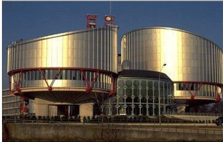
Figure 2 The 'head' comprises a pair of large stainless steel drums joined by a glass cylinder
