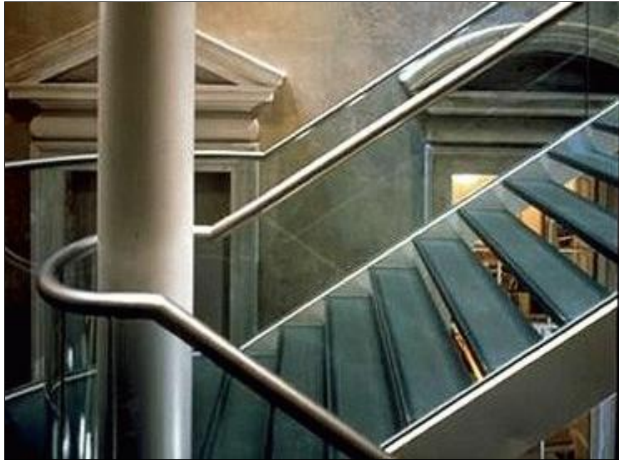
Figure 5 Bead blasted stainless steel handrail
