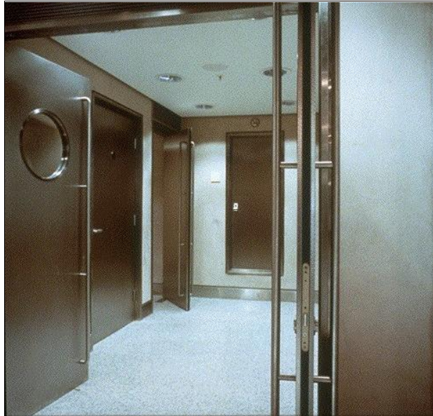
Figure 14 Stainless steel lined doors and door furniture
