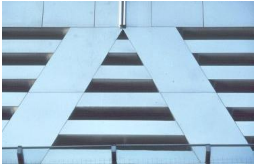
Figure 2 Single-sided textured stainless steel cladding is used for the external envelope
