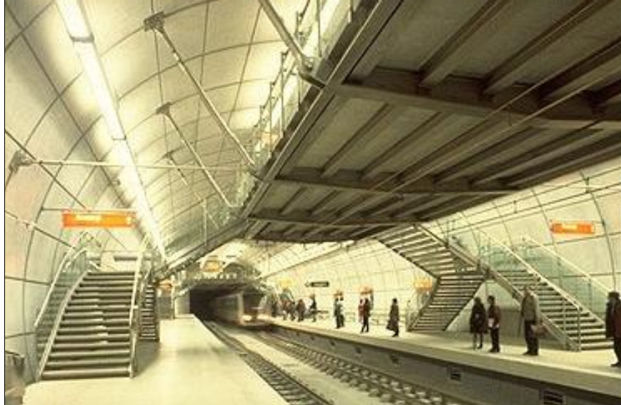
Figure 6 Stainless steel hangers and struts support the mezzanine
