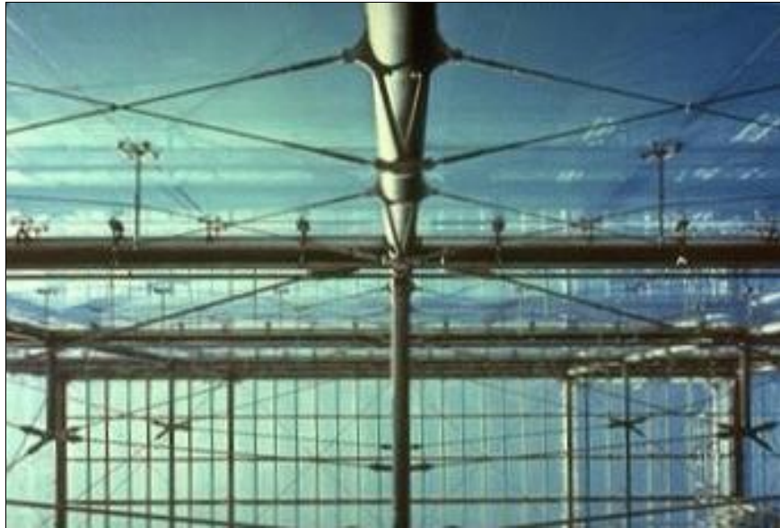
Figure 2 The support structure to the Serres
