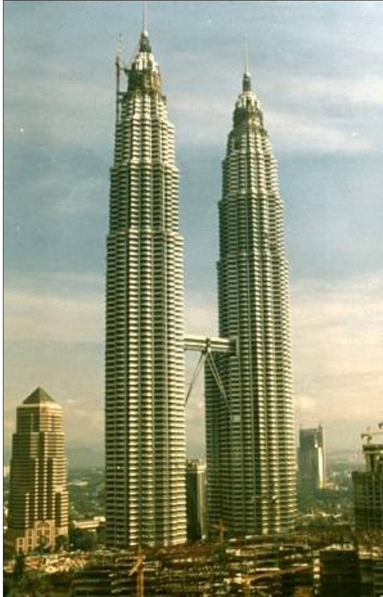
Figure 1 Twin towers under construction
