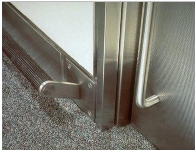
Figure 15 Stainless steel wall trims and skirting
