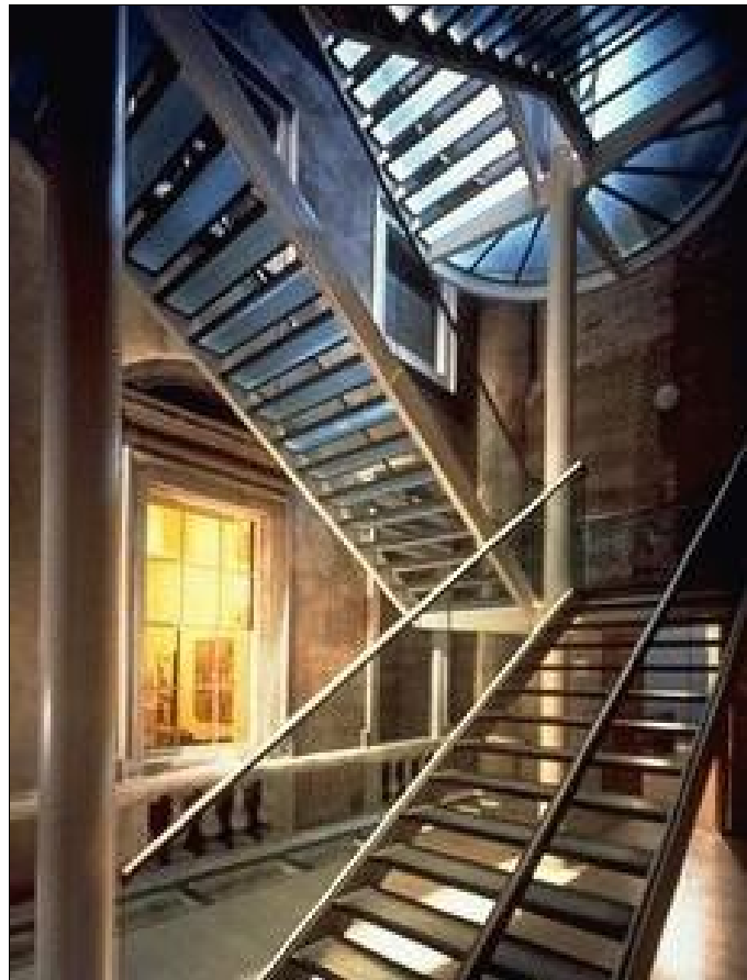
Figure 3 Glass treads and balustrades create a high degree of transparency
