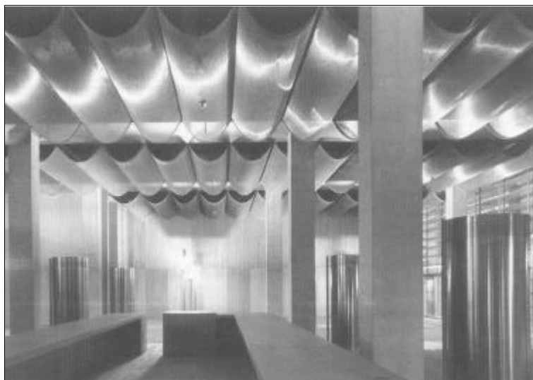
Figure D.2 Wire mesh suspended in the form of arches at the Bibliothèque Nationale de France in Paris
