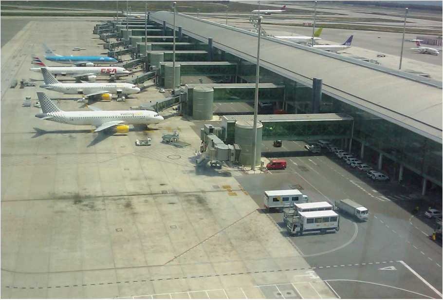
Fig. 2. Air side of terminal area.
