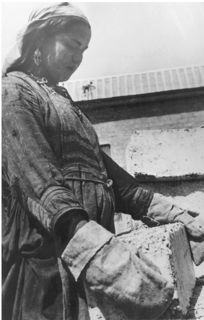
A woman worker hauls stones at Ural'mashstroï, a construction site for the Urals machine-building factory in Sverdlovsk. This work was typical of the unskilled labor performed by women on construction sites. 1931.
