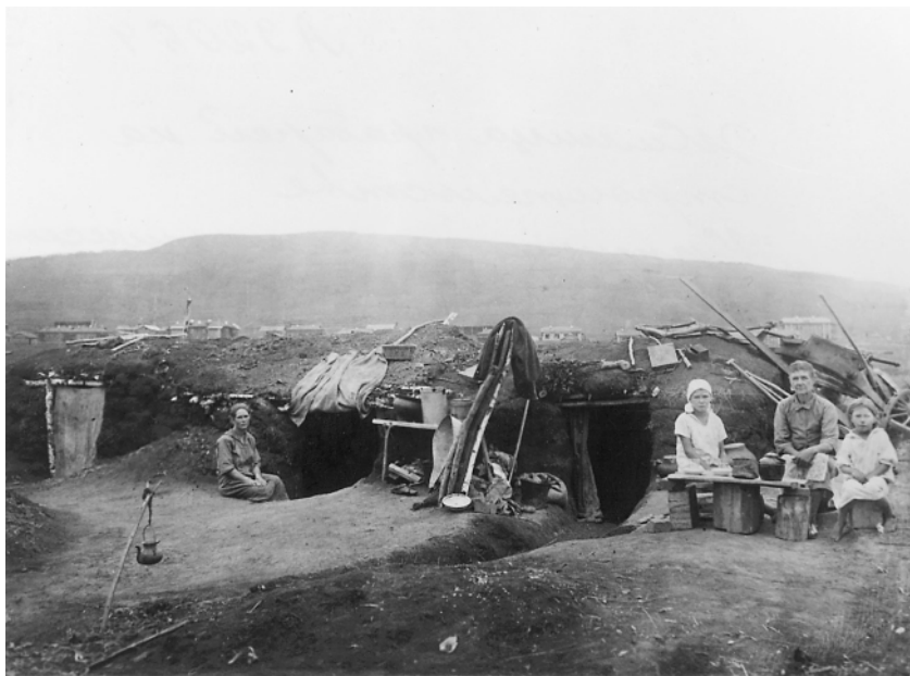
Temporary housing for workers on the construction site of the Kuznets metallurgical complex in Novokuznetsk. New workers on construction sites and in towns often lacked even the most rudimentary housing, furniture, and domestic comforts. 1930.
