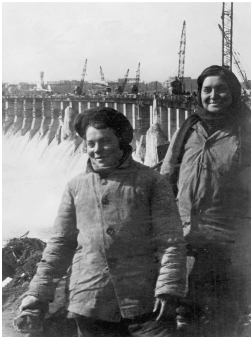
Dasiuk and Ianovskaia, two record-setting concrete workers on the construction site of the Dnieper River dam, in the Ukraine. 1932.
