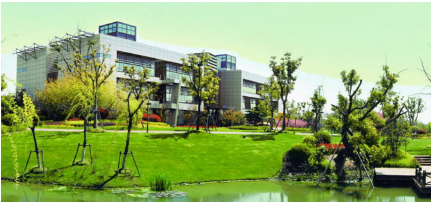
The ecological office building of Chenjiazhen company on Chongming Island in Shanghai
