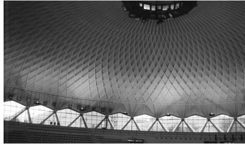
Figure 4-23 Palazetto dello Sport, internal view.
