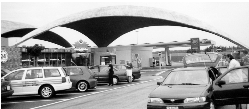
Figure 6-21 Concrete shell structure at service area on A12 motorway in Switzerland designed by Heinz Isler.
