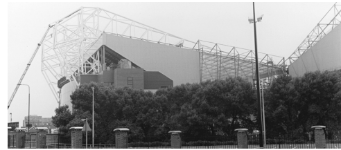
Figure 5-14 Manchester United Football Stadium.
