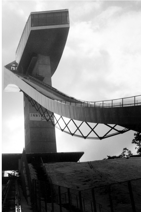
Figure 5-25 The Bergisel hill ski-jump tower and ramp, by architect Zaha Hadid and engineers Aste Konstruktion. Notice the large steel truss supporting the ramp.
