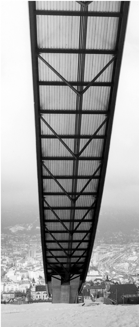
Figure 5-26 The Bergisel hill ski-jump ramp, viewed from underneath.
