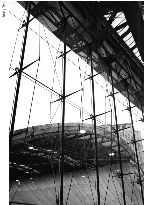
Figure 2-18 Glass mullions at Waterloo Eurostar terminal designed by Nicholas Grimshaw Architects and Anthony Hunt Associates.
