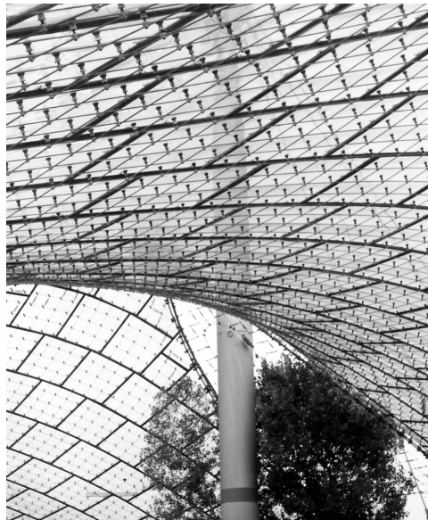
Figure 6-19 The Munich Olympic Stadium, detail of the membrane.
