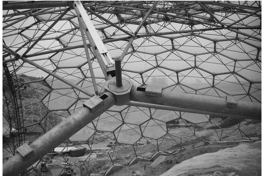
Case 4-12 Construction of the biomes, the Mero system.
