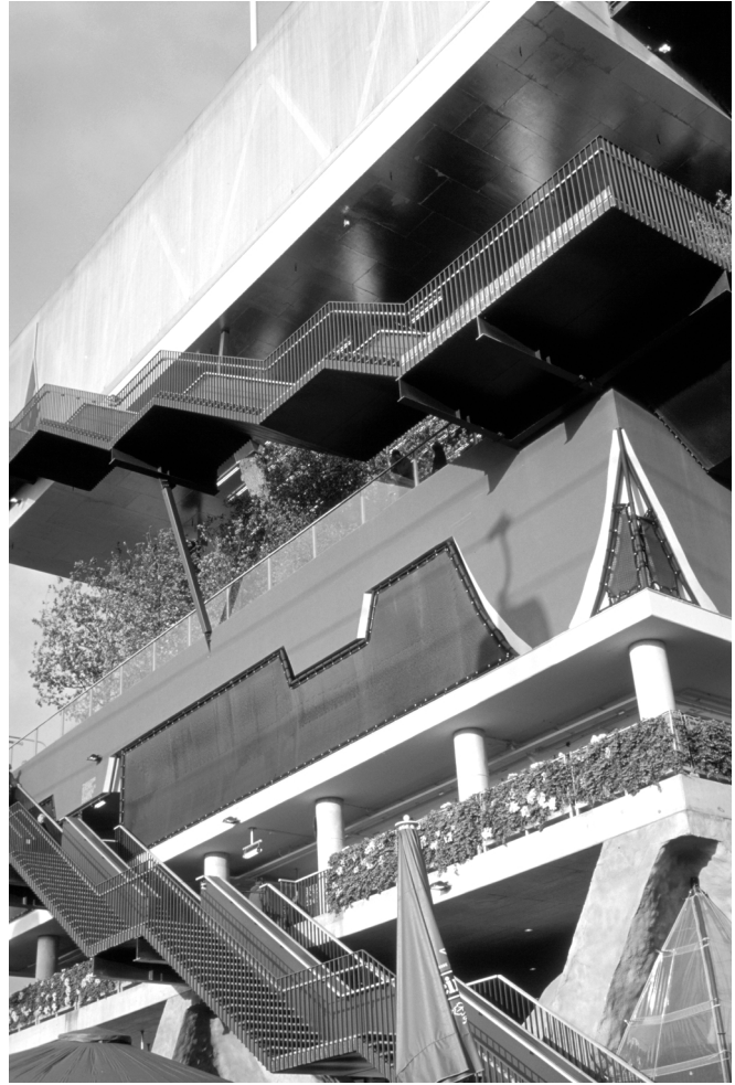
Case 3-18 Elevation, showing a glimpse of the concrete shell-like structure – bottom right corner.
