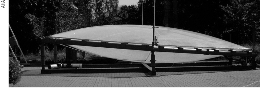
Case 4-16 ETFE cushion, trial construction and inflation.
