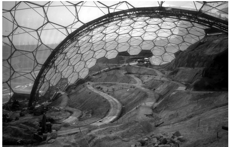
Case 4-15 Humid/tropics biome nearing completion. Note the unresolved geometry where the geodesic panels meet the stiffening arch.
