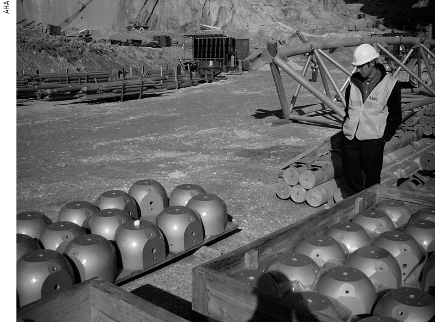
Case 4-13 Mero system connectors. Note the section of a stiffening arch in the background.
