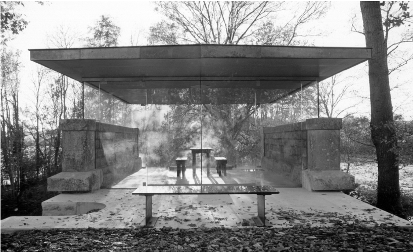
Case 2-14 The roof appears to be floating magically above the forest floor.
