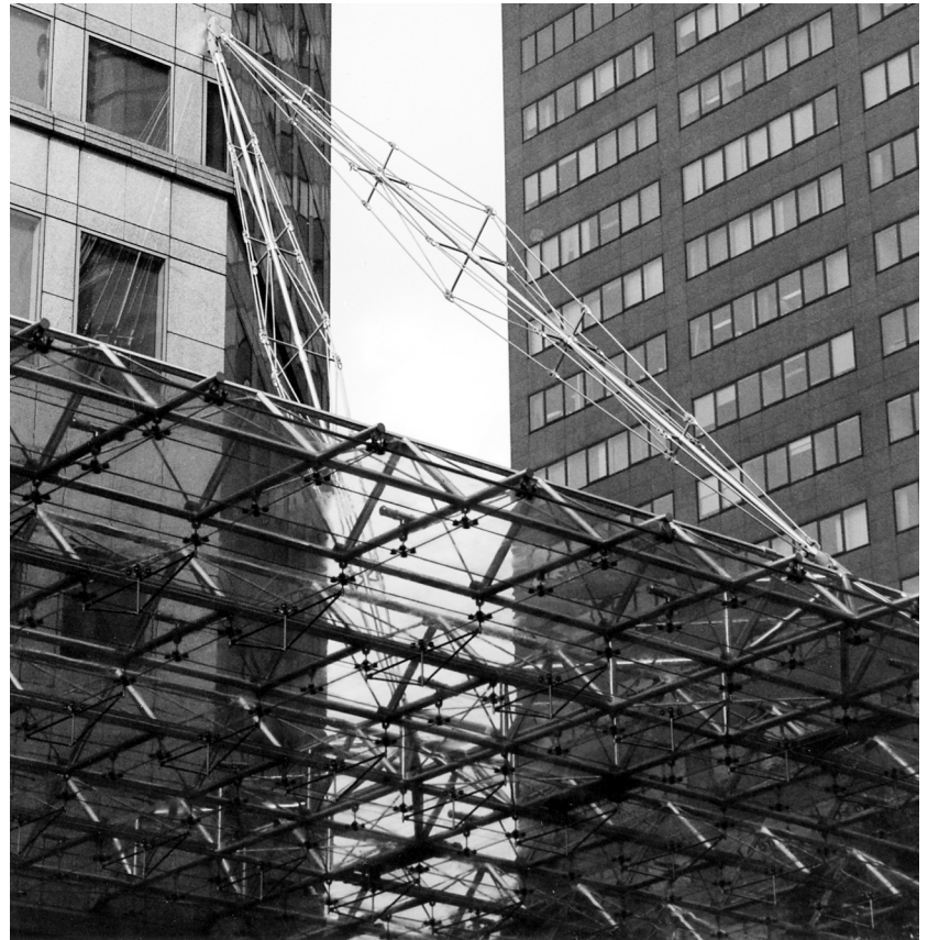
Figure 3-23 A self-stabilized support to an entrance canopy – Singapore, detail.
