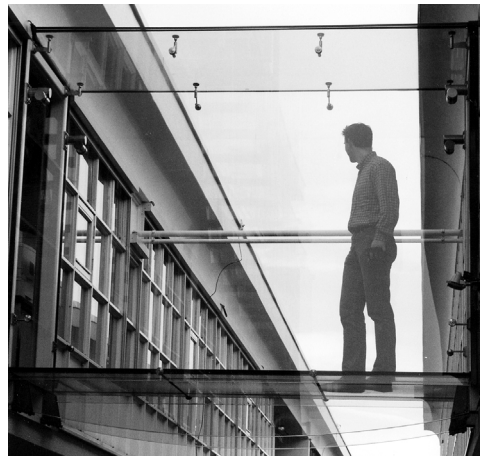
Case 2-4 Glass bridge connecting two buildings of the architectural practice Kraaijvanger Urbis Architectural Practice based in Rotterdam.
