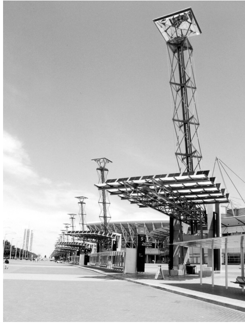
Figure 3-24 Self-stabilizing structures used for the photovoltaic lighting columns at the Sydney Olympic site.
