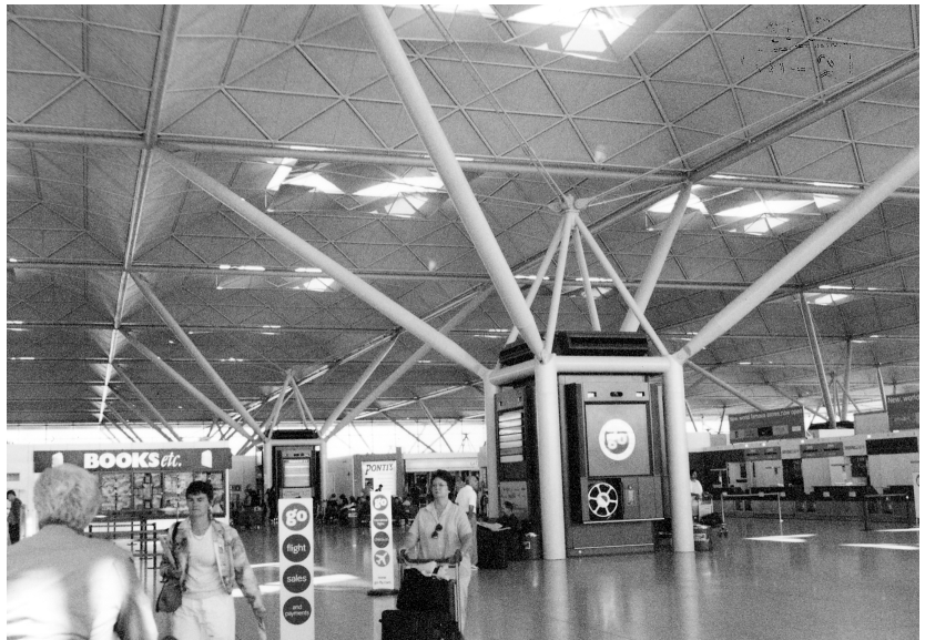
Figure 2-20 The tree structure at Stansted Airport.
