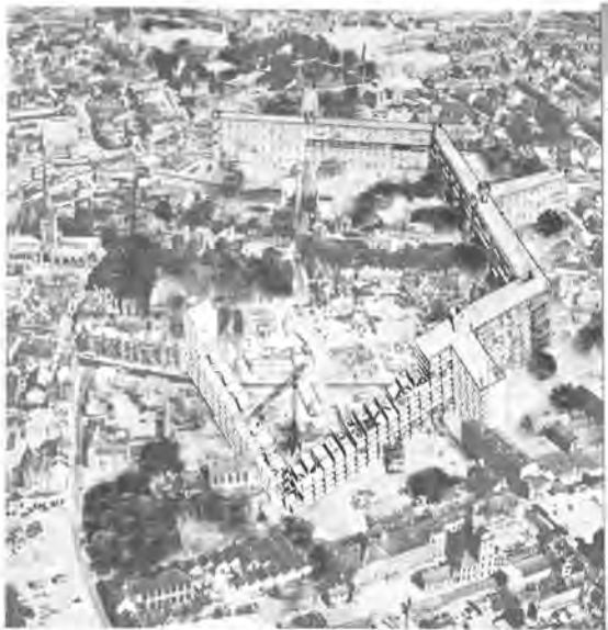
270 Alison and Peter Smithson, Golden Lane Housing system applied to central Coventry. (The parish church and ruined cathedral are on the left.)
