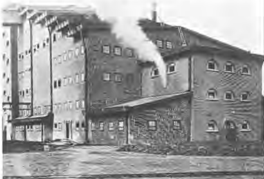
97 Poelzig, chemical plant, Luban, 1912.
