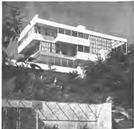
246 Neutra, Lovell Health House, Griffith Park, Los Angeles, 1927.
