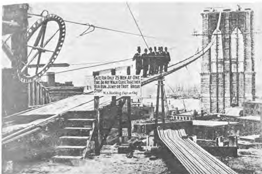
14 J. A. and W.A. Roebling, Brooklyn Bridge, New York, under construction, c.1877. Initial cable-spinning in progress.
