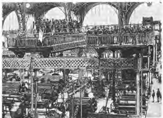
18 Dutert and Contamin, Galerie des Machines at the Paris Exhibition, 1889, showing the mobile viewing platform.
