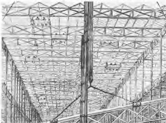
17 Paxton, Crystal Palace, London, 1851, under construction, showing glaziers' cradles.
