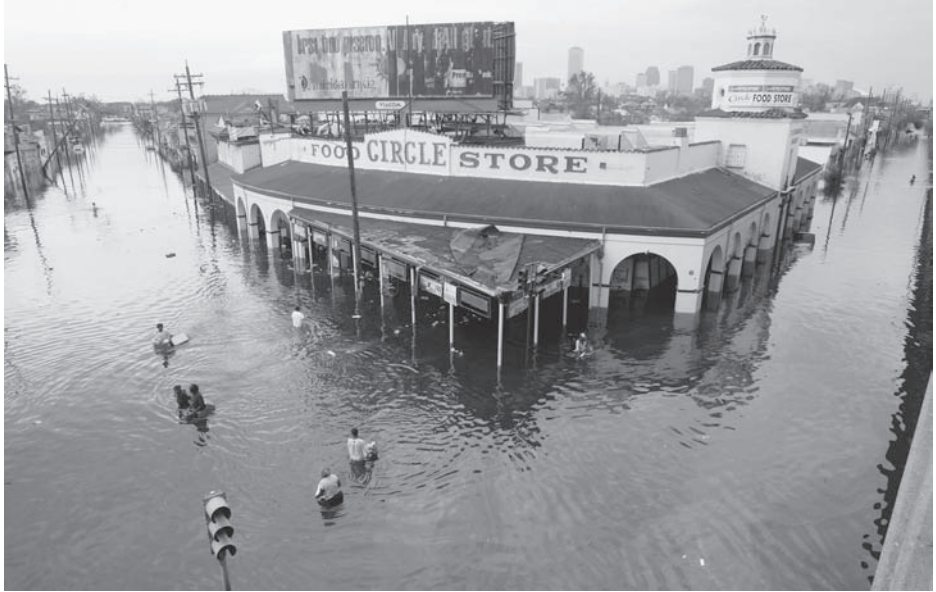
Property damage, loss of income, and other uninsured risks can ruin a business virtually overnight. AP Photo/Dave Martin.
