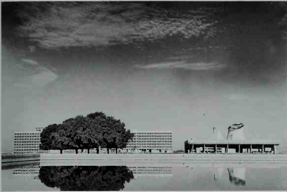
SECRETARIAT AND ASSEMBLY BUILDING. Le Corbusier with Pierre Jeanneret, Maxwell Fry, and Jane Drew. Chandigarh, India. 1952-57. The huge Secretariat building, with its sculptured forms and sun-controlled louvers, dominates Le Corbusier's plan for the new capital of Punjab.
