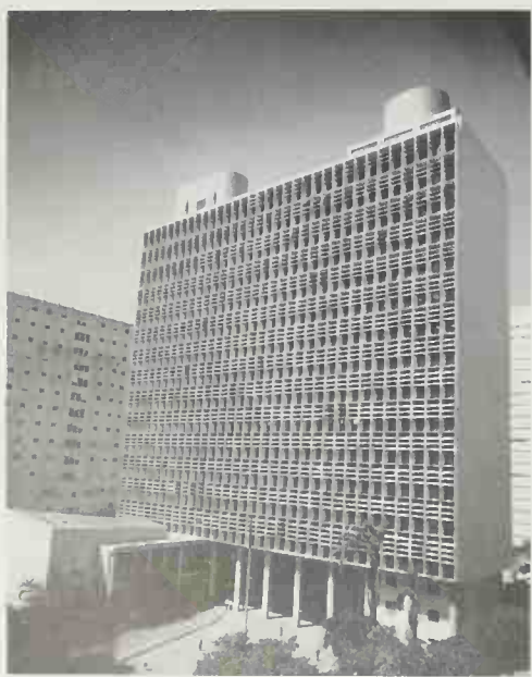
MINISTRY OF EDUCATION AND HEALTH. Lucio Costa, Oscar Niemeyer, Affonso Eduardo Reidy, Carlos Leão, Jorge Moreira, and Ermani Vasconcelos; Le Corbusier, consultant. Rio de Janeiro, Brazil. 1943. The uninterrupted, sun-shaded window walls made this sixteen-story office slab with auditorium and exhibition halls one of the most renowned examples of modern architecture in South America.
