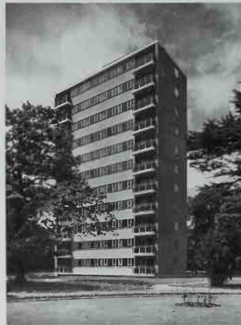
ROEHAMPTON ESTATE. London County Council. London. 1953. This London public authority created an outstanding post-war, low-cost housing development with an adept mix of high and low concrete slab buildings on a hilly park site.
