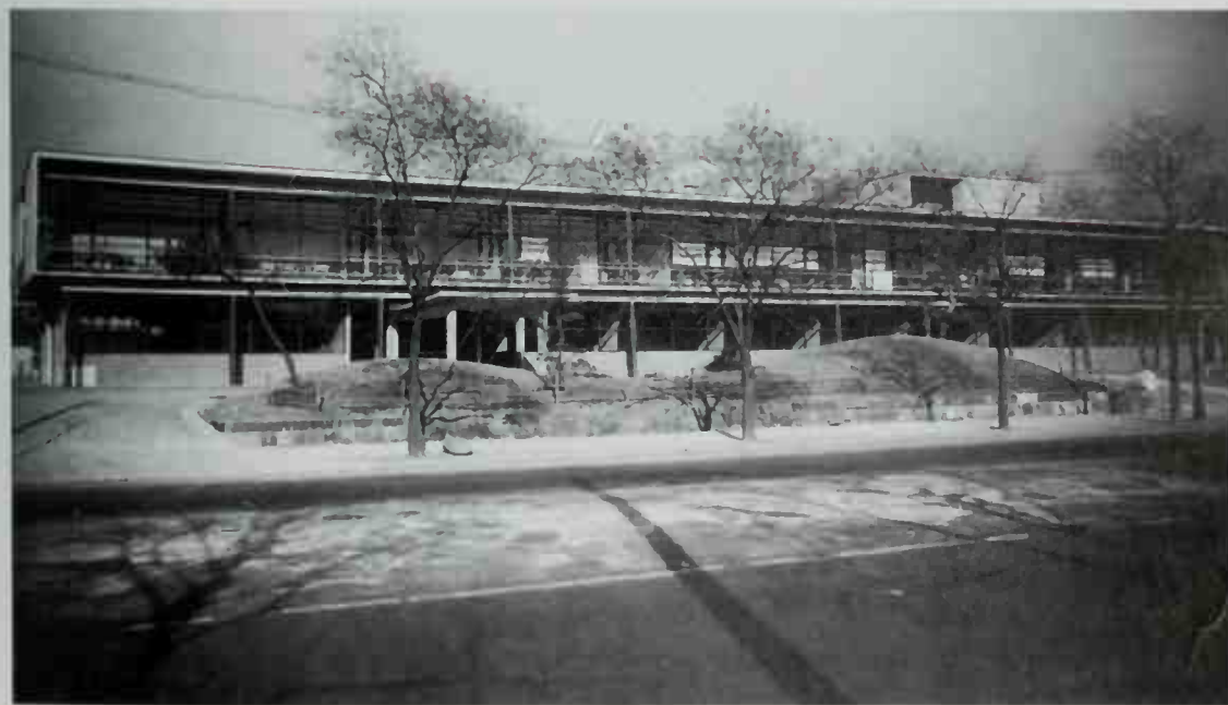
READER'S DIGEST BUILDING. Antonin Raymond with L.L. Rado. Tokyo. 1951. Considered the masterpiece of Raymond's Japanese career, this two-story office building combined modern American materials and technical innovations with traditional Japanese wood construction.
