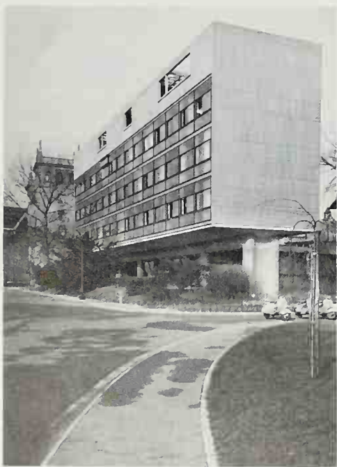
SWISS PAVILION, UNIVERSITY CITY. Le Corbusier. Paris. 1932. Elevated on sculptured concrete piers, this cantilevered residence hall for some fifty students was Le Corbusier's first major public building.
