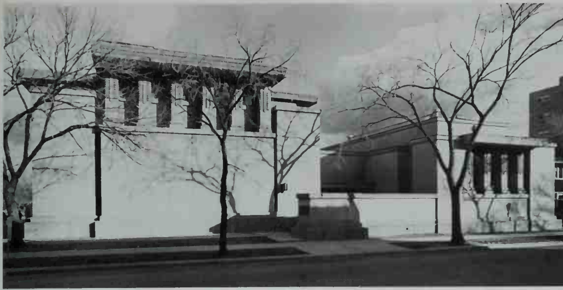
UNITY TEMPLE. Frank Lloyd Wright. Oak Park, Illinois. 1906. In America's first important poured-concrete structure, Wright broke with ecclesiastical architectural traditions. The building is divided into connected religious and social sections.
