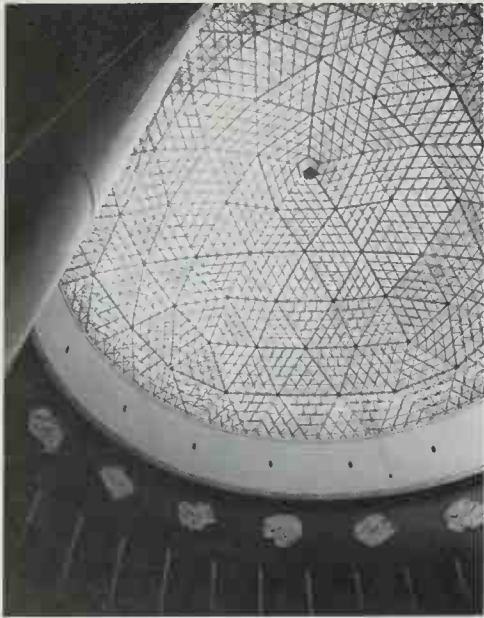
FORD ROTUNDA. R. Buckminster Fuller. Dearborn, Michigan. 1953. Erected in thirty days on an existing building, Fuller's first geodesic dome of aluminum and plastic was a celebrated structural breakthrough.
