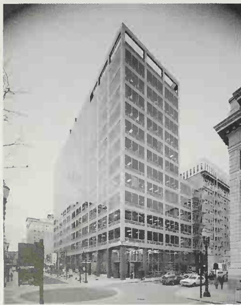
EQUITABLE SAVINGS AND LOAN ASSOCIATION BUILDING. Pietro Belluschi. Portland, Oregon. 1948. This structure was recognized as a pioneering work, both for its sleek reinforced-concrete frame, tinted glass, and aluminum cladding, and as the first sealed, air-conditioned building in the United States.
