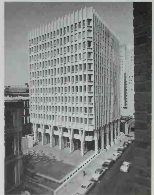
BLUE CROSS-BLUE SHIELD BUILDING. Paul Rudolph with Anderson, Beckwith, and Haible. Boston. 1960. Air-conditioning ducts and structural columns are incorporated in the verticals of the gridded precast-concrete facade.
