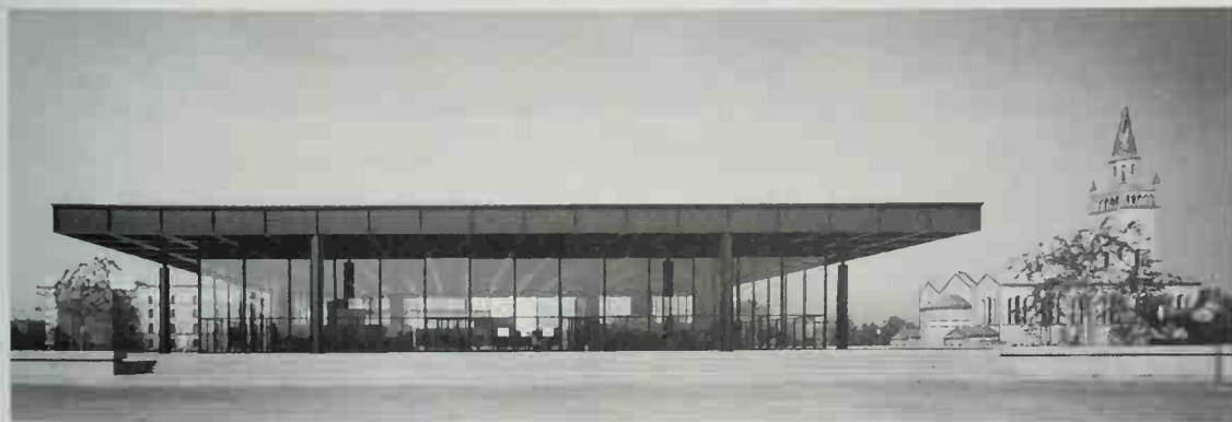
NEW NATIONAL GALLERY. Ludwig Mies van der Rohe. Berlin. 1966. This masterpiece, located in the city of his youth, was one of Mies's final works. The great steel roof is supported on eight massive steel columns erected on a lower gallery pedestal. Glass walls enclose the resulting undivided, universal space.
