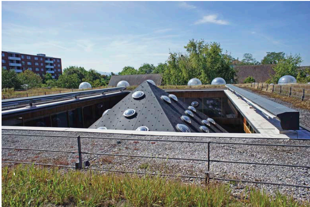
Figure 8.61 Bathhouse roof in courtyard. Source: Perry Gunther
