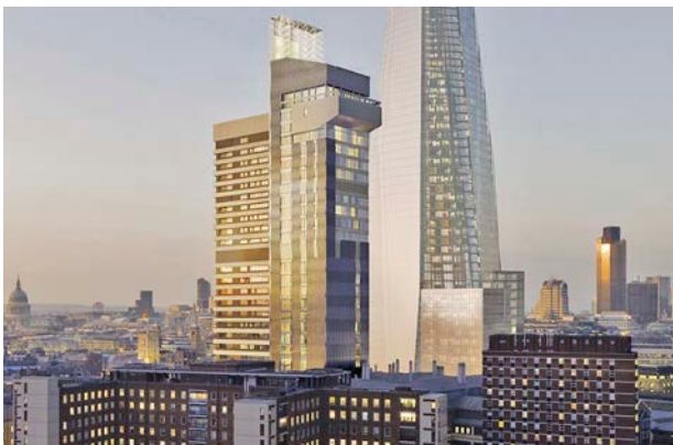
Figure 7.7 New façade elements fitted from the exterior. Source: Penoyre & Prasad
