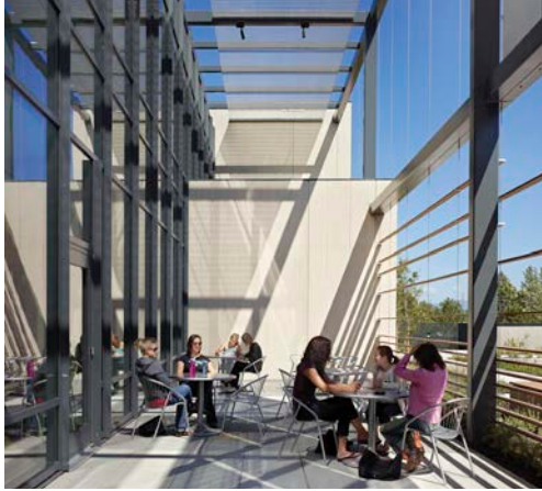
Figure 9.54 Solar shading protects full-height glazing from unwanted heat gain. Source: Copyright © Benjamin Benschneider/OTTO
