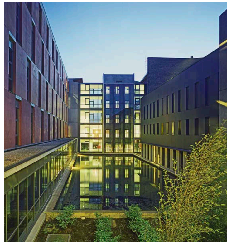
Figure 9.25 Reflective pool courtyard between bed wing and technical wing. Source: Copyright © groupe-6
