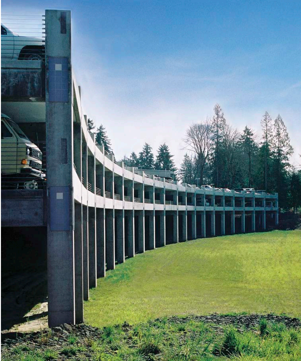
Figure 7.52 Structured parking integrated with bioswale. Source: Copyright © Eckert & Eckert
