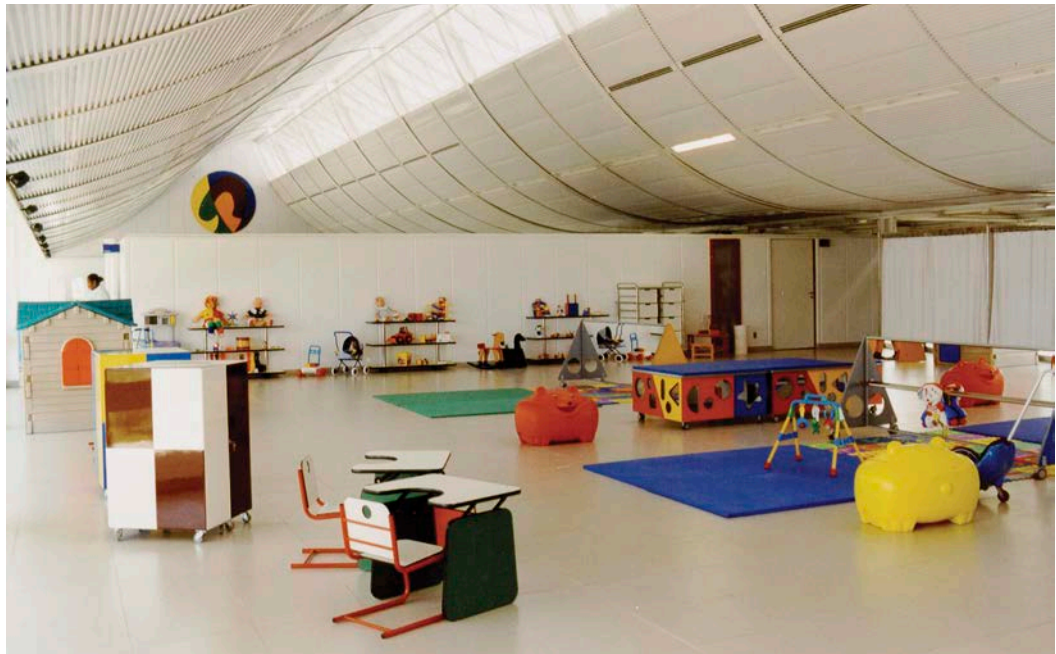
Figure 10.8 The Centro de Reabilitação Infantil, Rio de Janeiro, provides generous daylight in its physical therapy areas, using prefabricated building elements designed to maximize daylight while minimizing solar gain and facilitating natural ventilation. Source: Courtesy of the Sarah Network and João Filgueiras Lima
