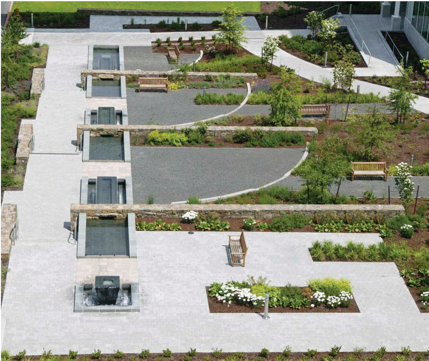
Figure 4.6 The Legacy Salmon Creek forecourt garden juxtaposes geometric and organic forms as it terraces from the entrance road beyond to the hospital entrance. Paving blocks and porous paving recharge groundwater; the water feature provides the sound of water in the court. Source: Walker Macy
