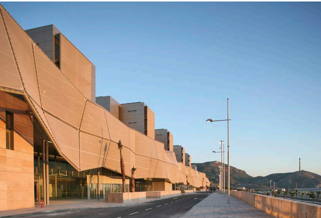
Figure 8.111 Mesh system wraps roof deck to provide continuous shading. Source: David Pernas
