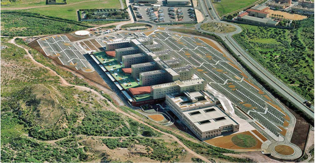
Figure 8.112 Aerial view of complex. Source: UTE Nuevo Hospital de Cartagena
