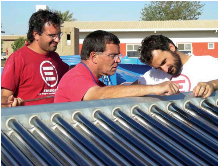
Figure 8.103 Evacuated tube solar collectors provide hot water for chillers. Source: Studio Tamassociati
