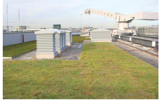
Figure 7.13 Green roof. Source: Llewelyn Davies Yeang
