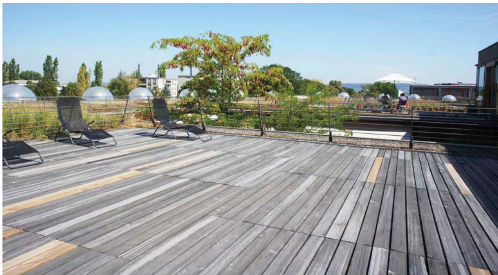
Figure 8.64 Roof deck with vegetated roof and patient room skylights. Source: Perry Gunther
