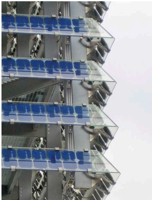
Figure 8.77 Photovoltaic shading system on research center tower. Source: Estudio Lamela Arquitectos
