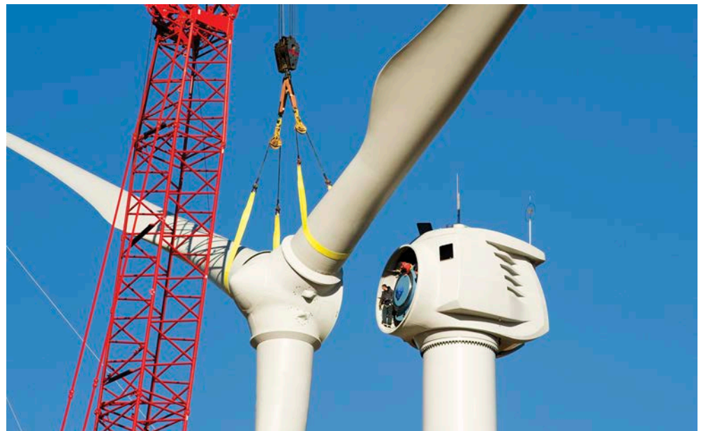
Figure 7.56 Gundersen Cashton wind turbine installation. Gundersen Health System
