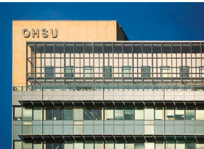
Figure 5.26 Solar air heater at 15th floor. Source: GBD Architects Inc./Interface Engineering
