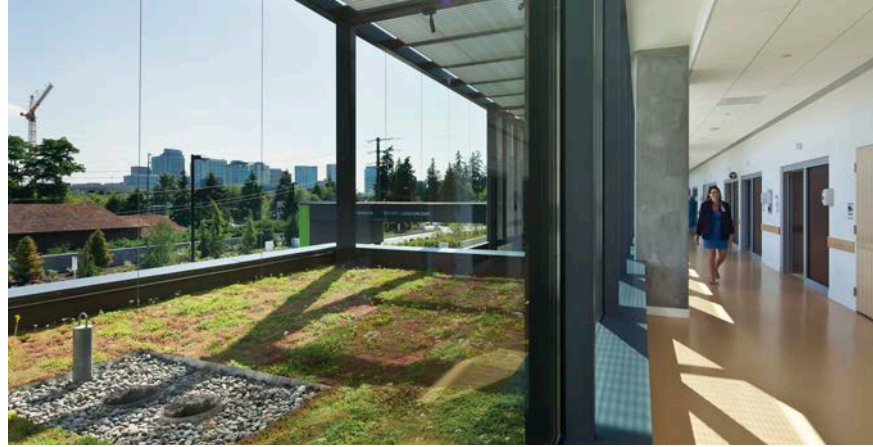
Figure 9.55 Exterior terraces inhabit facade shading system. Source: Copyright © Benjamin Benschneider/OTTO
