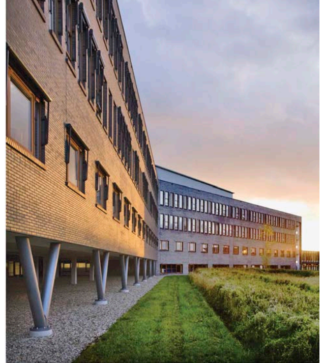
Figure 8.22 Elevated bed unit wings respond to risk of periodic flooding. Source: Phillip Driessen
