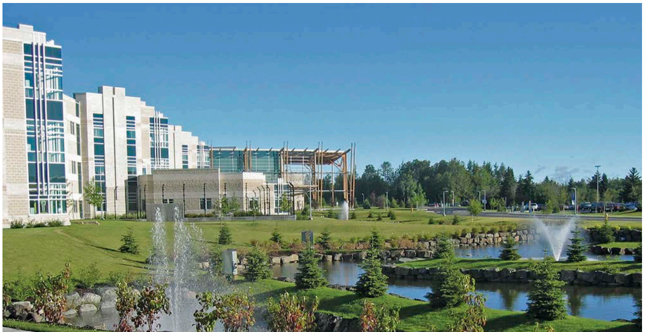
Figure 4.1 Thunder Bay uses its landscape design to support onsite stormwater retention and filtration. Source: Peter Sellar, Klik Photography
