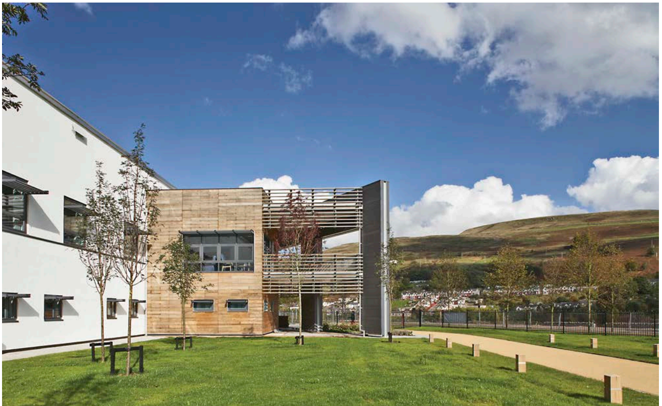
Figure 8.137 Exterior massing at the entry drive provides view of natural and salvaged material palette. Source: Charlotte Woods
