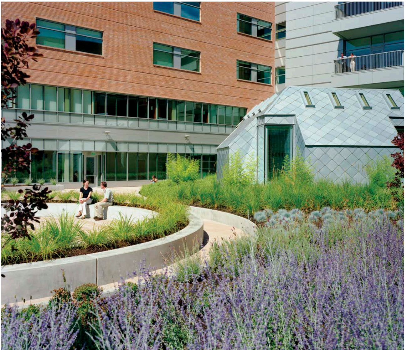
Figure 4.8 The meditation room floats in the healing garden, a landscaped roof space between the two inpatient tower wings. The garden was designed as an integral component of a horticulture therapy program. Source: Copyright © Eckert & Eckert
