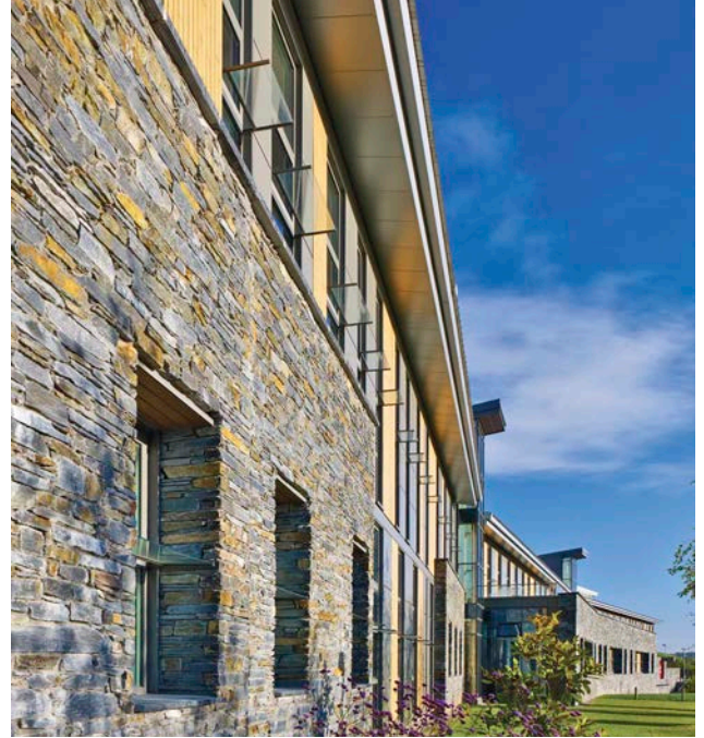
Figure 7.26 Exterior detail with local stone. Source: Copyright © Timothy Soar Photography
