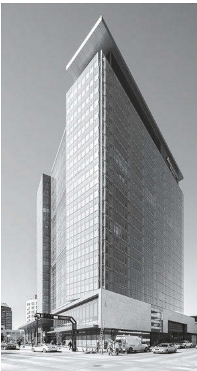
Manitoba Hydro Place, south-east corner view
