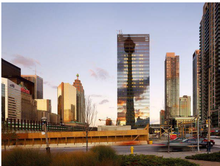
East view (bottom) and south-west view at Bremner Boulevard and York Street (opposite)
