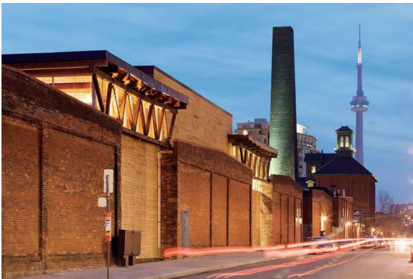
North elevation looking west (bottom); view of lobby (opposite)
