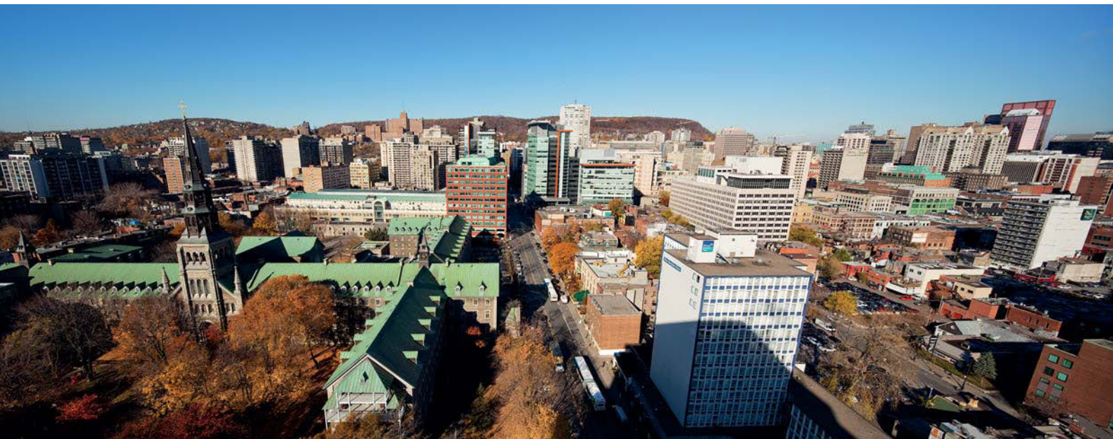
View looking north to Mont Royal (bottom); ENCS main entrance pavilion; below-grade metro connection; lounge in atrium with connecting stair (opposite, left to right)
