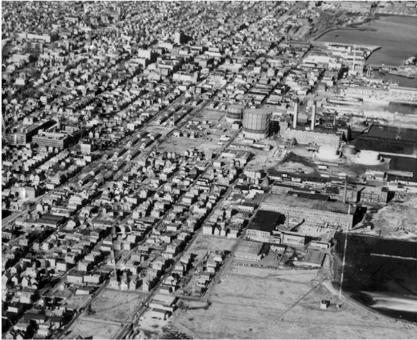
Fig. 6.1 South terminal before urban renewal project, c. 1965 (photo credit: City of New Bedford)
