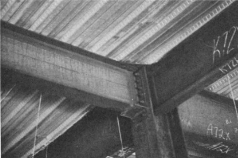
Fig. 5.3. A beam-to-column shear connection with web angles.
