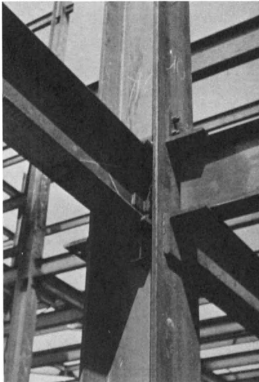
Fig. 7.4. A beam-to-column moment connection with flange angles.
