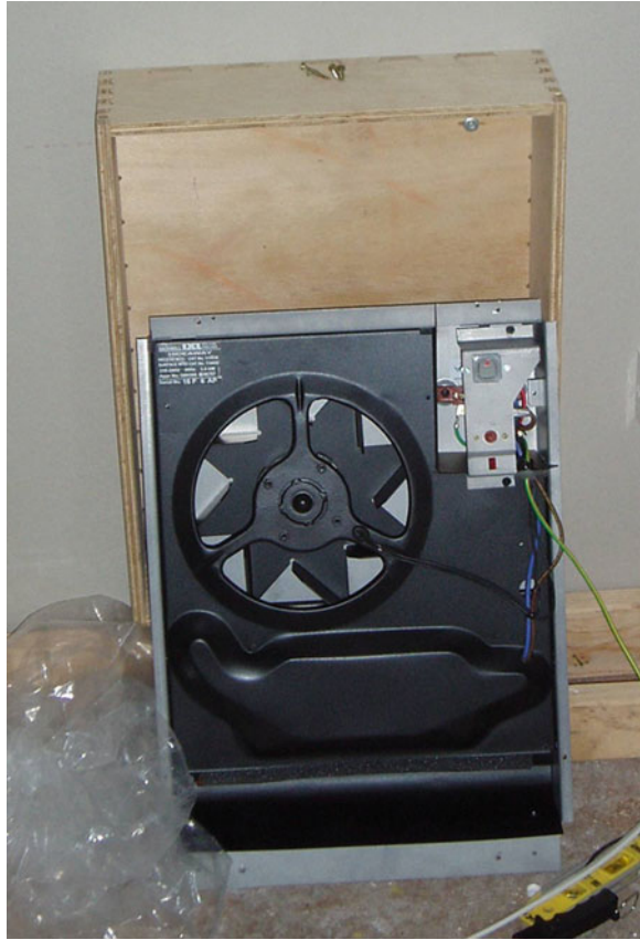
Fig. 4.61 Heater being inserted and screw-fixed into mounting box (July 11, 2006)
