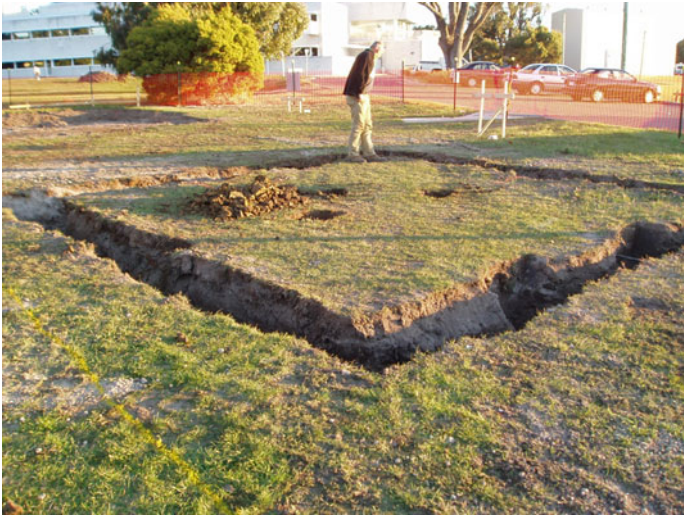
Fig. 4.29 Excavation for footings of test cell 2 (June 7, 2006)
