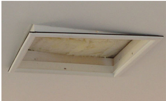
Fig. 4.45 Pushing prefabricated insert hard-up against the plasterboard ceiling (July 21, 2006)
