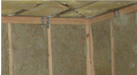
Fig. 4.74 Double top plate
