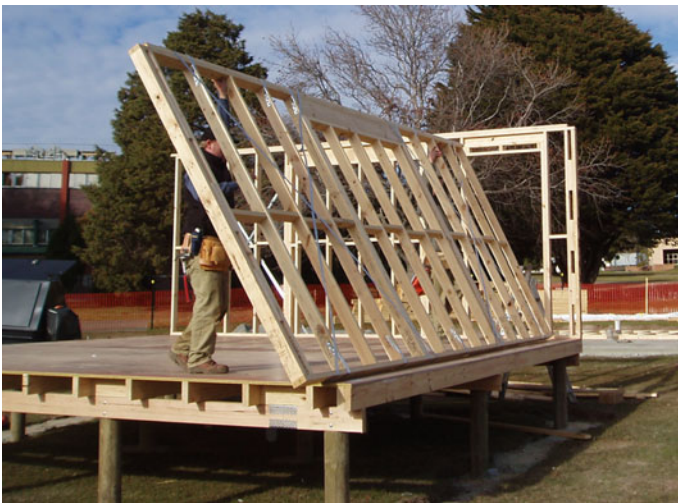
Fig. 4.31 The two-man process stage of erecting the prefabricated wall frames (June 20, 2006)
