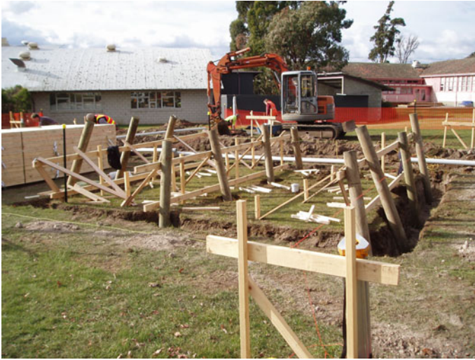
Fig. 4.30 Poles in place before concrete put in footings, test cell 2 (June 13, 2006)
