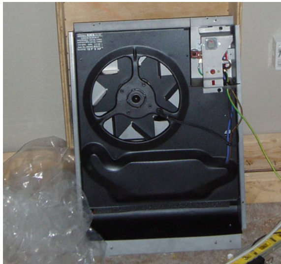
Fig. 4.103 3.6 kW wall heater being installed during thermal performance test cell construction
