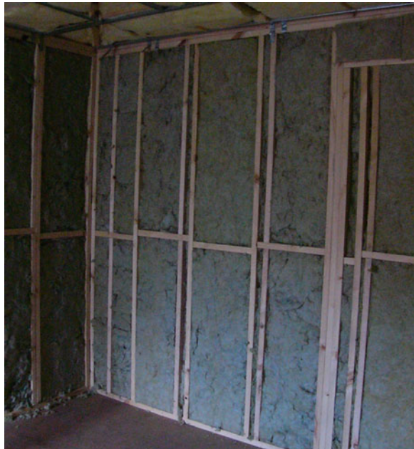
Fig. 4.72 Five additional vertical members inserted into wall for fixing plywood cladding
