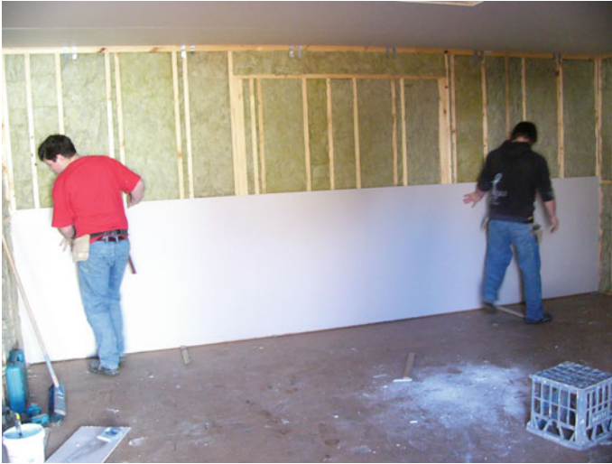
Fig. 4.38 Test cell 1—application of wall and ceiling plasterboard (July 6, 2006)
