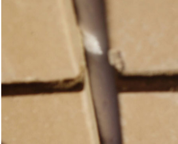
Fig. 4.51 Close up view of polypropylene rod inserted into construction joint (July 21, 2006)
