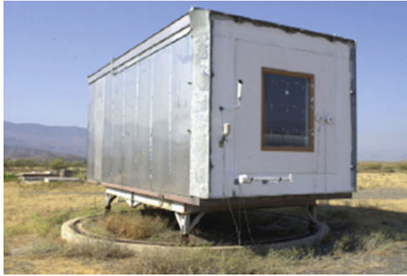
Fig. 3.9 PASSYS/PASLINK test building photograph (Jimenez and Madsen 2008, p. 157)
