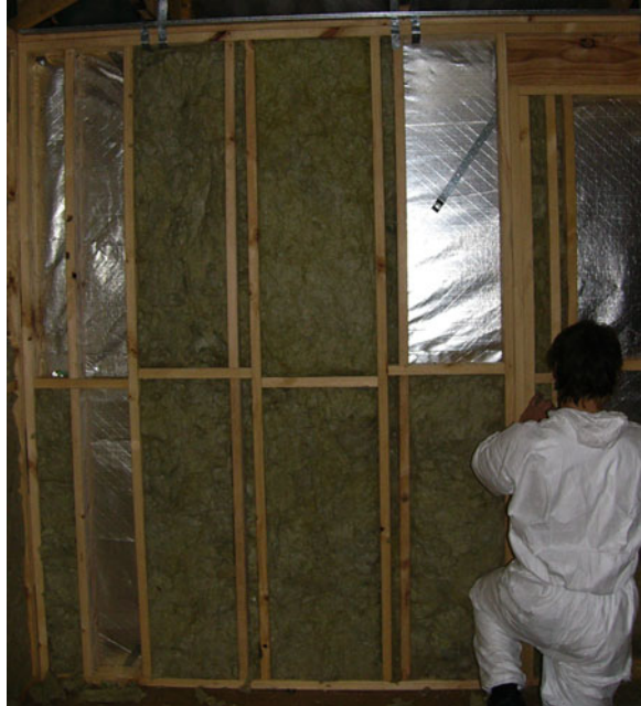
Fig. 4.71 Four additional vertical members inserted into wall for fixing plywood cladding
