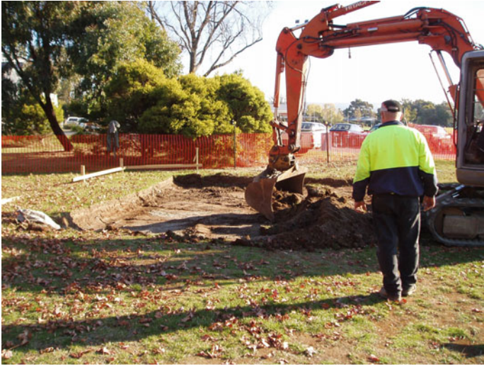
Fig. 4.28 Turning the first sod—top soil removal for test cell 3 (June 6, 2006)
