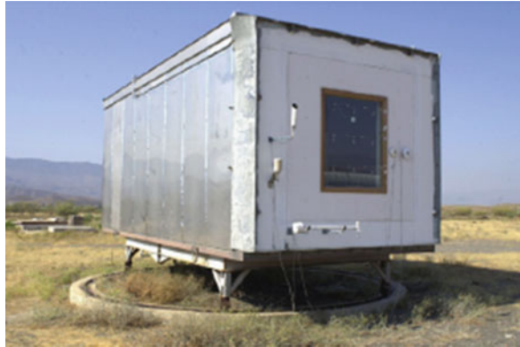
Fig. 4.80 PASSLINK test building (Jimenez and Madsen 2008, p. 157)
