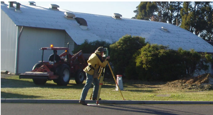
Fig. 4.24 Surveyor establishing site co-ordinates
