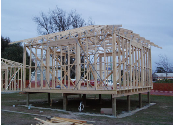
Fig. 4.32 Roof trusses erected on test cell 2 (June 21, 2006)
