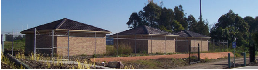
Fig. 4.11 University of Newcastle test buildings (photograph courtesy of Dr. Heber Sugo)
