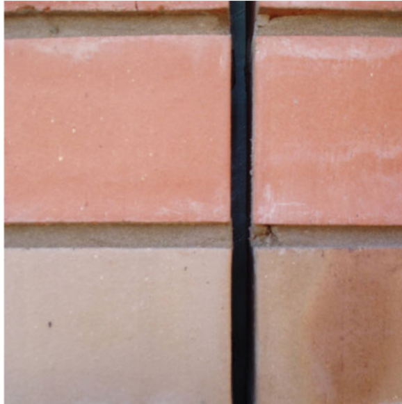
Fig. 4.53 External flexible sealant in construction joint (July 21, 2006)
