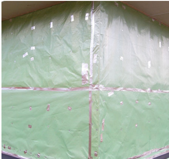
Fig. 4.65 Reflective foil tape repairs to building wrap during construction
