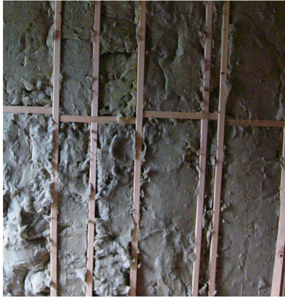
Fig. 4.70 Insulation installation in test cell 1—third attempt
