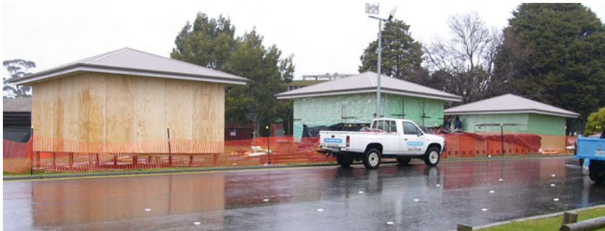
Fig. 4.37 Another rainy day halts external works (July 5, 2006)
