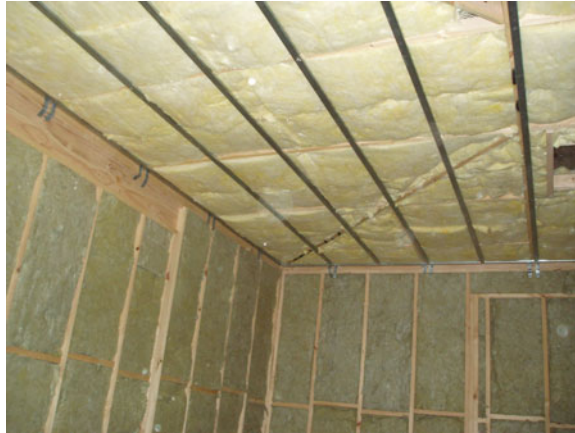
Fig. 4.36 Test cell 3—glasswool ceiling batt insulation installed (July 6, 2006)
