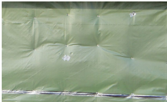
Fig. 4.69 Billowing of building wrap as a result of insulation installation
