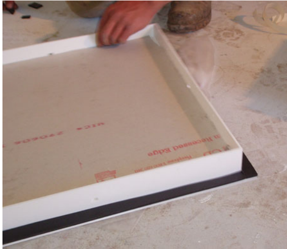
Fig. 4.44 Application of high density foam rubber tape to prefabricated insert (July 21, 2006)
