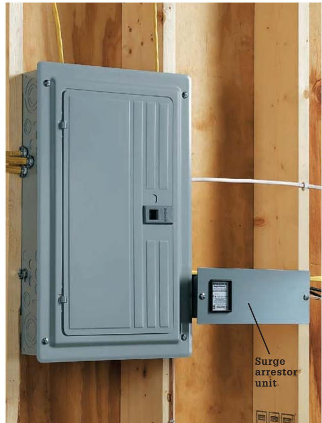
A whole-house surge arrester is an inexpensive defense against expensive damage from high-voltage shocks caused by lightning strikes and power surges. Most models install next to the main panel.
