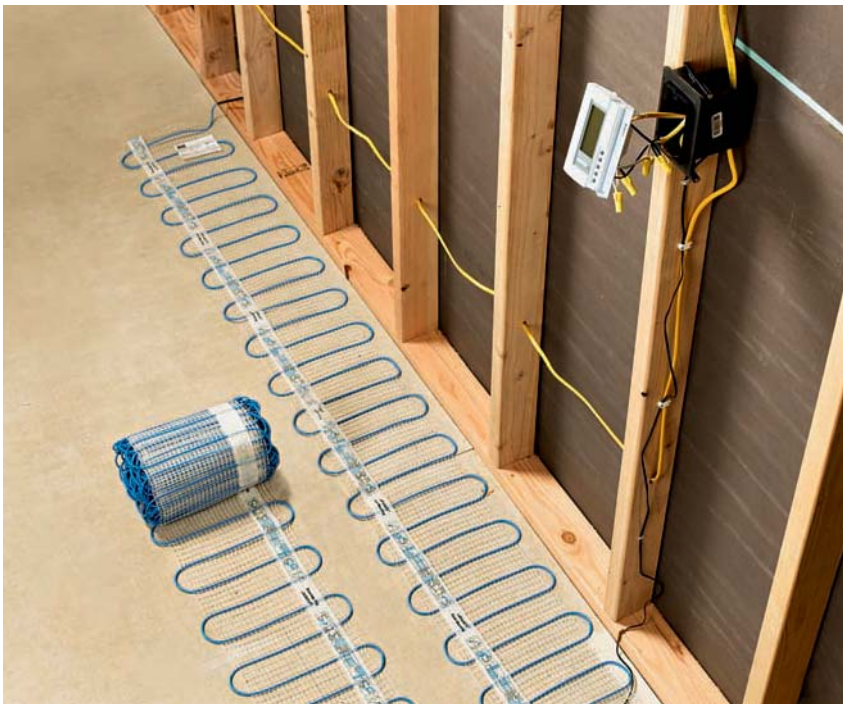
A radiant floor-warming system employs electric heating mats that are covered with floor tile to create a floor that's cozy underfoot.
