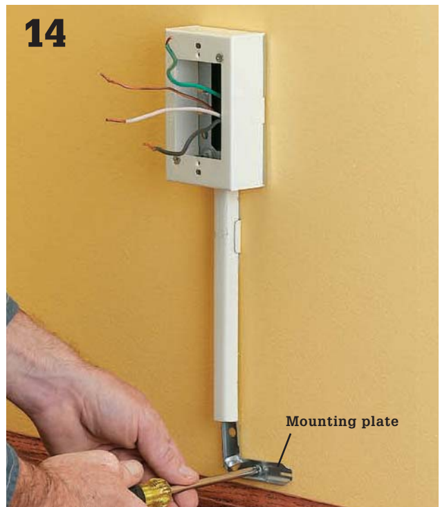
14 The elbow piece will have two parts , a mounting plate and a cap. Install the mounting plates directly below the pieces of track entering the receptacle boxes.
