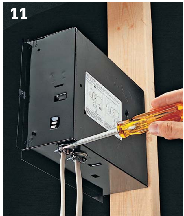
At metal boxes and recessed fixtures, open knockouts, and attach cables with cable clamps. From inside the fixture, strip away all but 1/4" of sheathing. Clip back wires so there is 8" of workable length, and then strip 3/4" of insulation from each wire.
