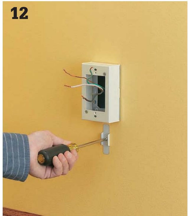
12 Install mounting clips \frac{1}{2} " or so below the knockouts on both the starter box and the new receptacle box. The clips should line up with the knockouts.
