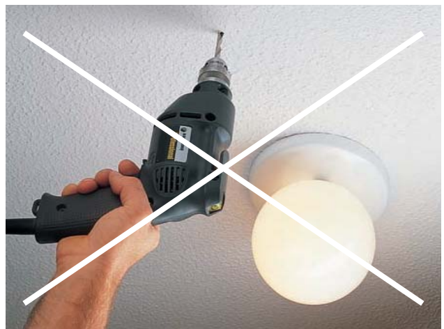
Do not penetrate walls or ceilings without first shutting off electrical power to the circuits that may be hidden.
