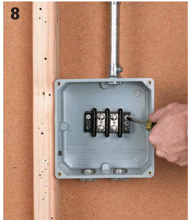
8 Mount a PVC junction box for the battery controller about 2 ft. above the battery location, and install two insulated terminal bars within the box.
