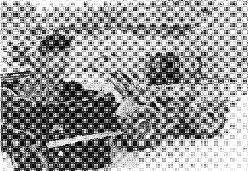
FIGURE 12-1. Soil being loaded at a borrow pit. [Ref. 7]
