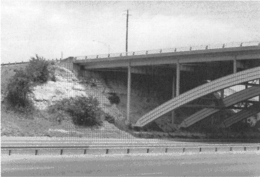
FIGURE 14-2. Hampton Road bridge over Interstate 30 bearing on bedrock. [Ref. 21]
