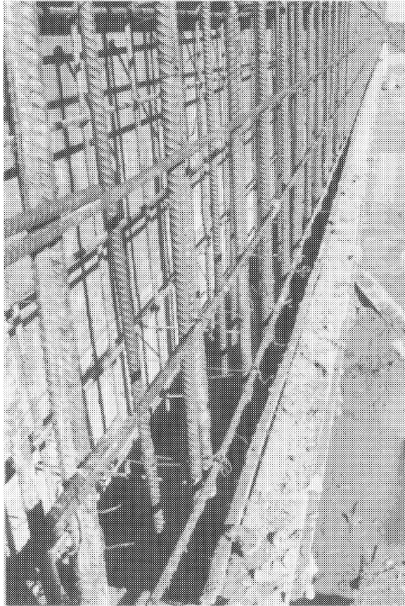
FIGURE 11-10. Reinforcing for a cantilever retaining wall. Note the heavy outside vertical bars.
