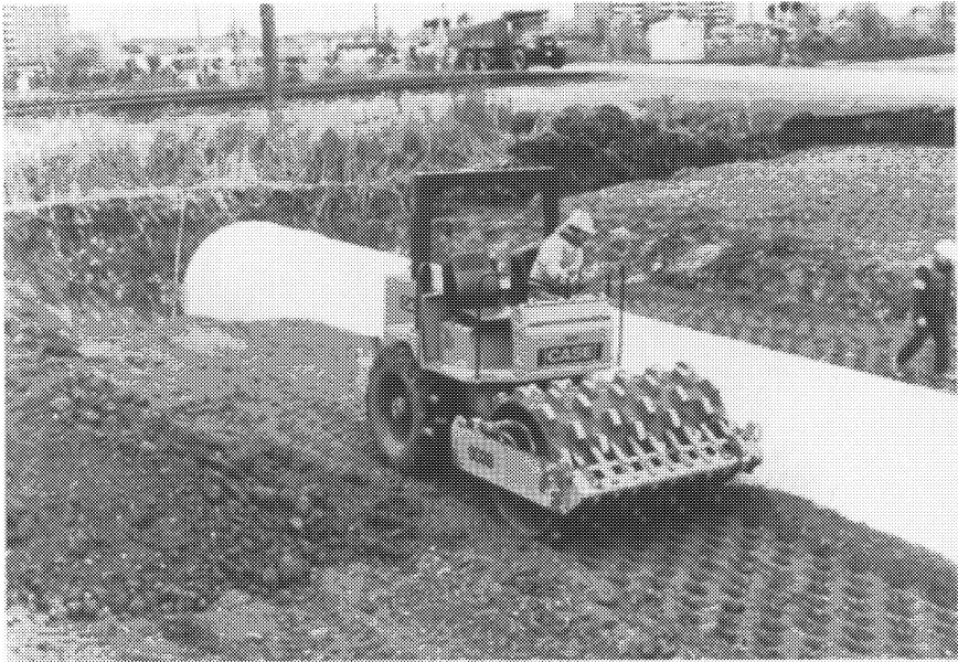
FIGURE 12-4. A paddlefoot drum vibratory roller. [Ref. 7]
