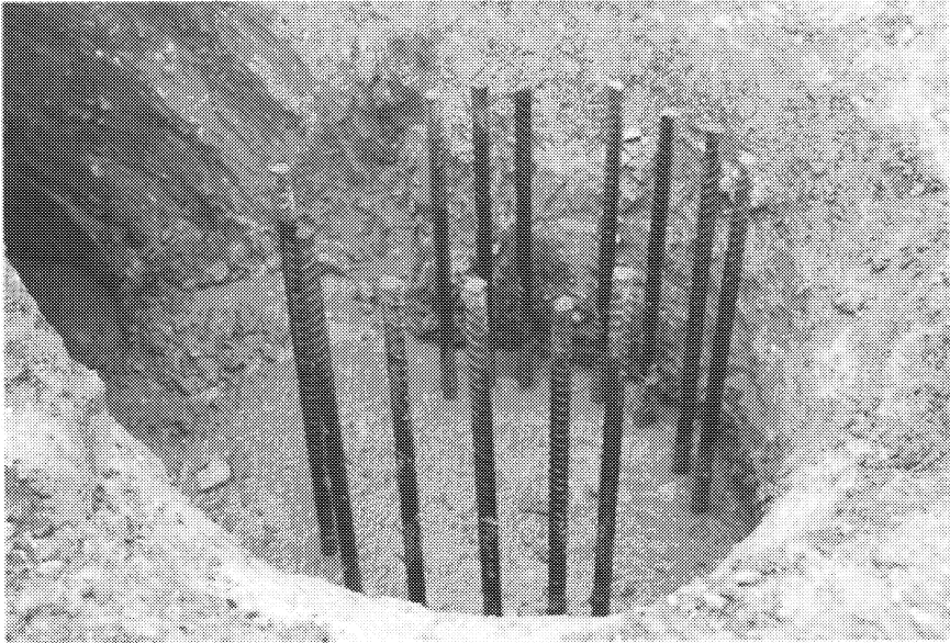
FIGURE 8-9. Placement of dowels in pier for anchorage of other elements.
