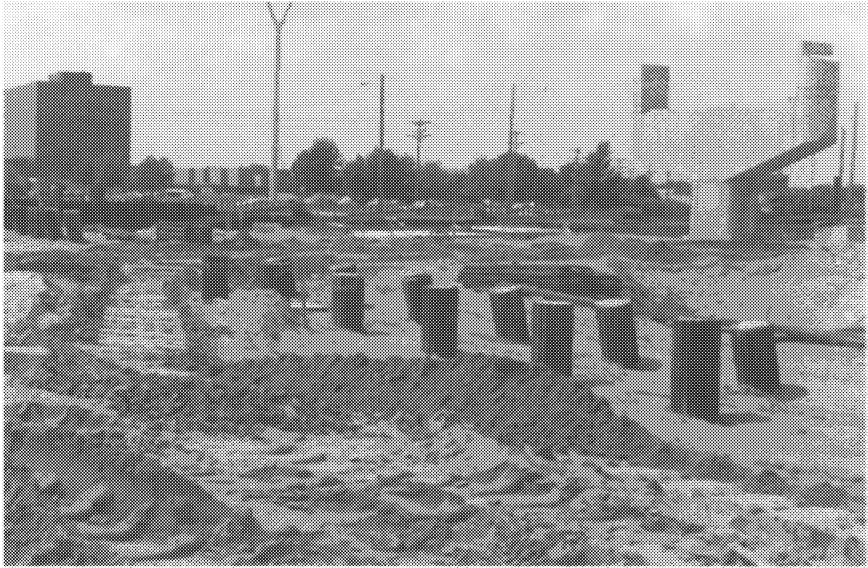
FIGURE 8-3. Typical installation of battered piles. [Ref. 15]
