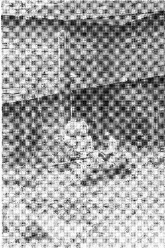
FIGURE 10-22. Rock anchor hole being drilled. [Ref. 9]
