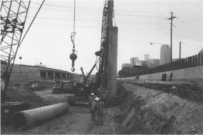
FIGURE 8-17. Installation of steel liners in pier and caisson work.
