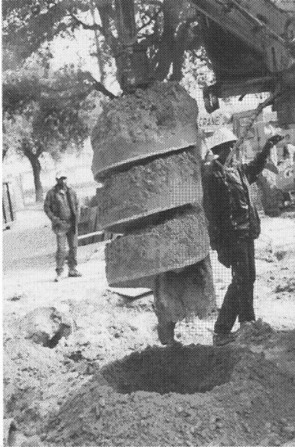
FIGURE 8-16. A large diameter earth auger used in caisson construction.
