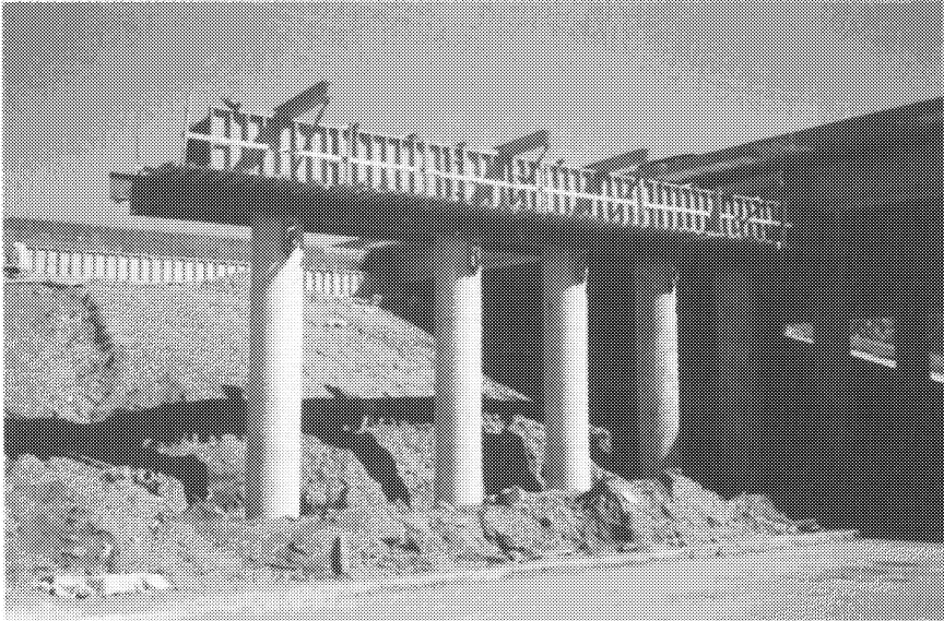
FIGURE 8-29. Exposed pier construction.
