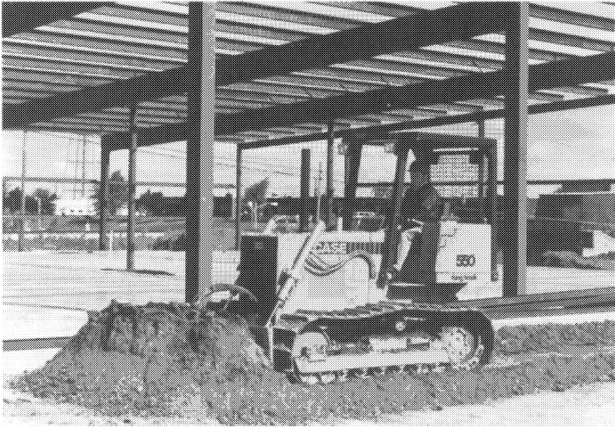
FIGURE 12-2. Spreading soil before compaction. [Ref. 7]
