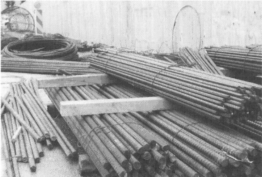
FIGURE 8-41. Example 8-8—Reinforcing grouped by size, ready for field fabrication into cages.
