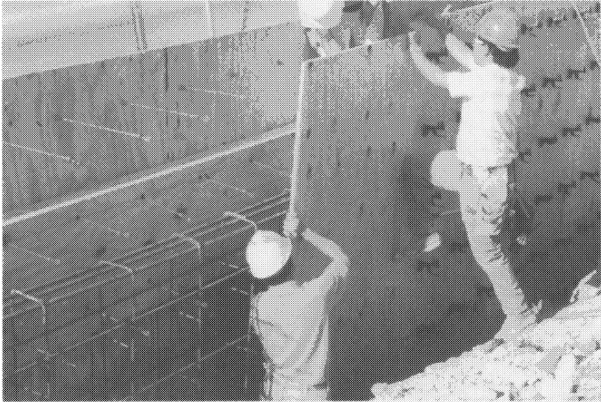
FIGURE 10-9. Formwork for a foundation wall in progress.
