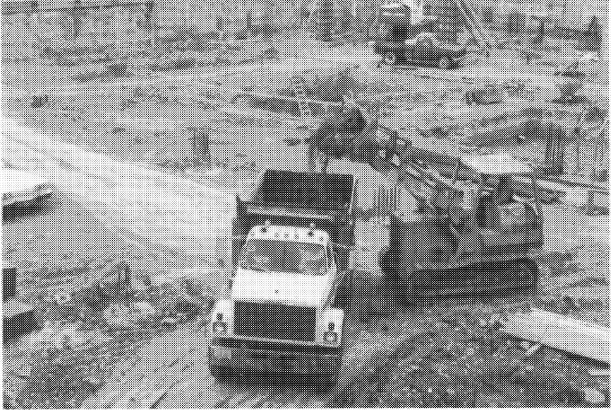
FIGURE 10-7. A typical site during construction of a major project.
