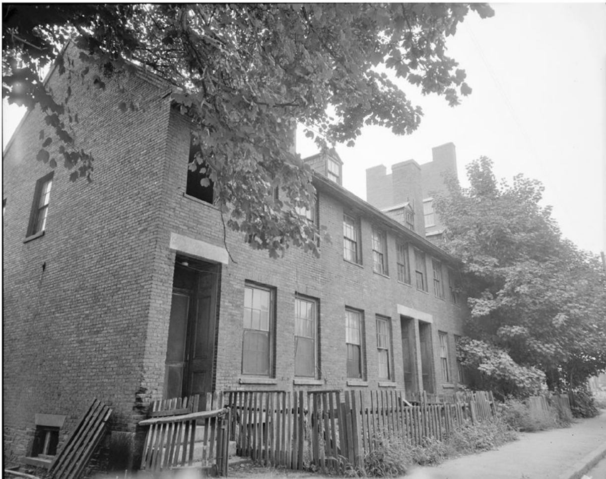
Figure 1.6 Slightly later version of the boardinghouses built in Lowell, Massachusetts, often sited near a canal or the river (circa 1840s; since demolished). Historic American Building Survey MA-1153-2, Richard Graber Photographer, 1960s
