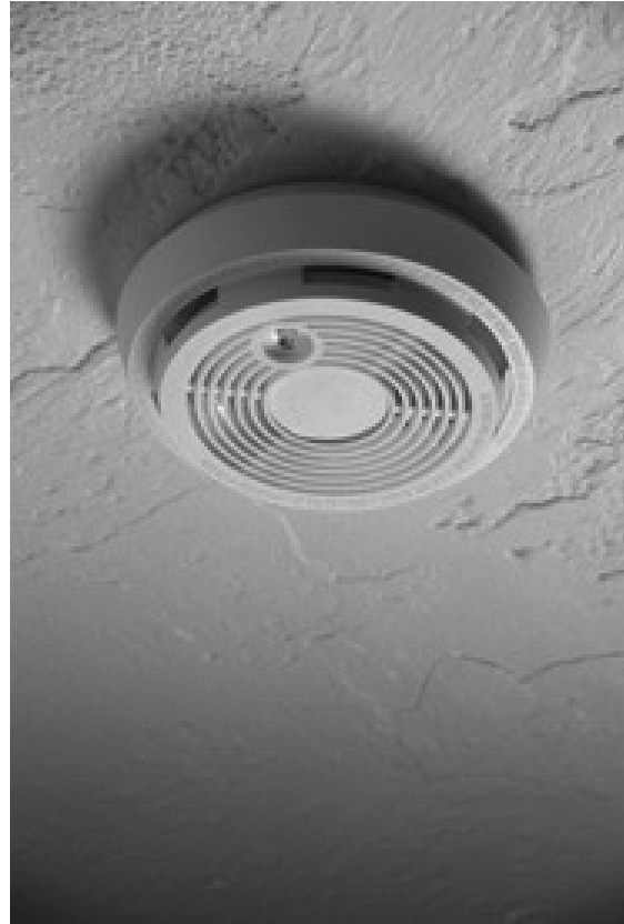
Ceiling-mounted smoke detector (can battery operated or wired to a permanent power source)
