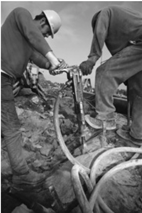
Workers using a jackhammer to break rock at a demolition site
