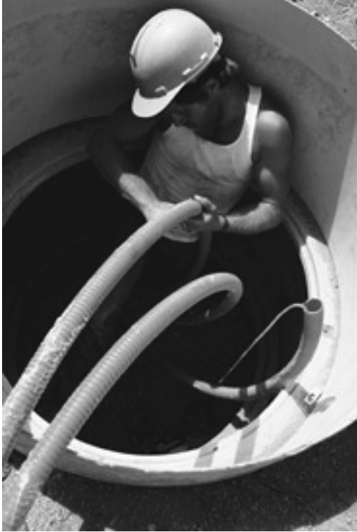
A worker prepares to enter a permit-required confined space
