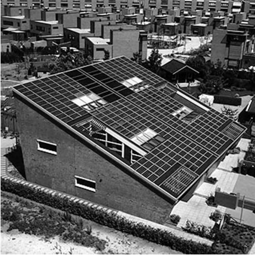
FIGURE 2.3 Roof-mounted Dutch PV subdivision, Nieuwland, in Amersfoort.
