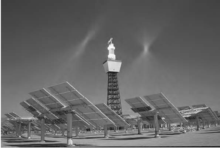
FIGURE 2.6 Warming the receiver at Solar 2 in Daguerre, CA. The “wings” on either side of the receiver result from atmospheric scattering of the sunlight reflected from the heliostat field. (Photograph courtesy of Sandia National Laboratories.)
