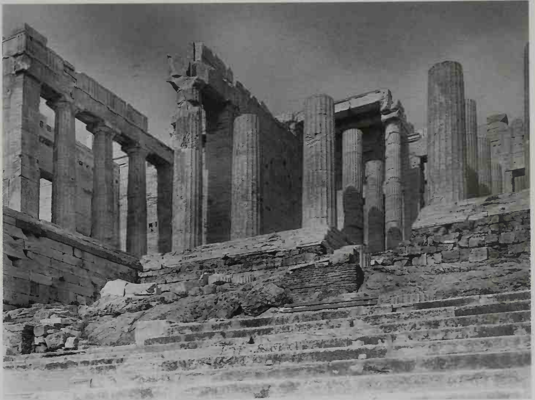
176. Athens, Propylaia, 437–432, north wing and central hall, from the west
