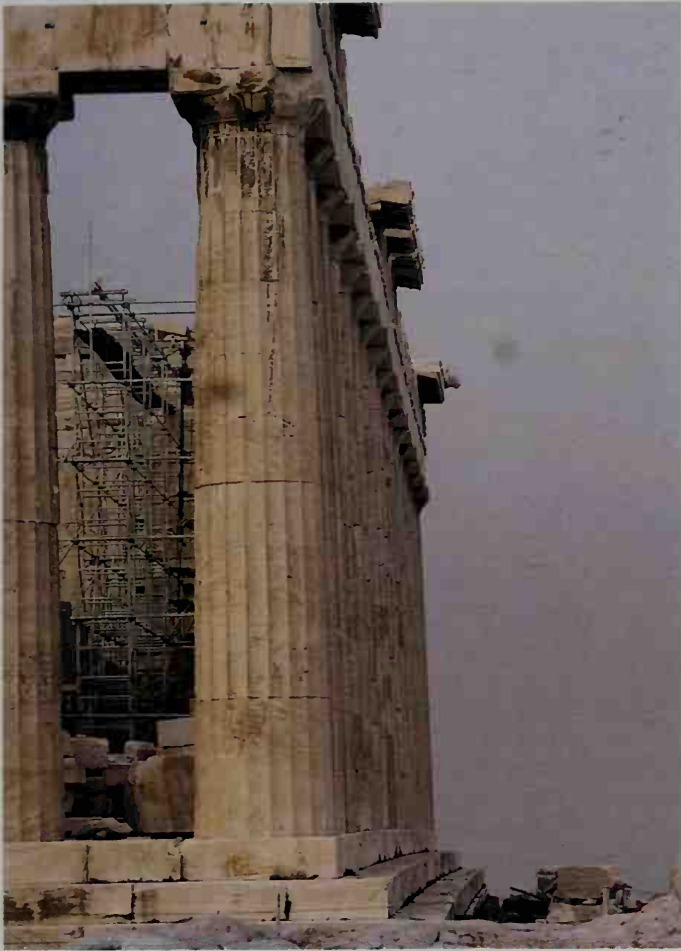
164. Athens, Parthenon, 447–432, curvature in steps
