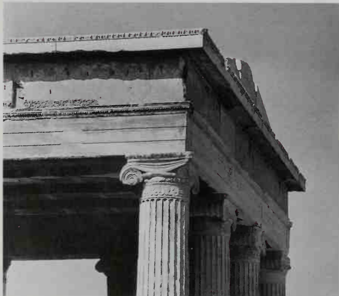
191. Athens, Erechtheion, 421–405, capitals and entablature of north porch
