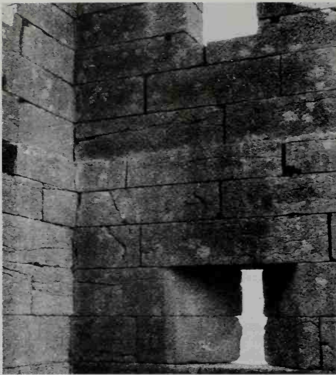
301. Messene, interior of tower near Arcadian Gate, mid fourth century
