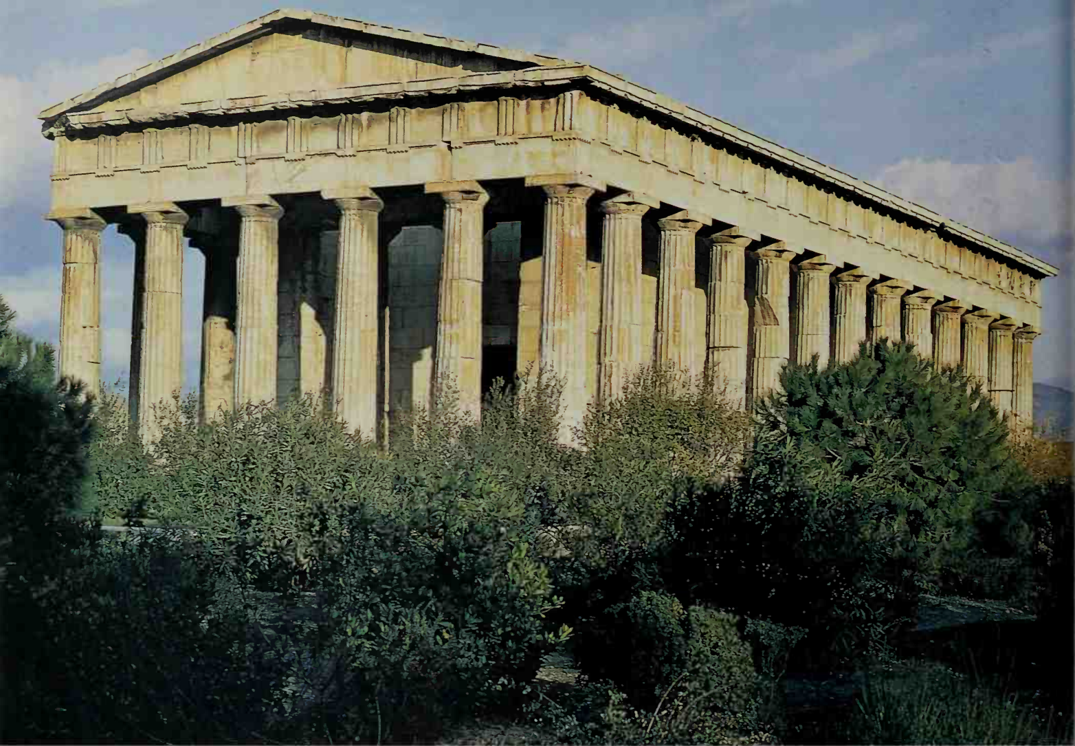
200 and 201. Athens, temple of Hephaistos ('Theseum') mid fifth century, from the south-west ( above ), and north-east corner ( below )
