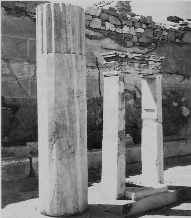
326. Delos, court with well and windlass-stand, and mural decoration, in house, probably second century
