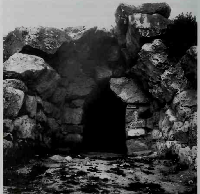
64. Tiryns, citadel, late thirteenth century, chamber in the thickness of the east wall
