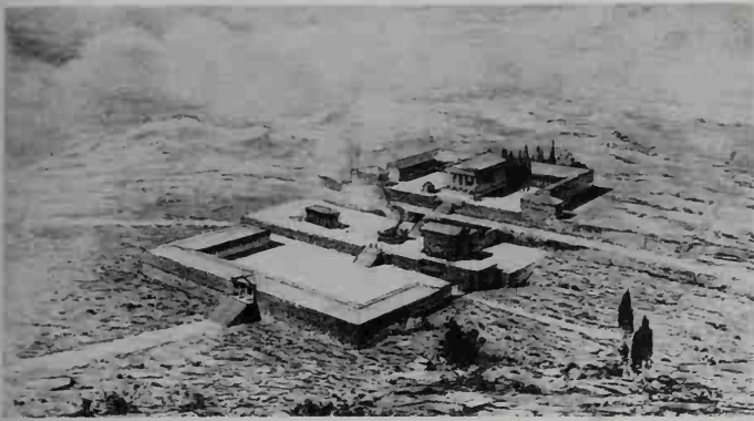
258. Kos, sanctuary of Asklepios, second century, restoration
