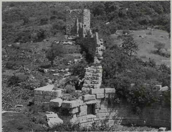
299. Messene, Arcadian Gate, north wall with tower, mid fourth century
