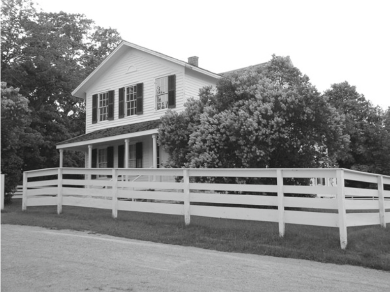
Fig. 5.13 Front facade of the superintendent’s family home in the upper-class neighborhood
