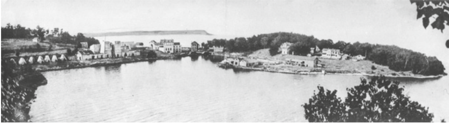
Fig. 1.5 View of Fayette townsite, circa 1907. Snail Shell Harbor is in the foreground. Notable features from left to right are several charcoal kilns, furnace complex, administrative and commercial buildings, and a knoll that housed upper and middle-class employees. Photo provided courtesy of the Michigan Historical Museum
