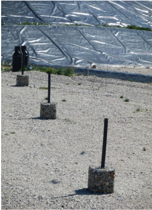
FIGURE 2.22 Sanitary landfill with biogas collection system and soil protection system. Courtesy: Valorlis, S.A.
