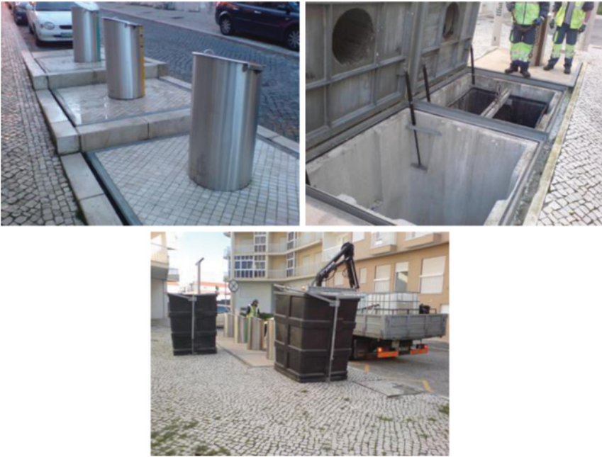
FIGURE 2.5 Underground waste containers. Courtesy: Valorlis, S.A.
