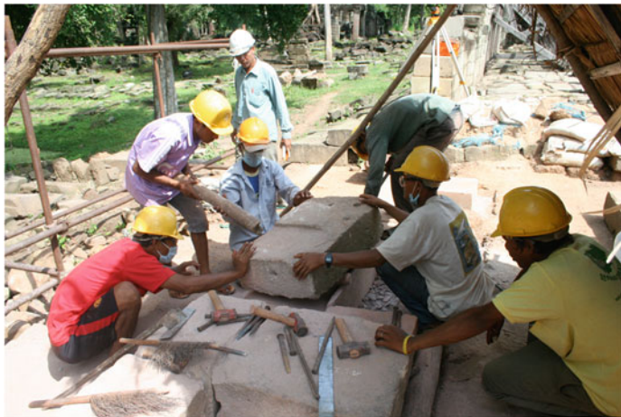
Fig. 10 Conservation of bas-relief stone blocks on site (Global Heritage Fund)
