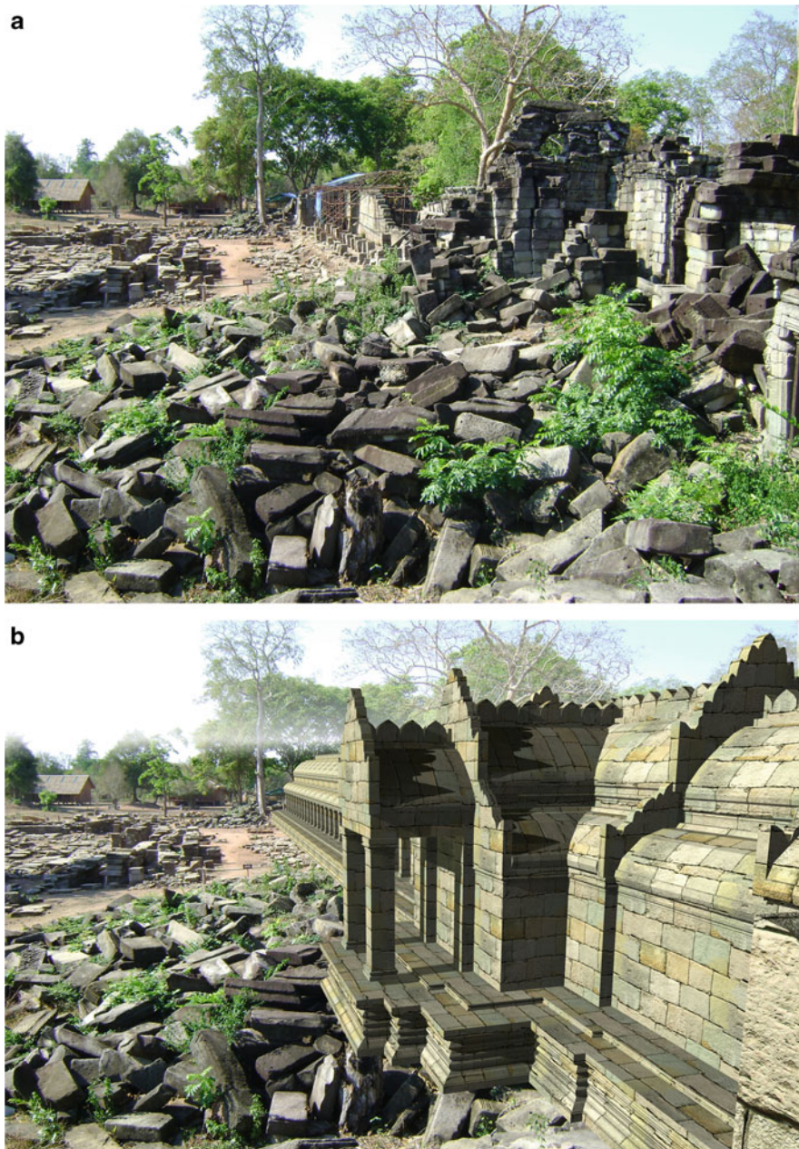
Fig. 12 (a, b) Real and virtual images of East Enclose Wall III looking south from Central Gopura (Global Heritage Fund 2012)
