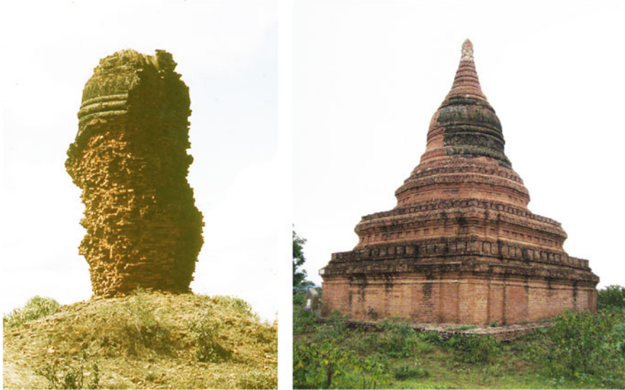
Fig. 5 Stupa 770, Pagan. Left : Condition in 1987 (Pichard 1987); Right : In 2006 after beautification. In this case, the reconstruction of missing parts has certainly prevented a future collapse of the monument. The details and proportions of the reconstructed parts are, of course, conjectural (Berliet 2006)
