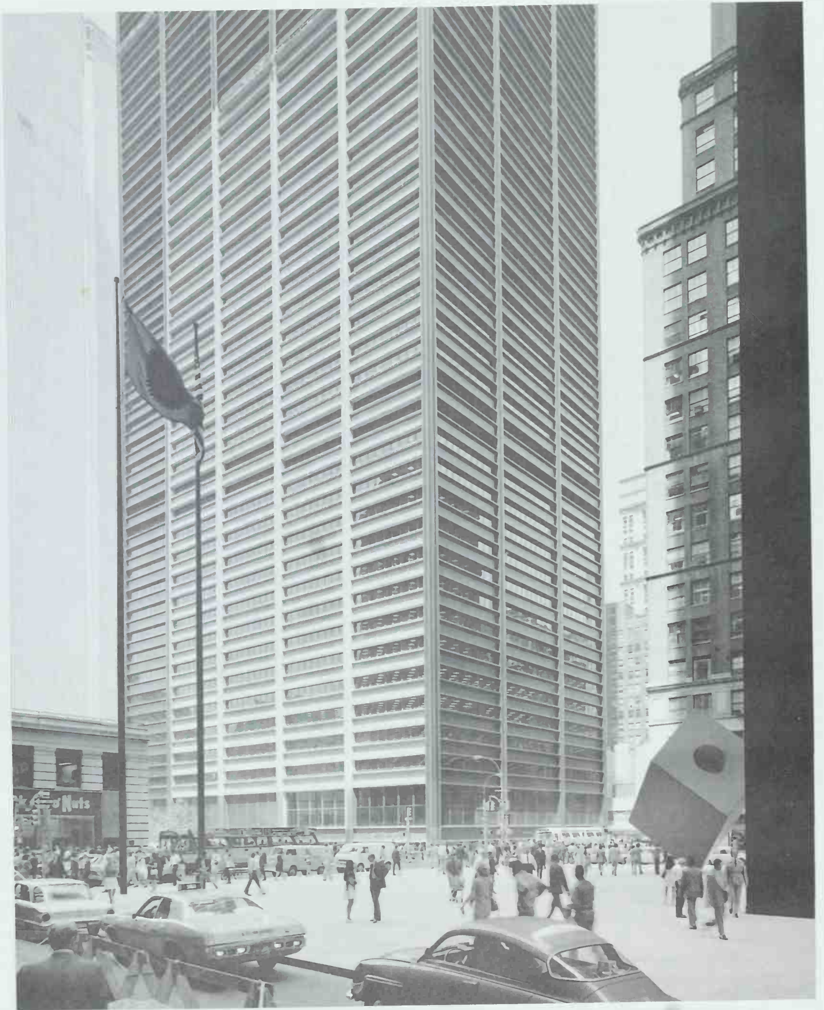
341 One Liberty Plaza (United States Steel Building); New York, New York. Skidmore, Owings & Merrill, 1970–72. Photo: Ezra Stoller, © Esto. Fifty-foot-long structural bays, six-foot-deep spandrels, and the use of special flame canopies to prevent fire-induced structural failure give the building a sense of mass exceptional for a steel-framed building.
