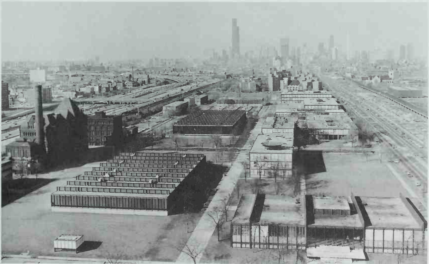
295 Illinois Institute of Technology; Chicago, Illinois. Mies van der Rohe, 1939-52 (and later). Photo: Office of Public Relations, Illinois Institute of Technology. Mies's uncompromisingly precise steel-framed buildings (seen in the right foreground) are designed on a strict twenty-four-foot module, projecting the campus's two-dimensional, right-angled plan into the third dimension.
