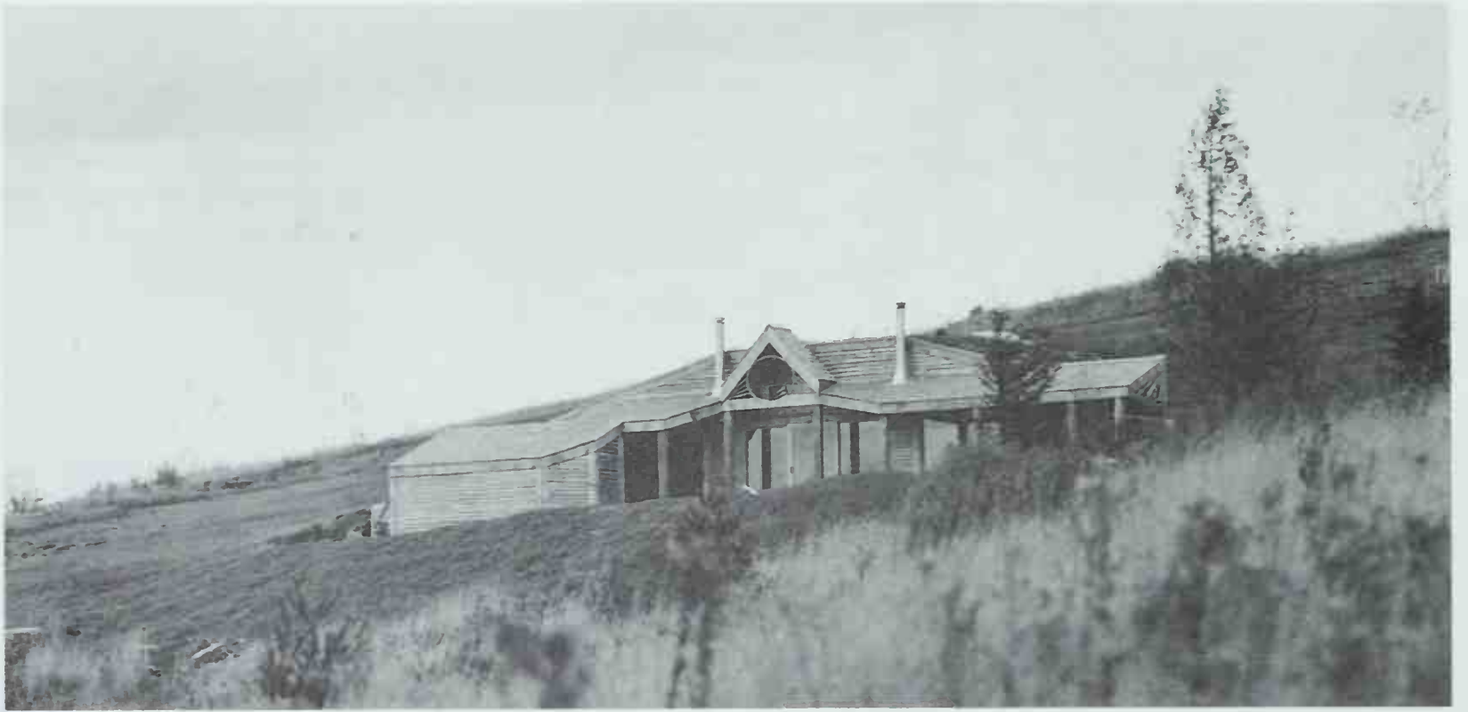
54 Crowell house; Green Mountains, Vermont. Moore Grover Harper, 1975. Photo: Robert Perron. The "handmade" aesthetic is strong in ecological design.
