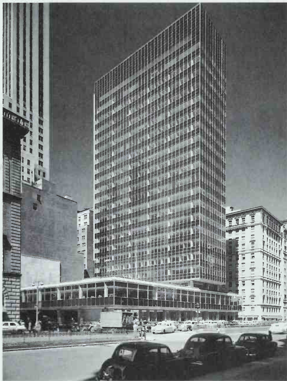
328 Lever House; New York, New York. Skidmore, Owings & Merrill, 1950–52. Photo: Ezra Stoller, © Esto. Contrasting to the heavy, ornamented masonry masses of nearby buildings, the spareness, lightness, and reflectivity of the precise green-glass curtain wall represented an explicit advertisement for modernity.
