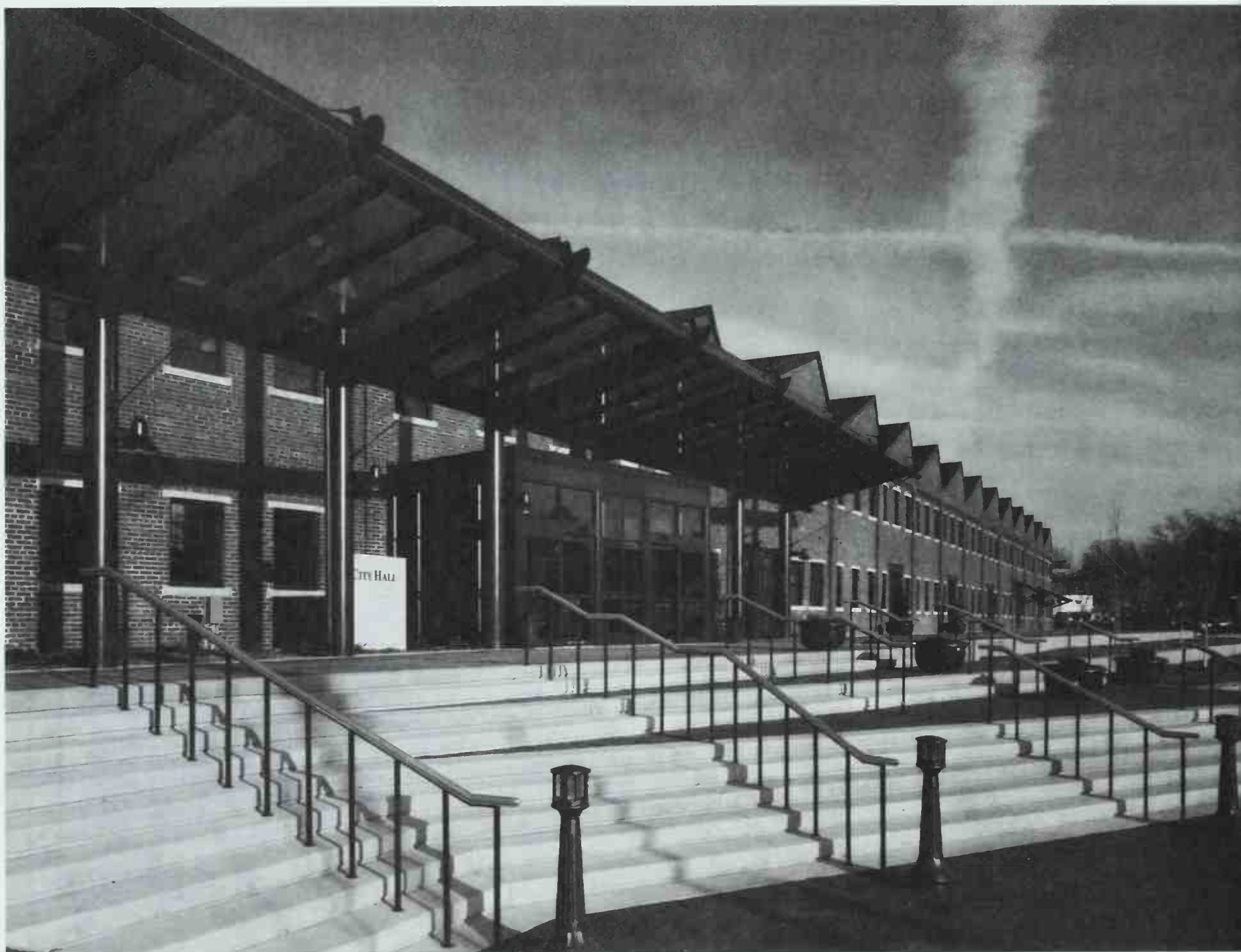
197 Showers Center; Bloomington, Indiana. The Odle McGuire & Shook Corp., 1990–95. Photo: Timothy Hursley. Sharing the facility with educational and commercial tenants, the City Hall's railroad canopy entrance signals the new civic function. Interior spaces were reconfigured to increase the level of natural light and to create double-height court spaces.
