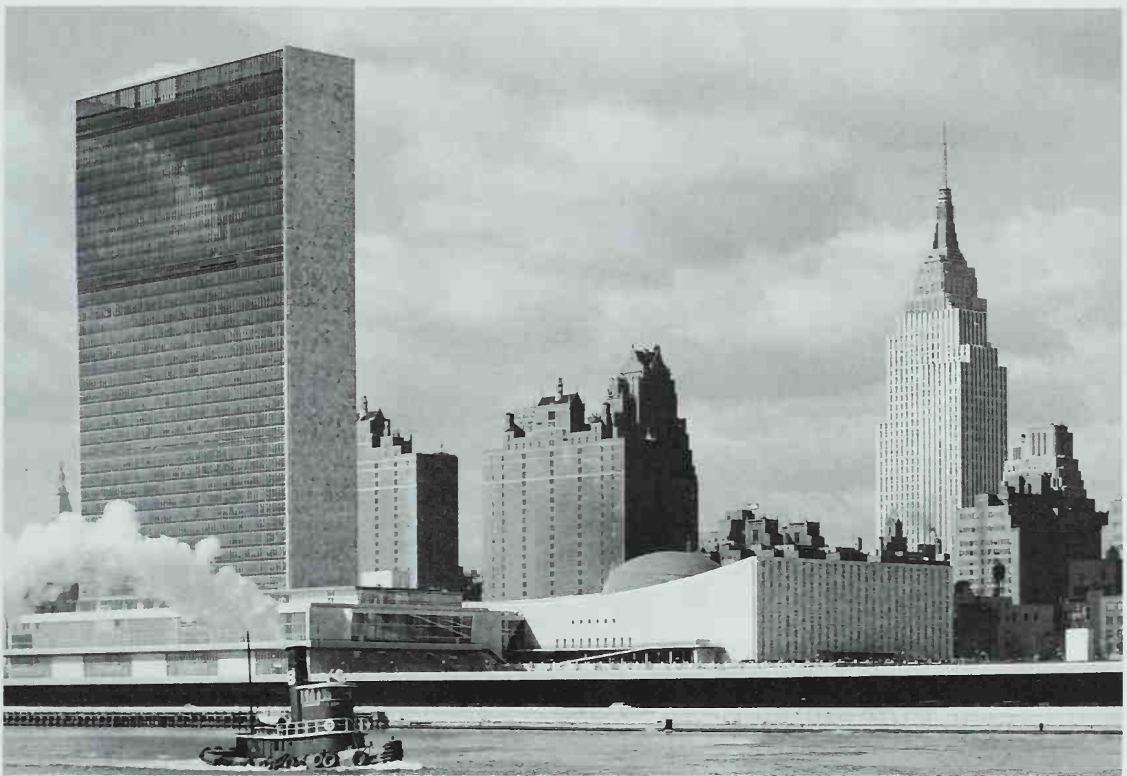
153 United Nations Headquarters; New York, New York. Wallace K. Harrison, supervising architect, 1947–50. The low silhouette of the General Assembly Building, crowned by a domelike element, sets off the insistent height and rectangularity of the tall Secretariat. Standing free in an open space, completely enclosed in tinted green glass on two long sides, the thirty-nine-story broad rectangular slab adds a bold silhouette to the skyline.
