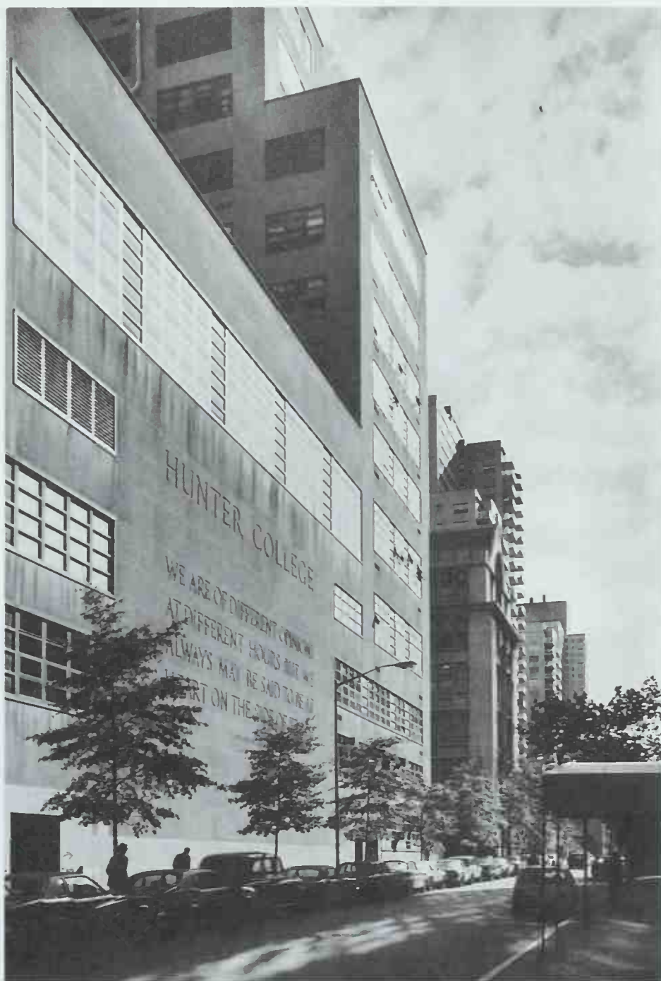
292 Hunter College; New York, New York. Shreve, Lamb & Harmon with Harrison & Fouilhoux, 1939. Photo: New York Landmarks Conservancy. The severe facade distinguishes the college from nearby apartment buildings.
