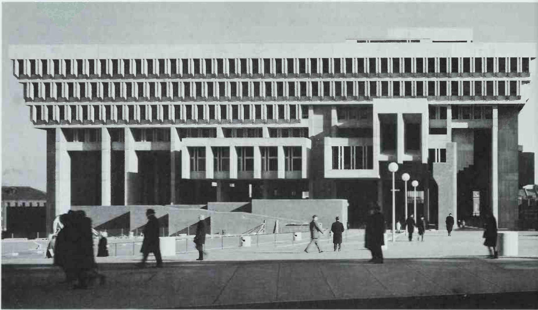
170, 171 Boston City Hall; Boston, Massachusetts. Kallmann, McKinnell & Knowles, 1963–69. Photo: © Cervin Robinson.
