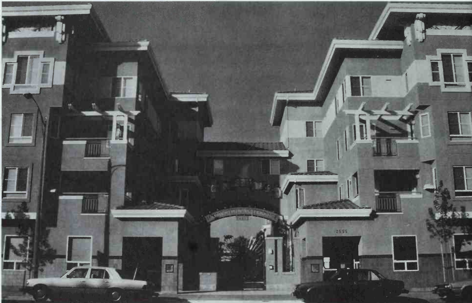
148 Hismen Hin-Nu Terrace; Oakland, California. Pyatok Associates, 1995. Photo: Michael Pyatok. Strongly articulated and embellished with decorative detailing and artwork, the building asserts the occupants' individuality. Through the gateway, interior open space is divided into three courtyards that serve neighborly activities.
