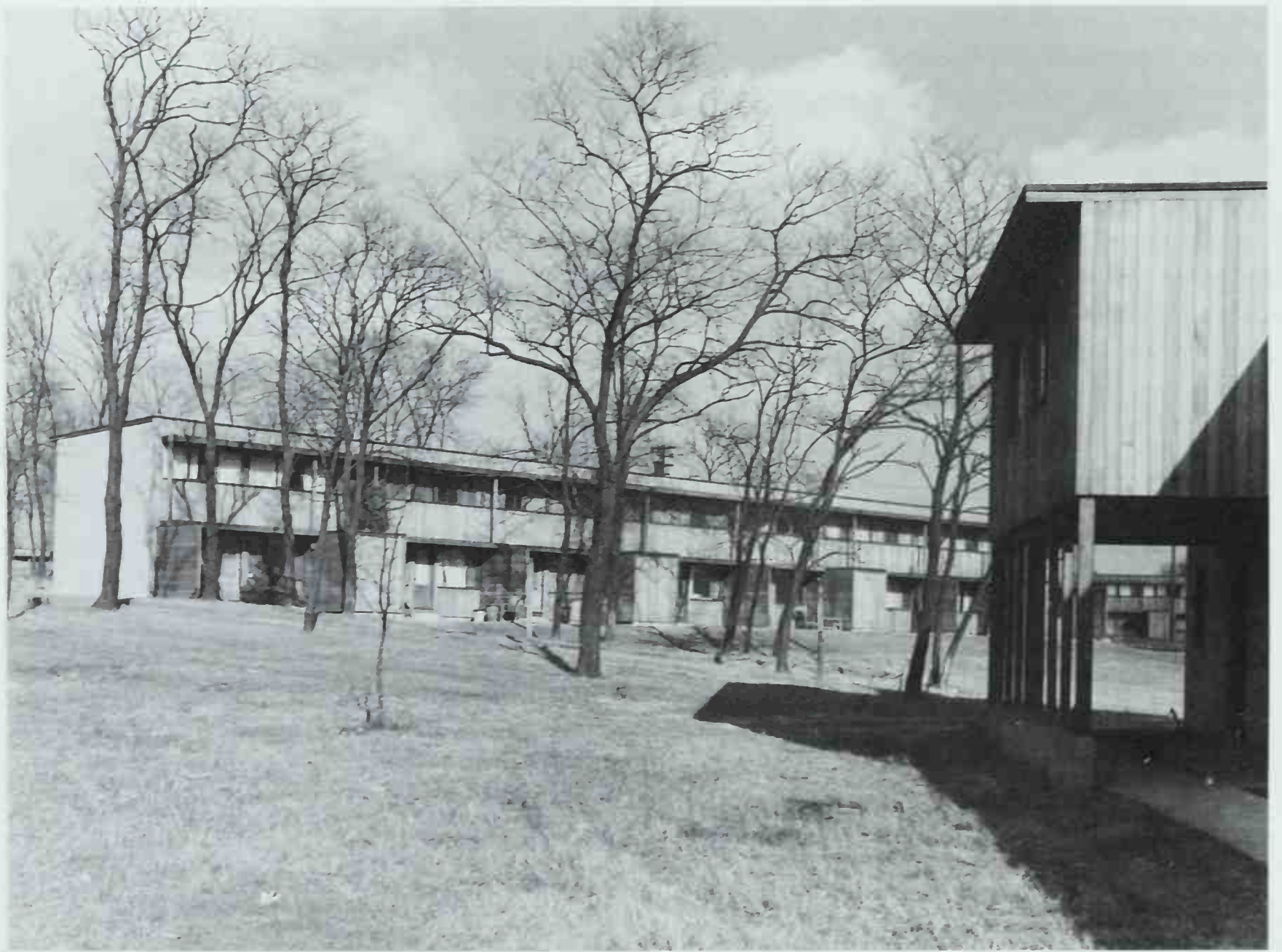
127 Aluminum City Terrace; New Kensington, Pennsylvania. Walter Gropius and Marcel Breuer, 1943. Photo: Gottscho-Schleisner Collection, Library of Congress. In terrace formation on a hillside site, the project consisted of 250 strictly Modernist row houses demonstrating open interior planning and modular construction technology.
