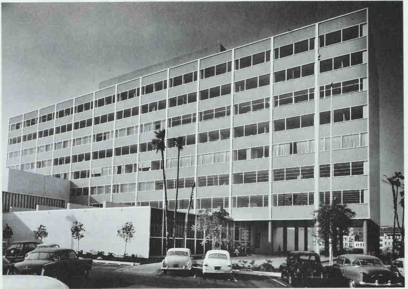
155 Police Station, Civic Center; Los Angeles, California. Welton Becket Associates, 1955. Photo: Julius Shulman. Exposed framing raises upper stories above the recessed base, an intentional contrast to the rootedness of traditional masonry.
