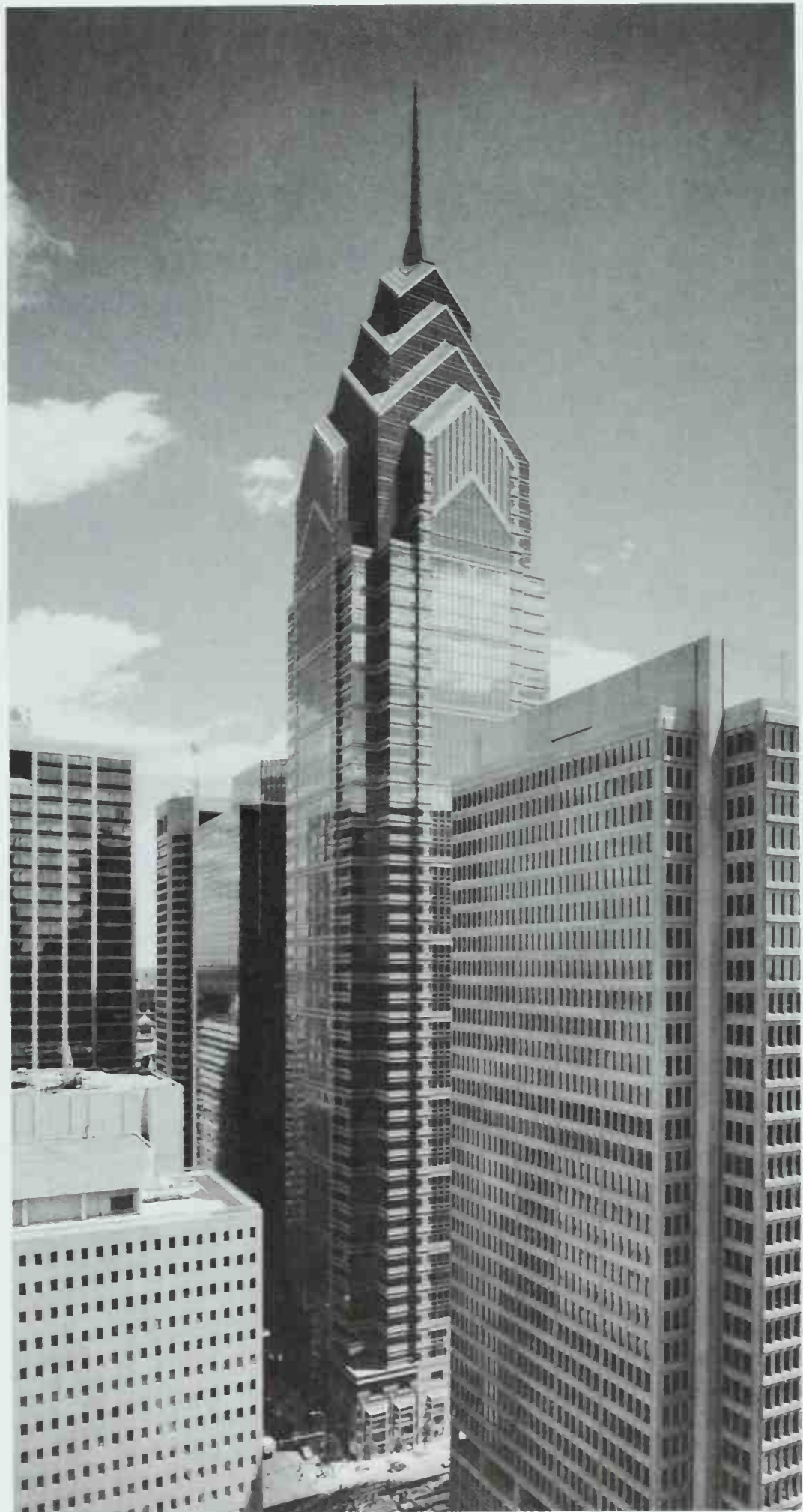
369 One Liberty Place; Philadelphia, Pennsylvania. Murphy/Jahn, 1984–87. Photo: Lawrence S. Williams, Inc. The position of the stone on the facade is emblematic of the underlying structure, while the triangular “wedding-cake” top is intended to create a glamorous effect.
