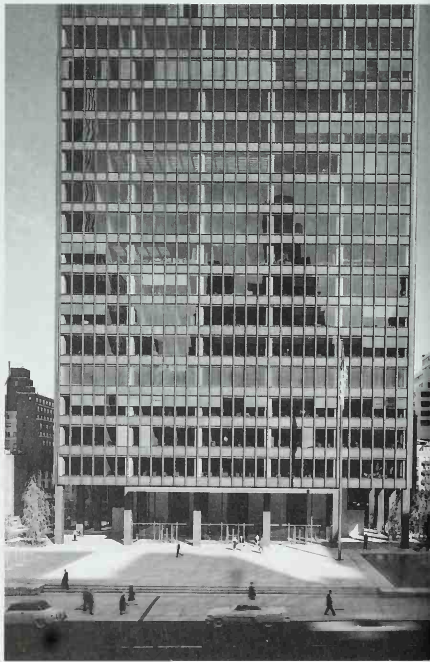
329 Seagram Building; New York, New York. Mies van der Rohe with Philip Johnson and Kahn & Jacobs, 1954–58. Photo: Ezra Stoller, © Esto. The facade is a grid of amber-tinted glass, bronze spandrel panels, and variously profiled bronze mullions whose composition creates subtle effects of depth, shadow, and scale. The regular rhythm of the vertically aligned elements up the facade serves to emphasize the building's tallness rather than to give a truly accurate expression of the underlying steel grid structure. A similar artfulness explains the treatment of the exposed columns at the base, which are concrete-encased in order to satisfy fireproofing requirements, but are then sheathed in bronze to serve as a reminder of their metal core.
