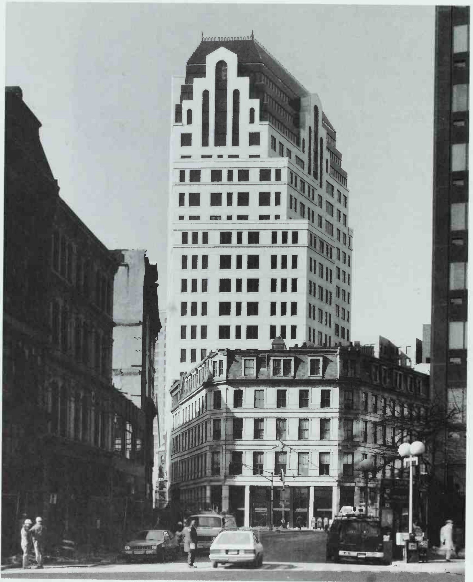
373 99 Summer Street; Boston, Massachusetts. Goody, Clancy & Associates, 1986–87. Photo: © Sam Sweezy. Moldings built up of several pieces of thin granite at the cornice lines and curved metal window surrounds painted to look like granite were used to give the facade a surface depth similar to that of older adjacent buildings.
