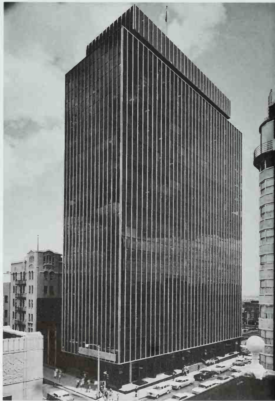
334 First National Bank of Nevada; Reno, Nevada. Langdon & Wilson, 1965. Photo: Julius Shulman. The building's vertical dimension is emphasized by the continuous alignment of the steel mullions, which project forward of the glass panels of the curtain wall.
