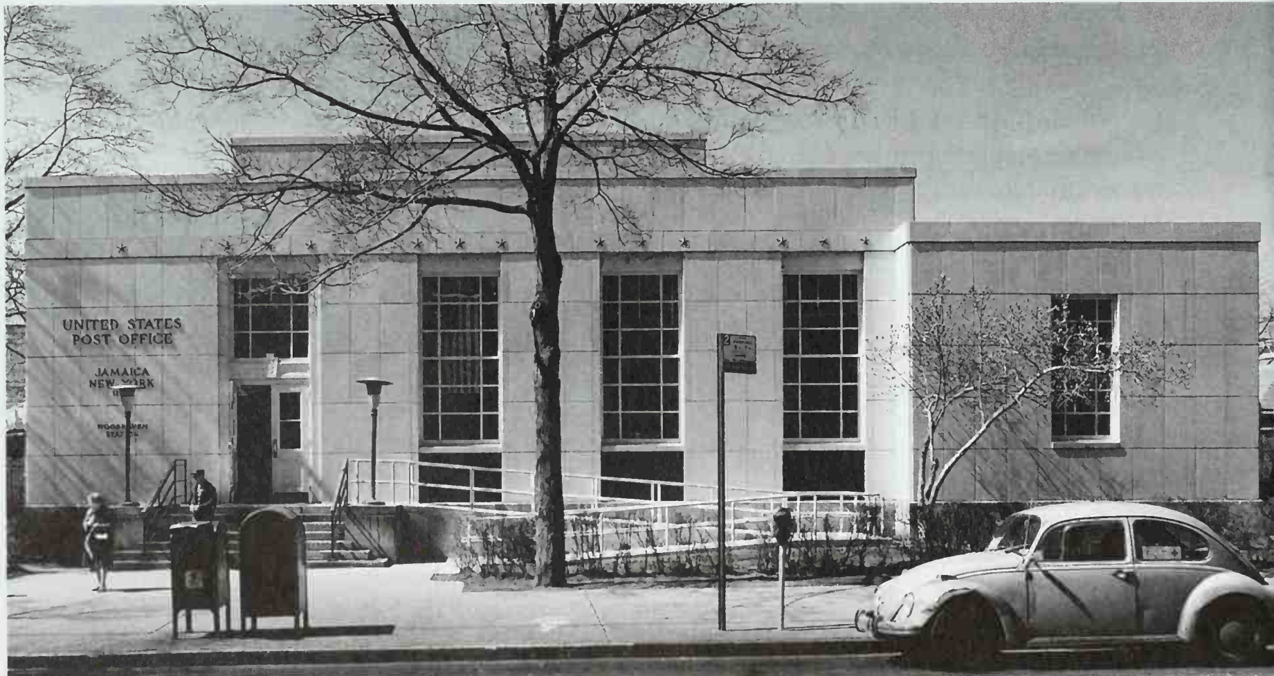
150 United States Post Office, Woodhaven Station; Queens, New York. Louis Simon, Works Progress Administration, 1940. Photo: New York Landmarks Conservancy. Public purpose is announced by emphatic signage and the monumental scale of window and door openings.
