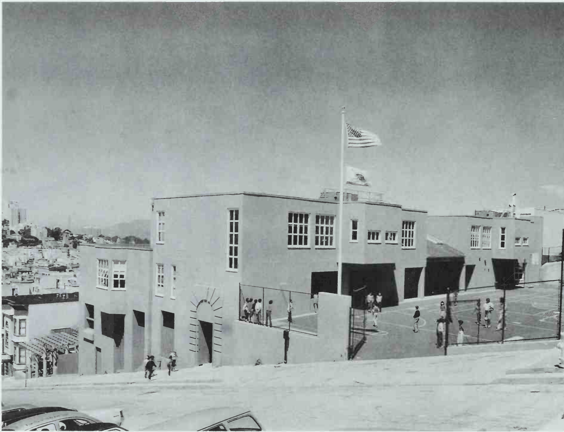
313 Garfield Elementary School; San Francisco, California. Esherick, Homsey, Dodge & Davis, 1980. Photo: © Peter Aaron/Esto. The school's small scale, gentle massing, and informal detailing maintain the character of the neighborhood.
