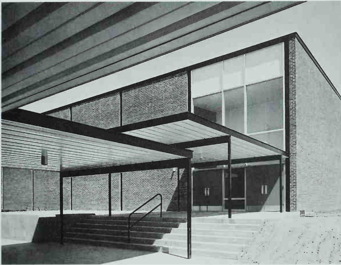
290 James Monroe Junior High School; Tulsa, Oklahoma. Murray Jones Murray, 1957. Photo: Ben Newby. The crisp steel frame, brick curtain wall, and modular window panels express the modernity of the school.
