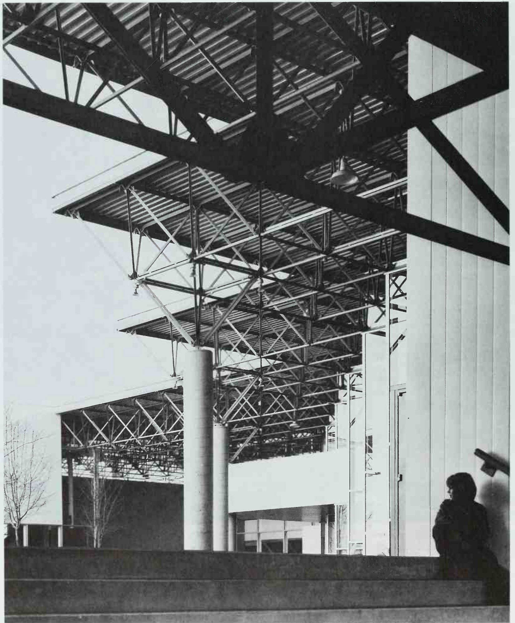
298 Fodrea Community School; Columbus, Indiana. Caudill, Rowlett & Scott, 1973. Photo: Balthazar Korab. A steel space frame resting on concrete columns produces open, unobstructed areas where students group and regroup for different learning activities.
