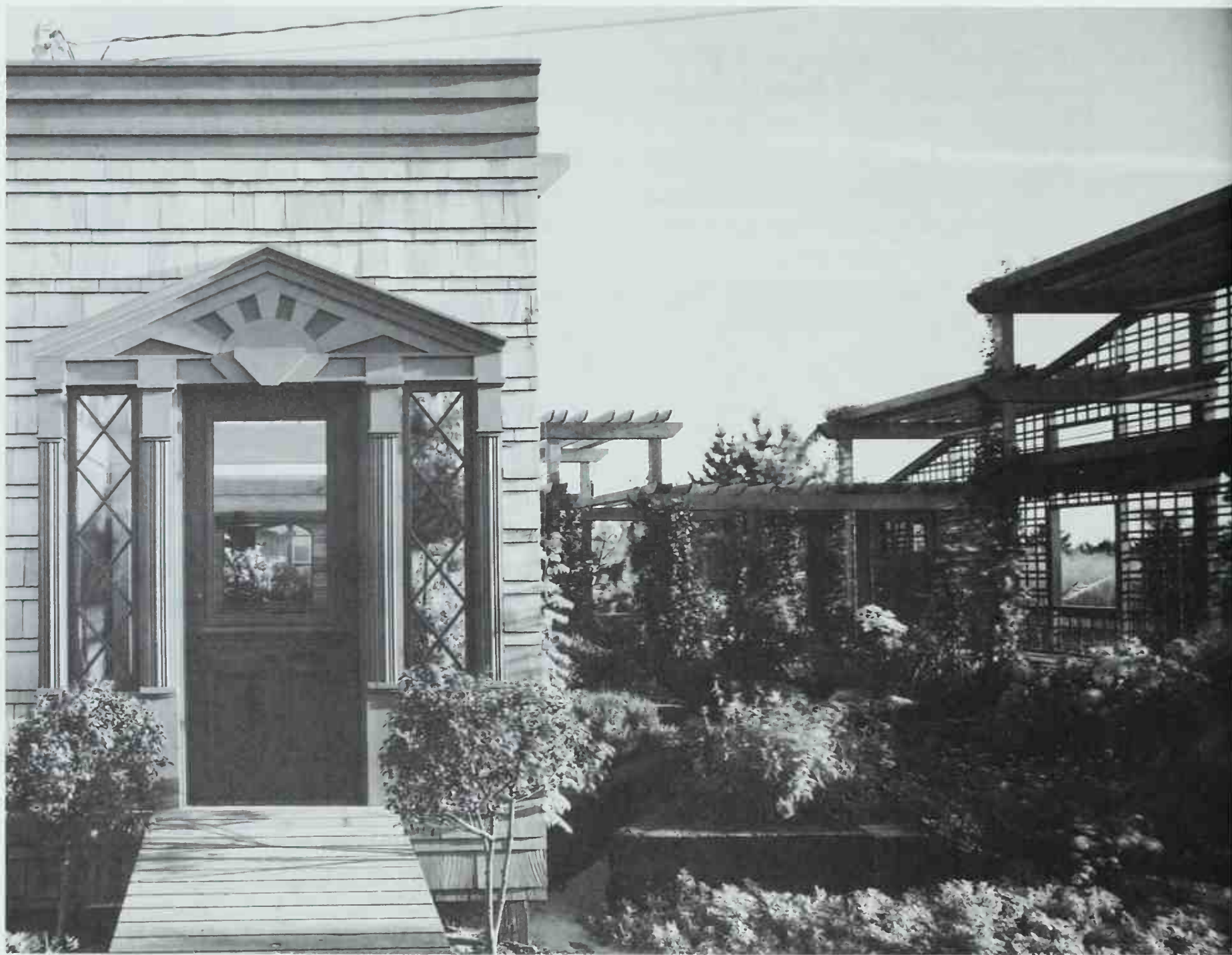
111 Peitsky house; Fire Island, New York. Peter Wilson, 1981–82. Photo: © Peter Aaron/Esto. The real focus of the house is a garden room framed by lattice screens and trellises.
