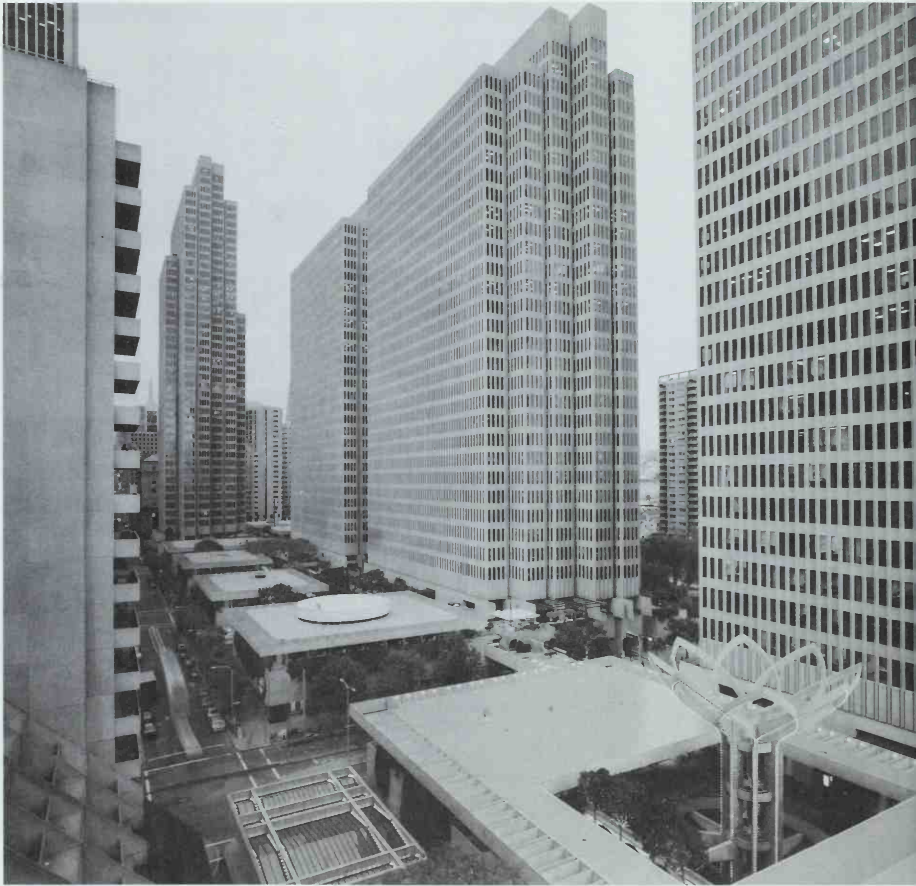
408 Embarcadero Center; San Francisco, California. John Portman & Associates, 1968–81. Photo: © Timothy Hursley. As at New York's pioneering Rockefeller Center, the design ties several shopping levels into the city sidewalks.
