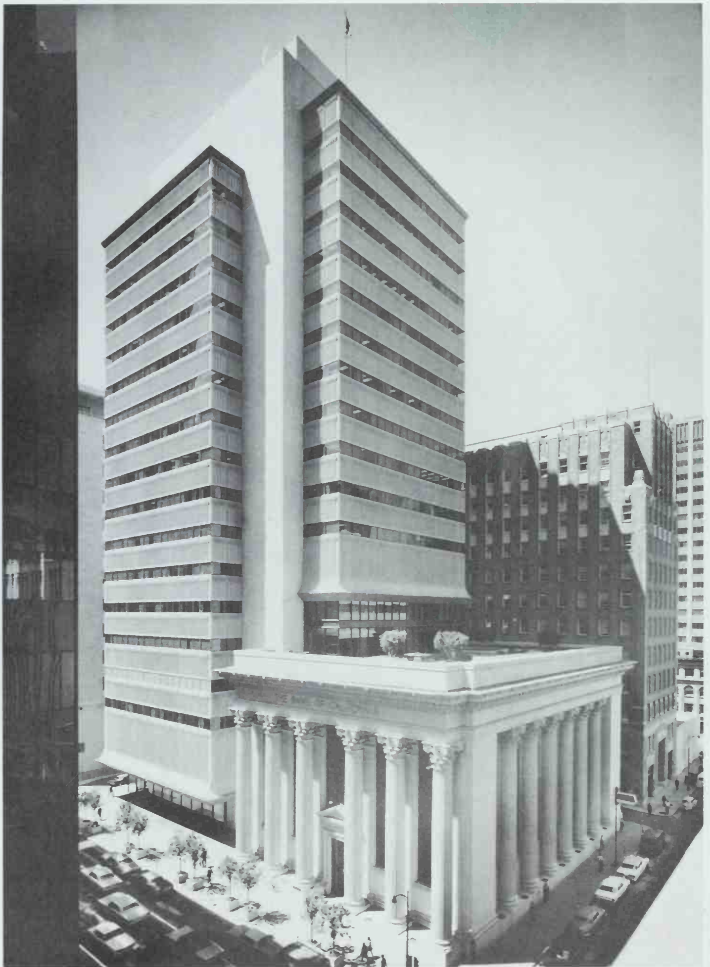
336 Bank of California Headquarters; San Francisco, California. Anshen & Allen, 1979. Photo: © Ted Mahieu. The heaviness of the concrete curtain wall is belied by the lightness and transparency of the glass-enclosed entrance level of the new tower. Cantilevered over the old bank, the new one uses its roof as a terrace.
