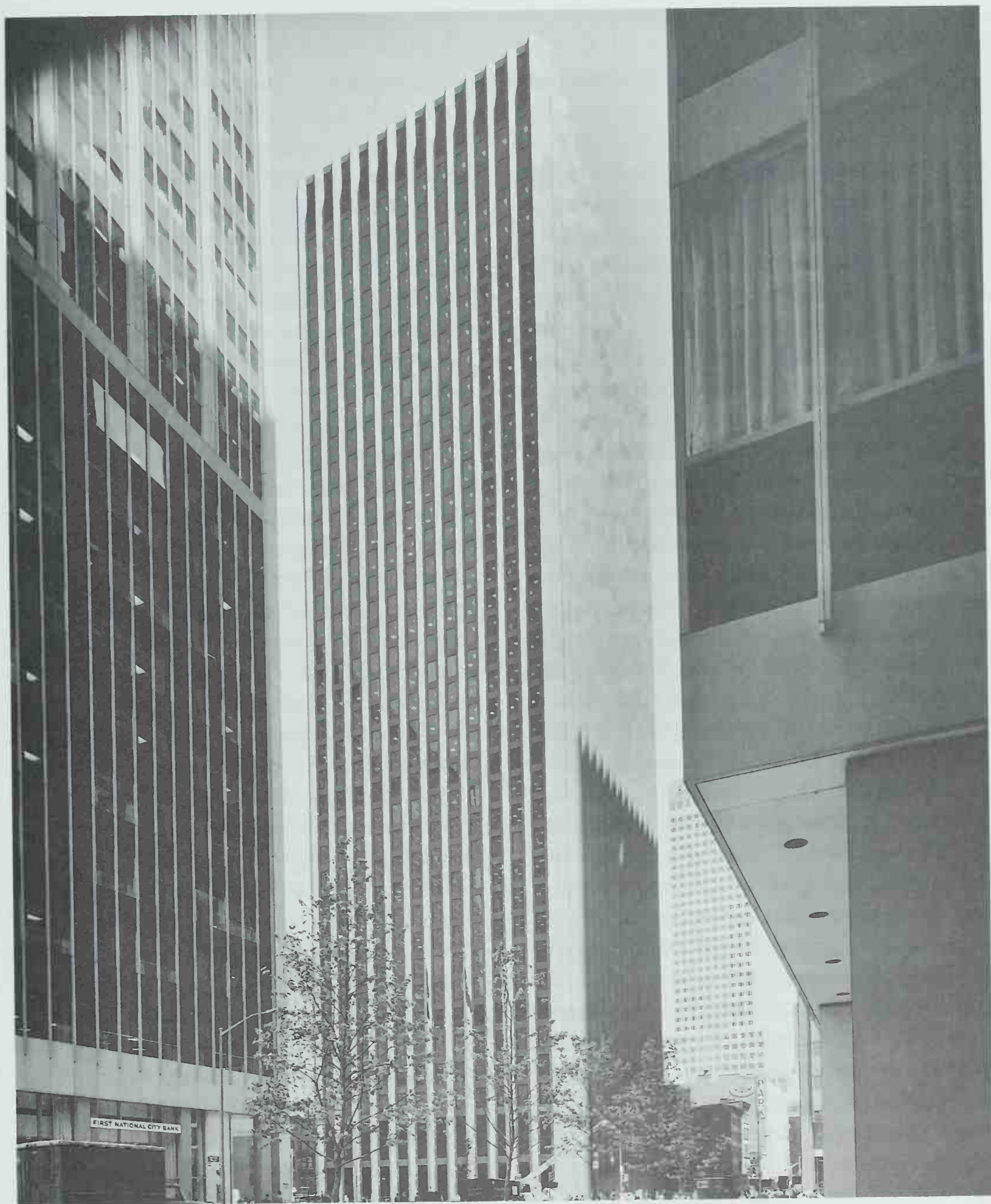
345 CBS Building; New York, New York. Eero Saarinen, 1963–65. Photo: Joseph Molitor. The close spacing and forward projection of the columns produce an effect of weight and mass, although the structure is actually highly efficient in its use of material. The setting of the columns on the diagonal makes the building surface appear solid when it is seen from certain angles.
