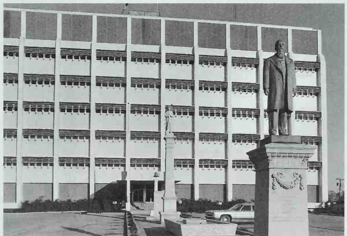
154 St. Mary Parish Court House, Franklin, Louisiana. John Baker and Neild-Somdal Associates, 1950–51. Photo: Geoff Winningham, Seagram County Court House Archive, Library of Congress. The functionalism of the design is apparent in the simply expressed piers and window grilles.
