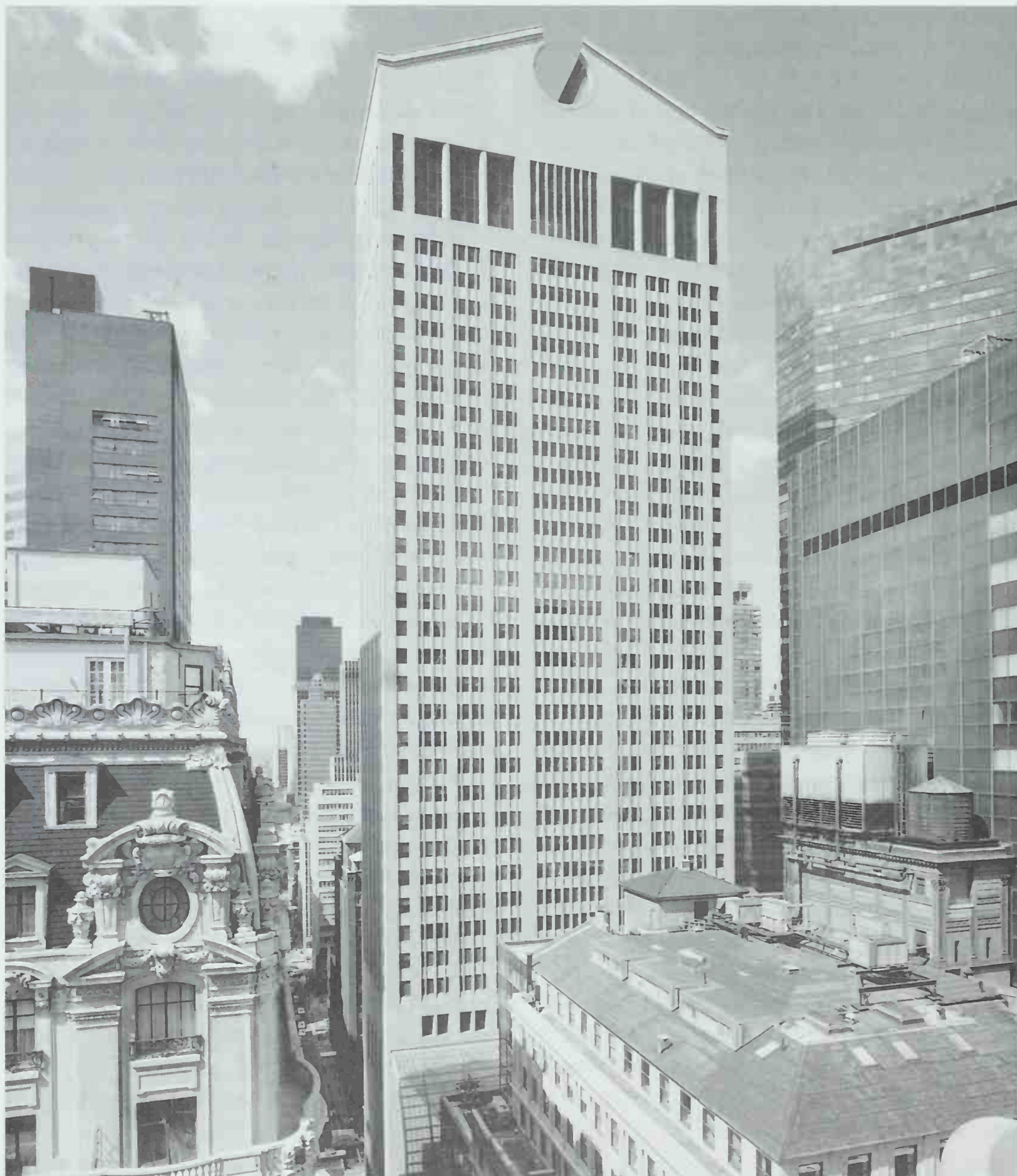
366 AT&T Headquarters (now SONY); New York, New York. Johnson/Burgee Architects, 1978–84. Photo: © Peter Mauss/Esto. A series of tubes are used in combination in order to achieve the desired configuration: two vertical shear tubes in the core on either side of the eight-story lobby space; a cross-braced tube that transfers weight from upper tubes to the stilted columns at the base; a cross-braced tube carrying the weight of the pediment at the top; two partial tubes supporting the narrow end walls. Although it has no structural role, pink granite cladding is heavily detailed to give the appearance that it is weight bearing.
