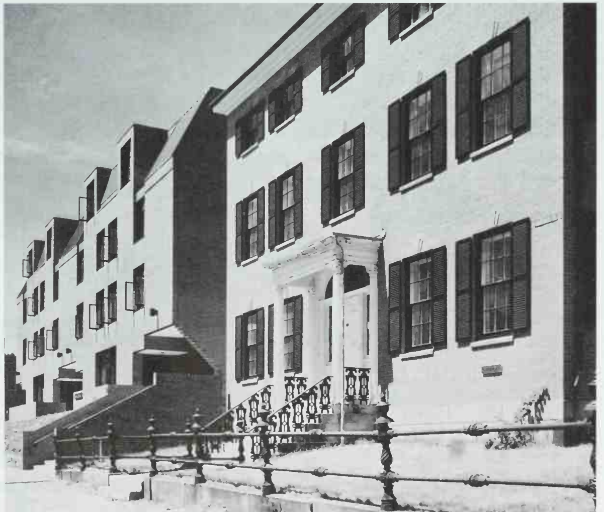
141 Park Danforth; Portland, Maine. Stecker LaBou Arneill, 1970. Photo: Bill Maris. Designed for compatibility, the modern addition echoes the historic mansion in its relationship to the street, materials, fenestration, and eaves line.
