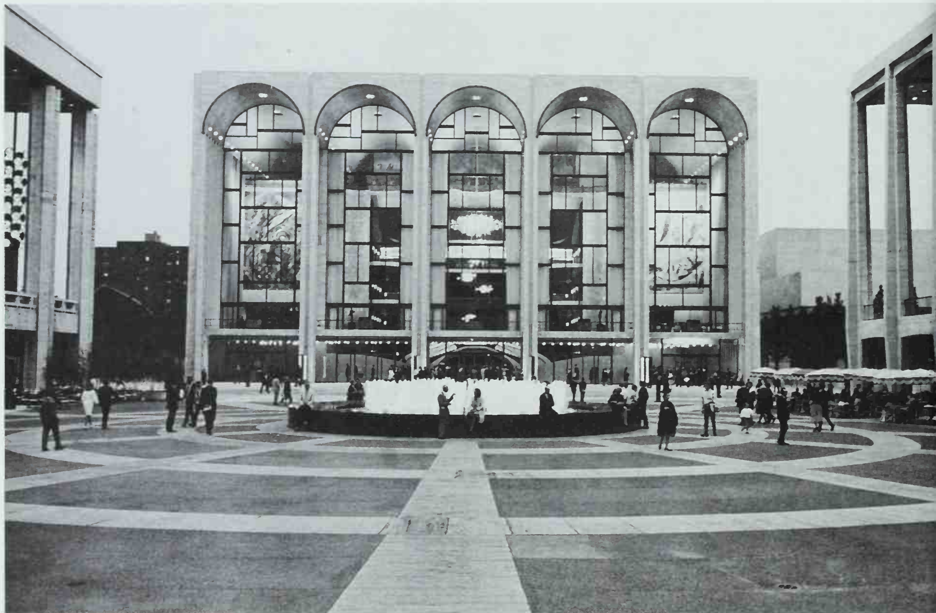
159 Lincoln Center for the Performing Arts; New York, New York. Avery Fisher Hall (right), Max Abramovitz, 1962; Metropolitan Opera House (center), Wallace Harrison, 1966; New York State Theater (left), Philip Johnson, 1964. Photo: © Katrina Thomas. The uniform roof and entrance height, common use of travertine facing, repeating colonnade, and formal plaza dramatize classicizing ambitions.
