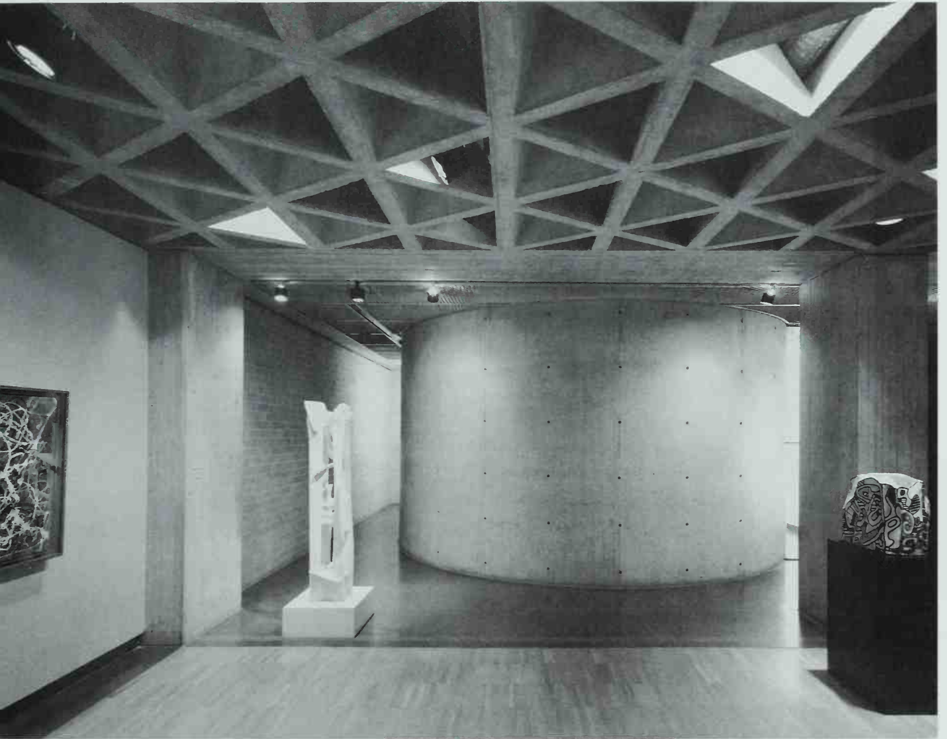
200 Yale Art Gallery; New Haven, Connecticut. Louis I. Kahn, 1951–53. Photo: © Grant Mudford. Architecture exerts its presence in the powerful form of the round stairwell and the deep trusses that integrate structure with lighting and ventilation.
