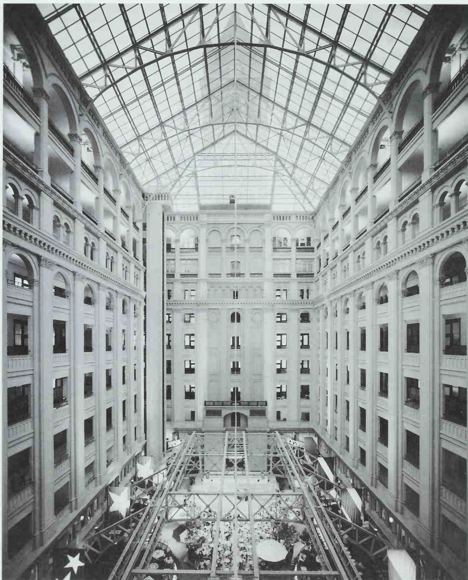
194 Old Post Office; Washington, D.C. Arthur Cotton Moore Associates, 1983. Photo: Hoachlander Photography Associates. The adaptive use of the historic post office required a cut into the main-floor level to create a three-level atrium for a shopping and dining mall.
