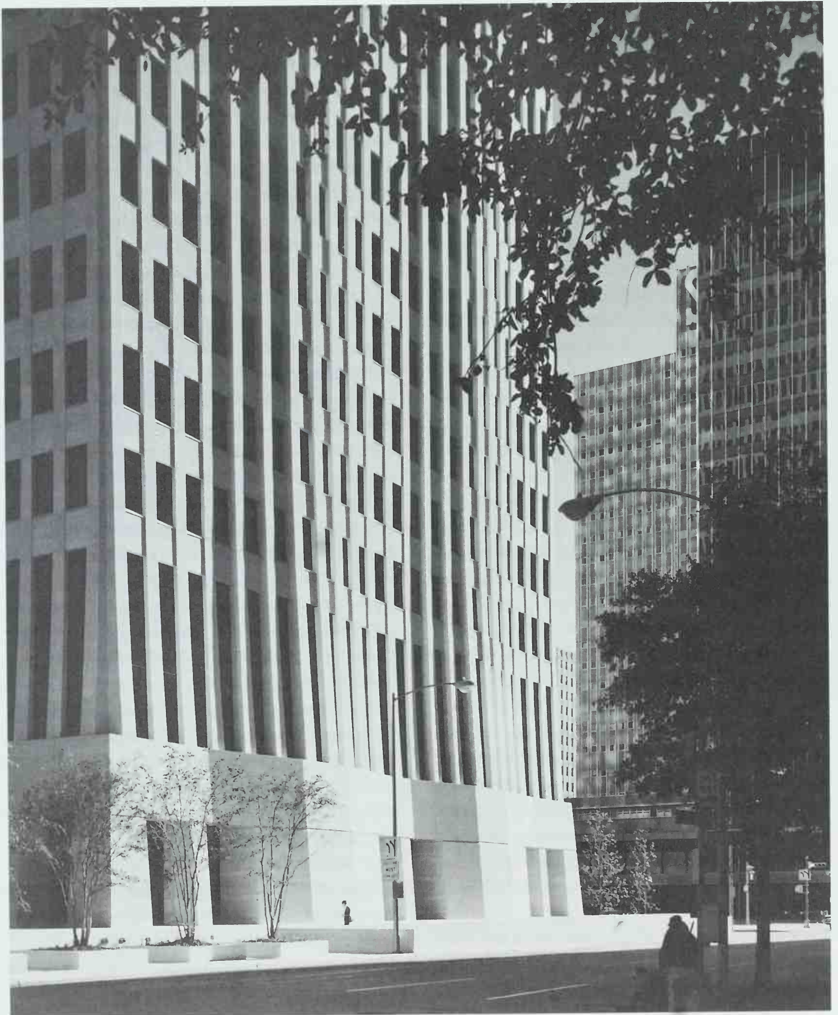
346 One Shell Plaza; Houston, Texas. Skidmore, Owings & Merrill, 1968–71. Photo: Ezra Stoller, © Esto. Projecting out of the walls, rather than hidden within, thickened structural members eloquently portray the support needed at certain points where the interior tube does not provide it.
