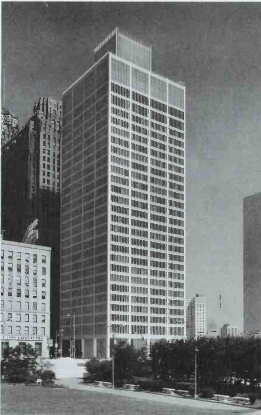
333 Michigan Consolidated Gas Company; Detroit, Michigan. Minoru Yamasaki with Smith, Hinchman & Grylls, 1961. Photo: Balthazar Korab. The wall's division into bays corresponds to the module of the skeleton. Although it rises from a bulky square plan, the tower achieves a striking vertical effect with slender window openings and the tracery effect of narrowly spaced steel mullions.
