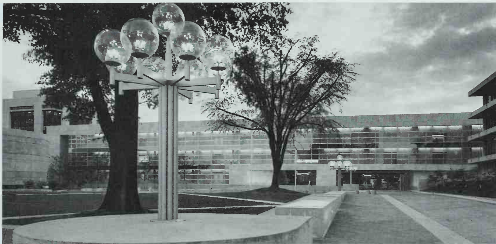
180 Mecklenberg County Courthouse; Mecklenberg, North Carolina. Wolf Associates, 1977. Photo: © David Franzen/ Esto . Defining a new public plaza, the glass-fronted courthouse also serves as a circulation spine that links a parking garage and government office building.
