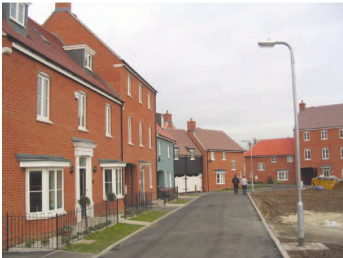
Plate 4.2 The BAe site development approaching completion. Architecture is by Reeves Bailey. Note the provision of small front gardens. Source: Chelmsford Borough Council.
