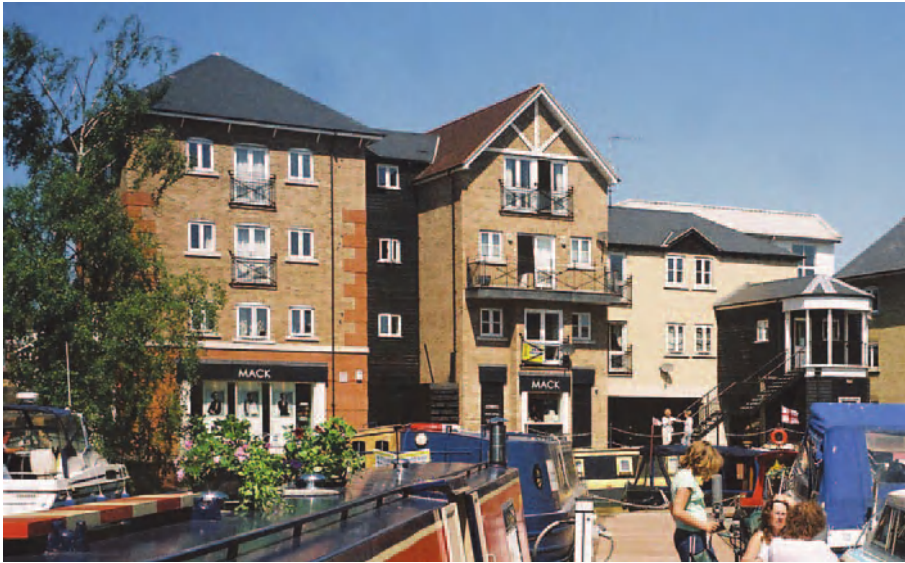
Plate 7.2 Coate's Quay – Phase 2. Source: Roy Chandler.
