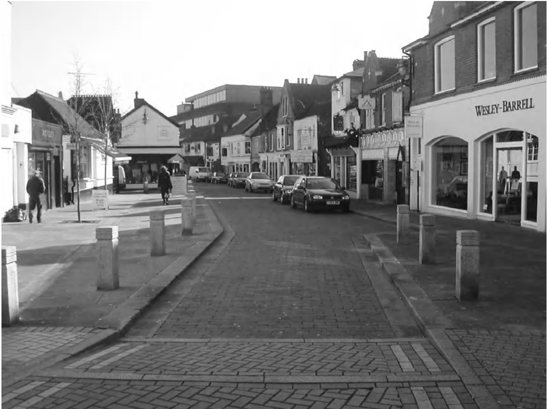
Figure 6.5 The section of Baddow Road within the town centre repaved with the use of York stone to increase the space for pedestrians while retaining vehicle access. Source: Chelmsford Borough Council.
