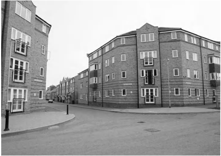
Figure 5.13 Flats used to turn corners at the centre of the Writtle Road development. Source: Chelmsford Borough Council.
