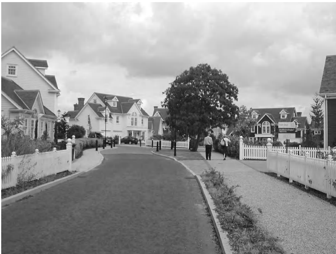
Figure 5.5 The second stage of the Beaulieu Park development by Copthorne. Source: Chelmsford Borough Council.
