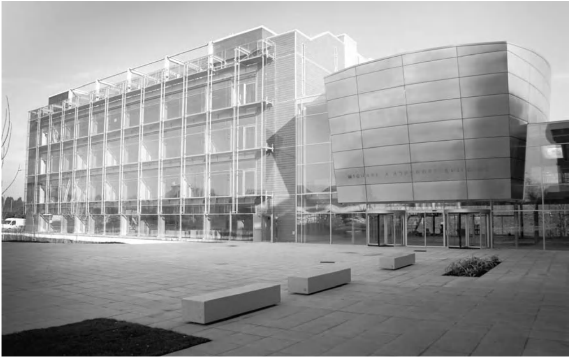
Figure 6.30 The new university campus – the Ashcroft Building, by Wilkinson Eyre, containing the business school. Source: Anglia Ruskin University.
