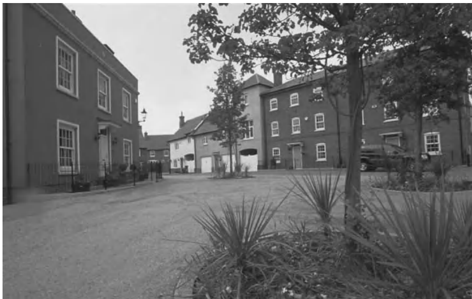
Figure 5.7 The central square and visitors parking court at Bishops Mead. Note the provision of small front gardens. Source: Chelmsford Borough Council.
