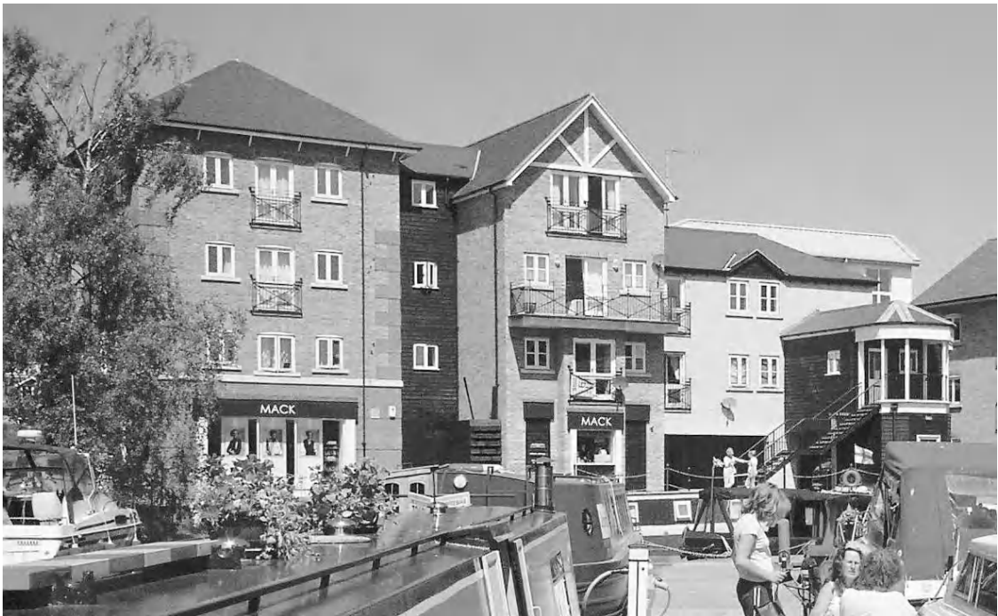
Figure 7.6 Coate's Quay – Phase 2. See also Plate 7.2. Source: Roy Chandler.
