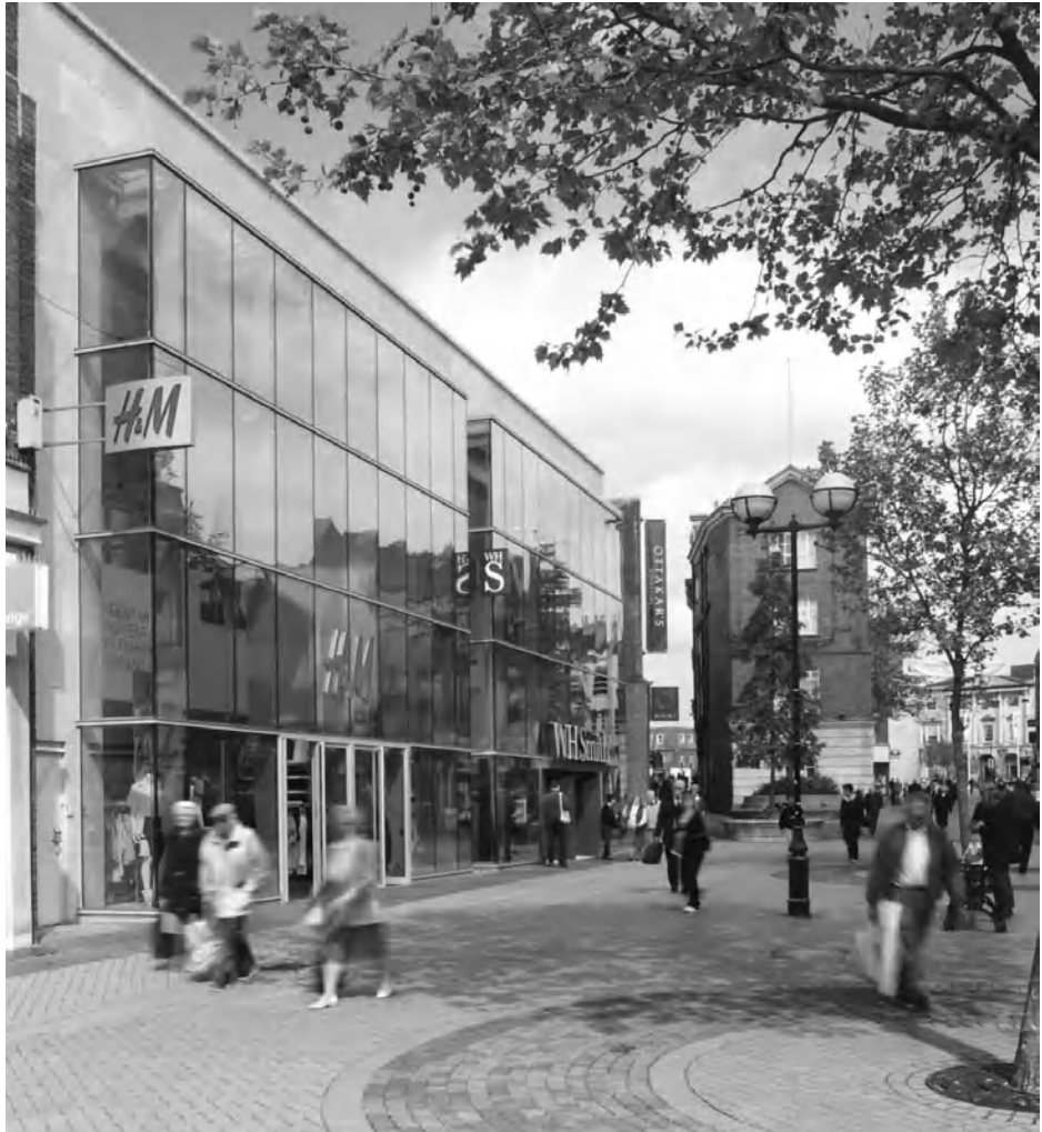
Figure 6.7 Replacement of High Street shops in a contemporary style. Source: Anglia Ruskin University.
