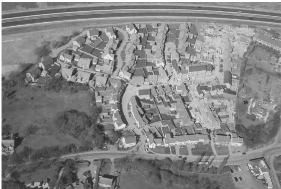
Figure 5.27 An aerial view of phase 1 of the Great Leighs development under construction. See also Plate 5.5. Source: Peter Rodgers.
