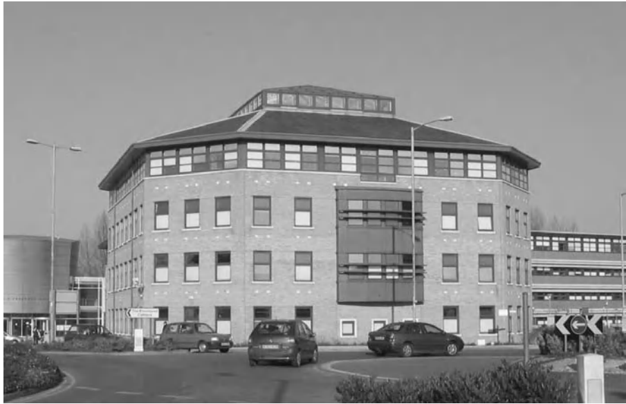
Figure 6.26 The new University campus – the first major new low-energy building, the Queen’s Building containing the university library. Source: Anglia Ruskin University.
