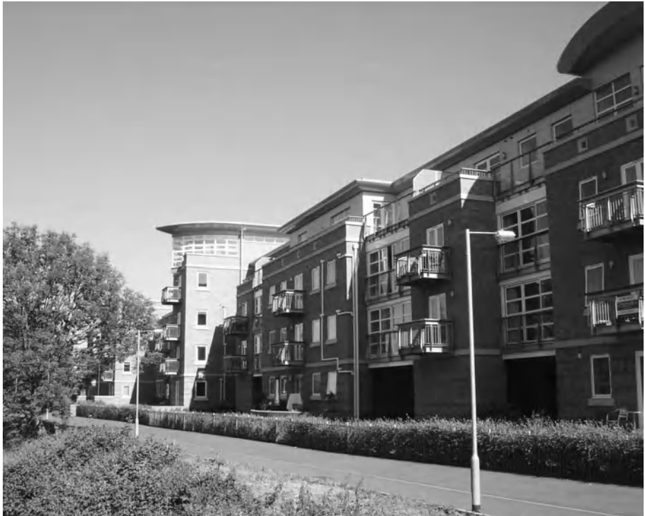
Figure 7.15 The Callow Court flats by Barratt overlooking the Central Park. Source: Tony Hall.
