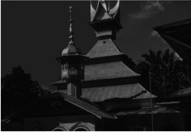
Fig. 3.2 A mosque in Sumatra Barat with a syncretic roof form depicting inflectional images from Minangkabau, Java and the Middle East
