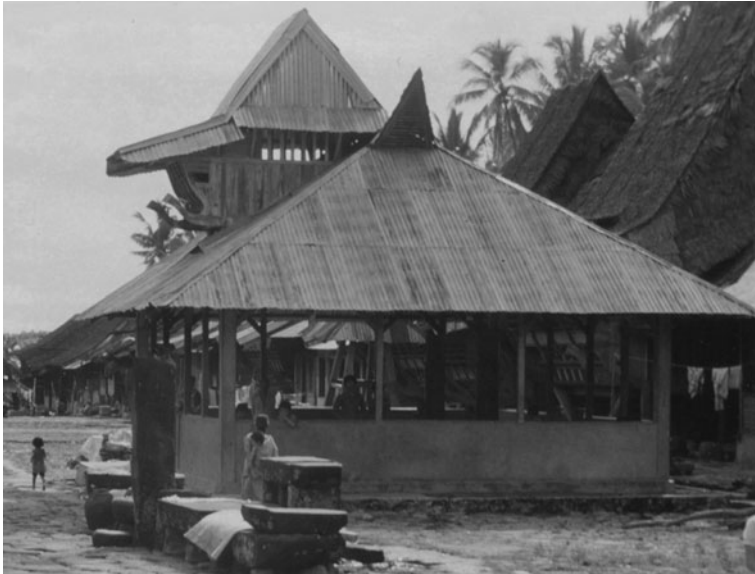
Fig. 8.11 Bale in the village of Orahili built with galvanized zinc roof-covering material and pyramidal roof
