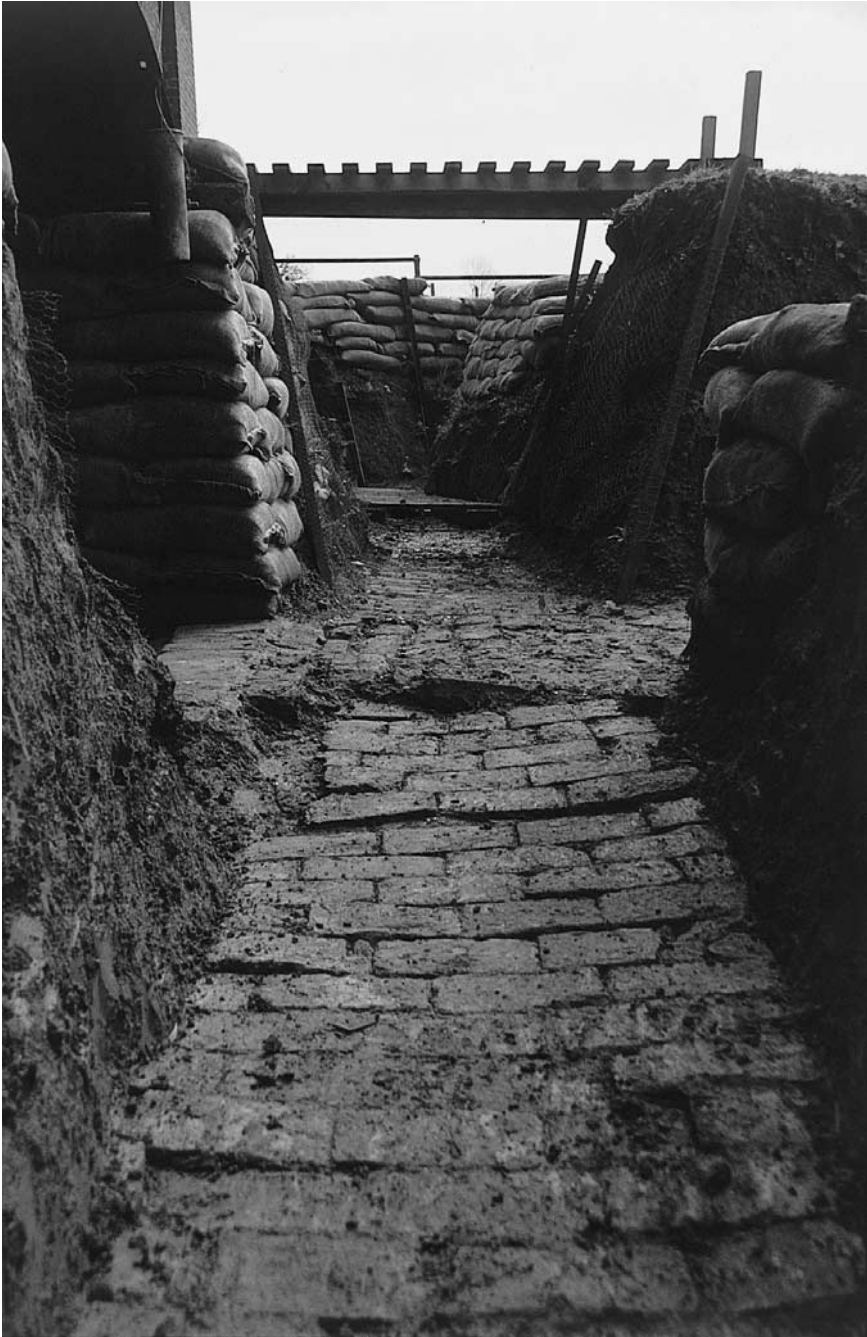
Figure 13.2 A trench floor, as consolidated, looking east, Auchonvillers. The chicken wire and angle iron were replaced from excavated evidence (© author).
