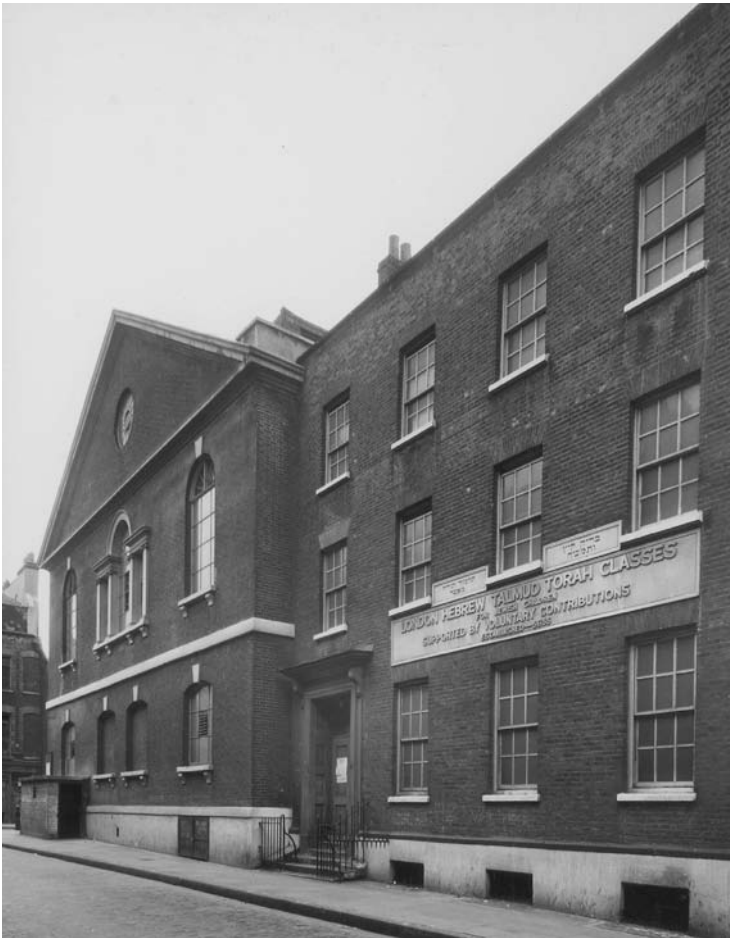
The 'Neuve Eglise' on Brick Lane, built in 1743 by Huguenot immigrants, later remodelled as a Methodist chapel, in the nineteenth century transformed into a synagogue, and finally in the 1970s converted into a mosque for the Bangladeshi community (photograph, 1953).
