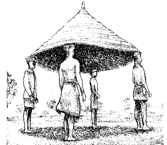
MOVING THE ROOF OF A HOUSE IN GUINEA
