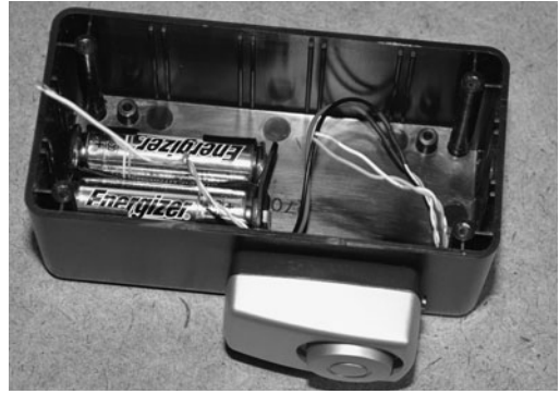
Figure 20-22 Mounting the alarm siren and the battery pack to the enclosure.
