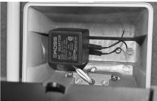
Figure 6-9 The AC-to-DC power pack was installed in the light enclosure.
