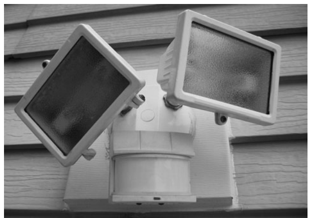
Figure 24-1 Any common outdoor motion-sensor light can be used for this project.
