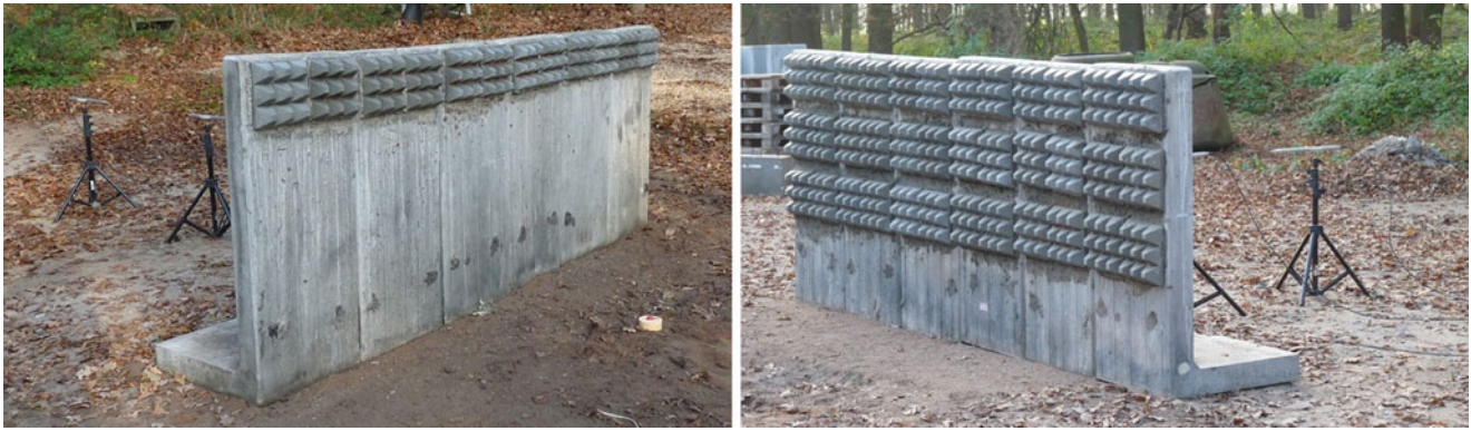
Fig. 3 Barriers equipped with concrete sheeting
