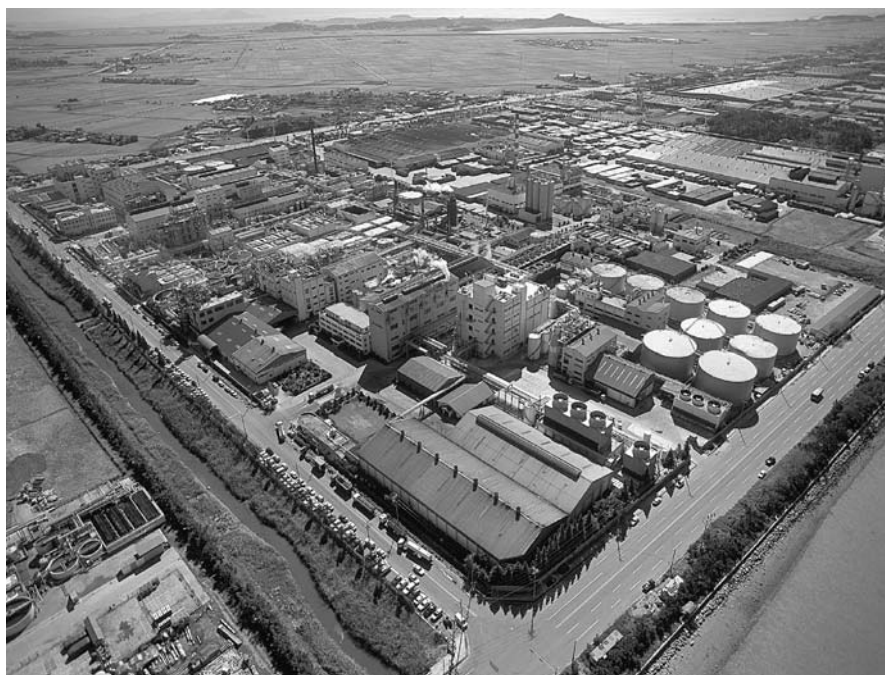
Fig. 9 Lysine production plant of the BASF AG located in Gunsan, South Korea with an annual capacity of about 100 000 tons. Copyright BASF AG—The chemical company (2003). Reproduced with permission
