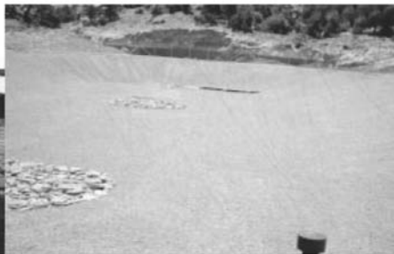
Erosion Pad in Shallow Pond with Surface Aerators
