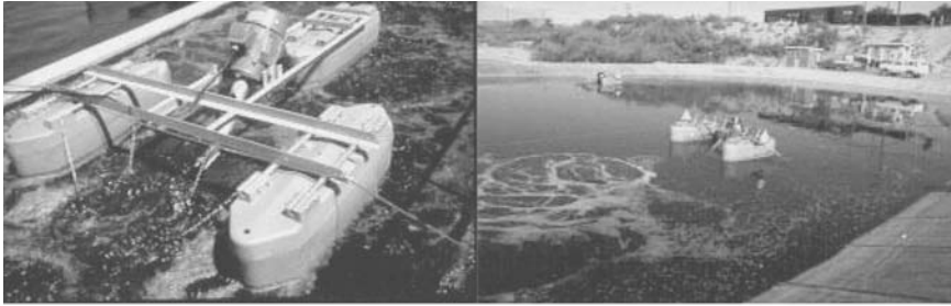
Aspirating Aerator Up Close and Mixing Effects of Aerator
