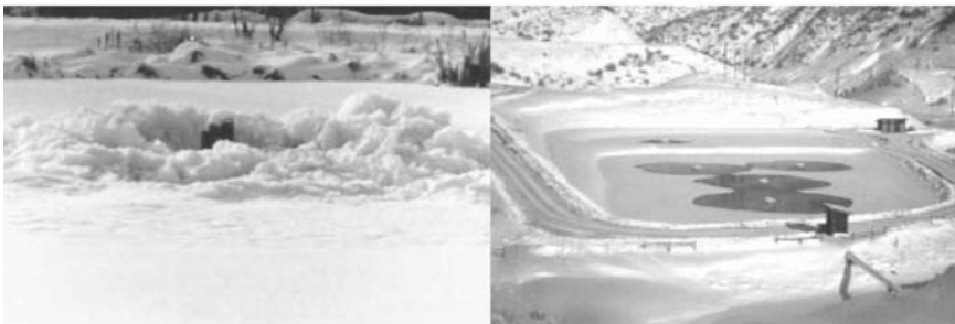
Floating Aerators During Winter Operation
