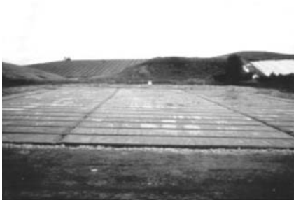
Covered Aerated Pond
