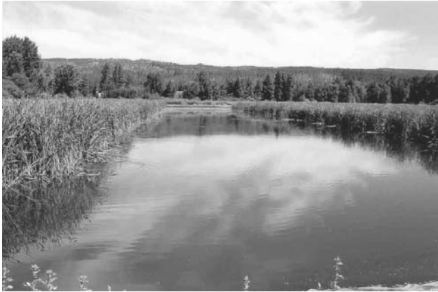
FIGURE 6.4 Free water surface (FWS) wetland at Cle Elum showing bulrush and open water.
