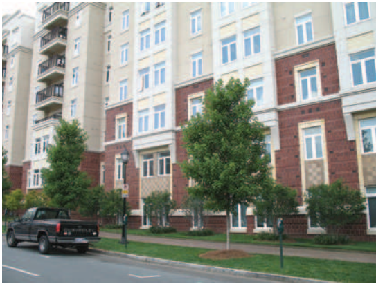
Figure 6.4 City center housing, Charlotte, NC, 2005. At a large scale, this urban housing block demonstrates decent urban design in terms of placement and massing, but the architecture fails through its lack of attention to street-level detail. The omission of porches, stoops or visible entrances diminishes the pedestrian environment, and the low placement of windows to private rooms severely compromises the visual privacy of those spaces. The useless strip of grass and a few bushes against the building are a feeble attempt to provide a privacy screen, but they simply create an unwanted suburban feel completely at odds with the building's context.
