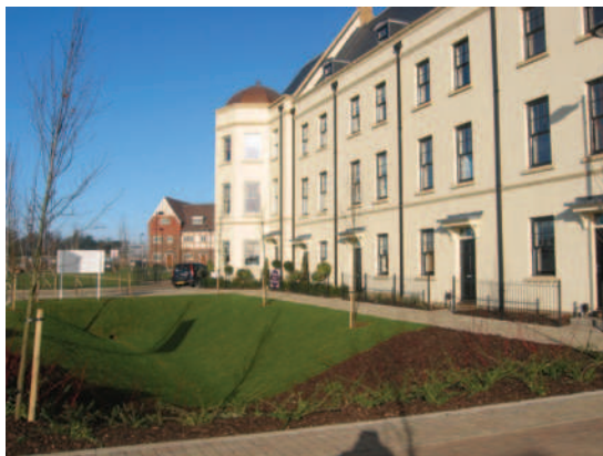
Figure 5.34 Sustainable Urban Drainage System (SUDS) at Upton, Northampton, UK. Landscaping devices to retain water for on-site filtration are incorporated into the urban design detailing for public spaces. See also Figure 5.11.
