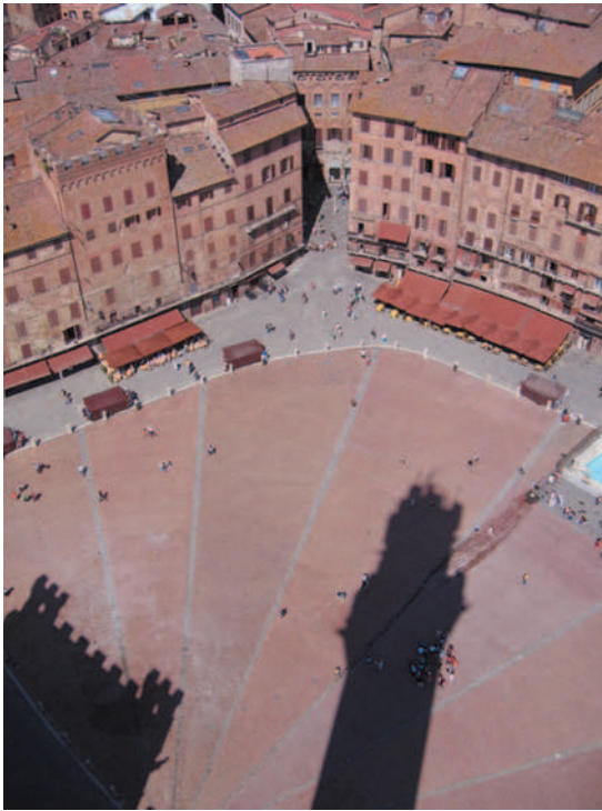
Figure 5.2 Piazza del Campo , Siena, Italy, 1262 onwards. The design of the palazze surrounding the main public square demonstrates the unifying themes imposed by medieval design codes. (Photo by Adrian Walters)
