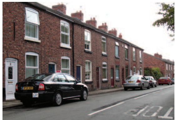
Figure 4.8 Refurbished terrace houses, Black Road, Macclesfield, UK. The end of this row of houses is marked by a plaque commemorating the successful efforts of architect Rod Hackney in 1974 to forestall demolition and obtain local government grants for the conversion and renovation of older housing.
