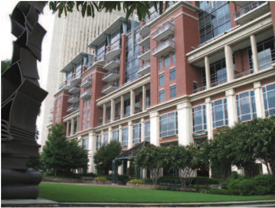
Figure 2.2 Uptown Housing on the Green, Charlotte, NC; FMK Architects. High-density urban living is now commonplace in the center of mid-size American cities such as Charlotte. This good example is constructed over an underground parking garage topped by a landscaped park, providing the city with good public space replete with public art.
