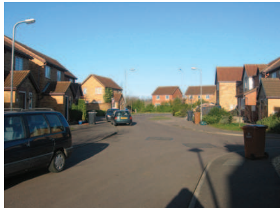
Figure I.1 Mediocre contemporary British suburban development. This housing estate adjacent to the new Upton development in Northampton, UK, illustrates sloppy design qualities typical of much British suburban housing. No attention is paid to creating defined urban spaces or good detailing of the public realm. Compare to Figures 3.5, 5.11 and 5.34.
