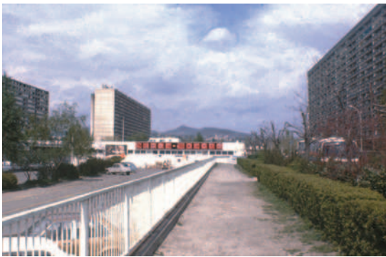
Figure 6.13 Housing at Lyon, France, 1977. Modernist urban design swept away traditional multi-purpose spaces of streets and squares, replacing them with single function walkways and parking areas amidst widely spaced, large buildings.
