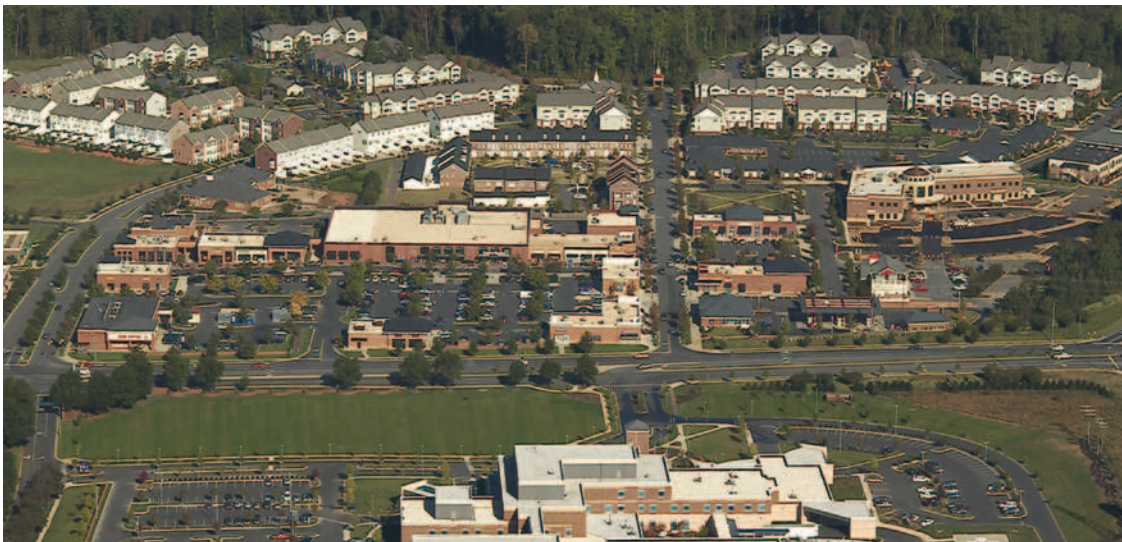
Figure 8.7 Rosedale development and Presbyterian hospital, Huntersville, NC. In the late 1990s, the author helped resolve the plans of two competing developers on the Rosedale site. The end result was a cohesive plan for shops, offices and housing organized around a connected street pattern instead of separate parking lots. Less ambitious than the mixed-use Birkdale Village (see Figure 8.1), Rosedale has become a model for 'multi-use developments' where uses are horizontally adjacent but not mixed vertically within buildings. Like Birkdale, the urban form of this development was created through the town's form-based zoning regulations. (Photograph by Aerial Dimensions; reproduced courtesy of Town of Huntersville)
