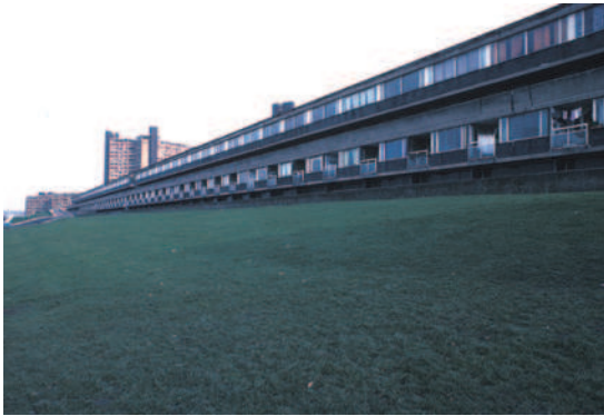
Figure I.2 Housing at Park Hill, Sheffield, UK. These gargantuan exercises in brutalist formalism from the 1960s were highly regarded by architects but despised by most residents. The concrete housing blocks have been listed as Grade II historic buildings and are due for a major refurbishment by the development company Urban Splash whereby 1000 original flats will be converted into 867 new apartments, and the public spaces completely revamped and reconnected to the city center.
