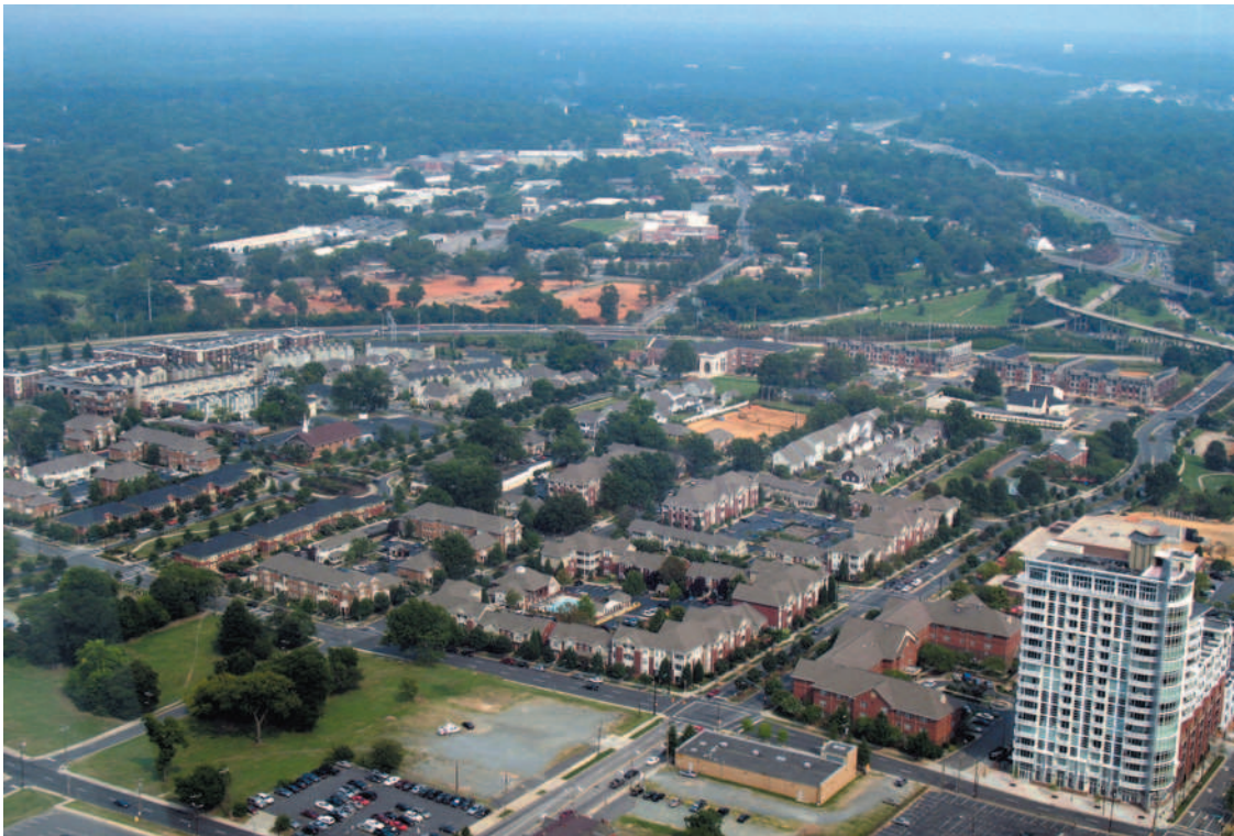
Figure 6.3 First Ward Place and Garden District, Charlotte, NC, 2006. While other sites await the arrival of light rail transit and future development, the HOPE VI project (center foreground) has stimulated extensive private development on adjacent blocks in a part of town once considered a ‘no-go area’ due to gang violence.
