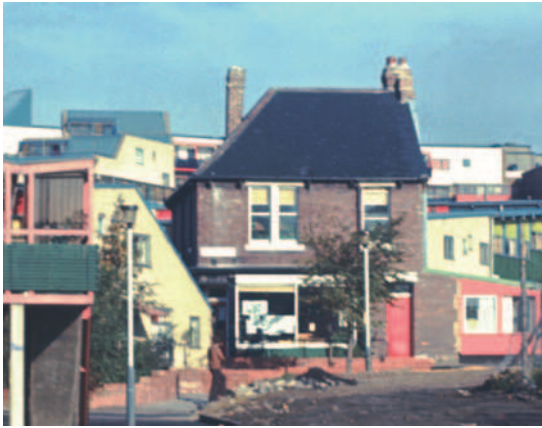
Figure 4.10 Architects' office, Byker, Newcastle-upon-Tyne, UK, 1971. This converted funeral parlor was the setting for much community activity during the lengthy redevelopment process (See Table 4.1).
