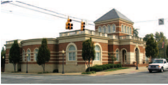
Figure 8.31 Huntersville town hall, 1997; David A. Creech, AIA, while with TBA2 architects. The town hall and adjacent police department share a neo-classical style in an attempt to bring a sense of civic presence to the faded downtown.
