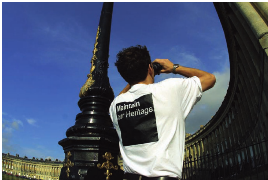
Figure 16.1 Maintain our Heritage undertook a pilot maintenance inspection service in the Bath area. High-level areas were accessed in most cases but remote inspection with binoculars was also helpful.
