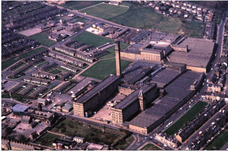
Figure 6.7 Lister's Manningham Mills, Bradford, Yorkshire.
