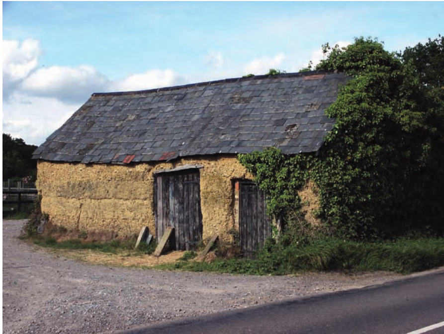
Figure 5.5 An earth-walled stable/cow house typical of a New Forest commoner (Bob Edwards). The farm buildings of commoners in heathland areas offer little opportunity for reuse and so are highly vulnerable, but there is little information available. Most of these buildings are of relatively poor quality and are rarely listed. The mapping of farmsteads has highlighted the need to research this building type.
