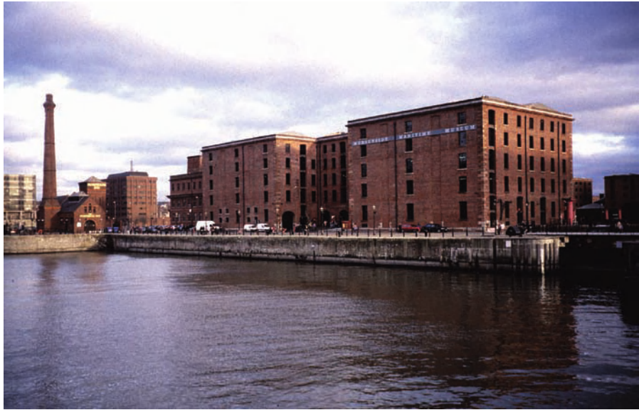
Figure 6.4 Jesse Hartley's Albert Dock, Liverpool, constructed 1846–8.
