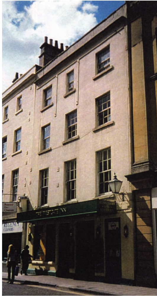
Figure 13.1 The plain street elevation of 38 Westgate Street. Everything on this 'Georgian' facade except the masonry dates from 1969. Nonetheless, study showed a building with a complex building history.
