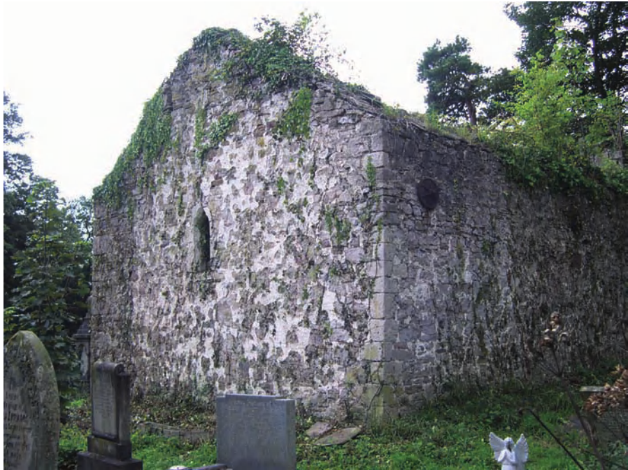
Figure 13.3 The chapel at Tal y Garn from the north-east. The seventeenth-century masonry is clearly recognisable as the darker stone on the left corner and the upper right corner. The tiny window and the wall around it are thirteenth or fourteenth century.
