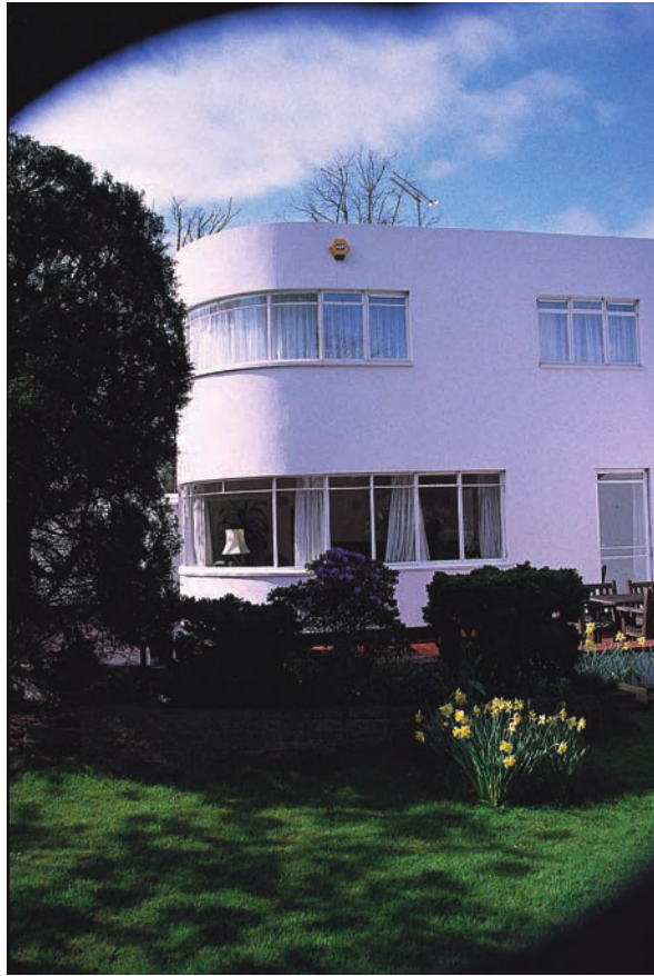
Figure 8.2 'Sunsan' after restoration.
