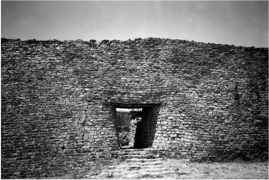
Fig. 11.1 The ruins of Great Zimbabwe consist of massive structures surrounded by un-mortared stone walls, often 30 feet tall. (Photo: Lance Larkin)
