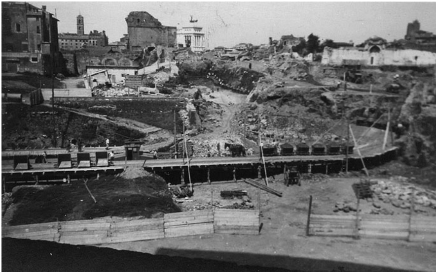
Fig. 9.2 Removal of the Velia Hill for the construction of via dell’Impero 1932 (Archivio Storico Istituto Luce)
