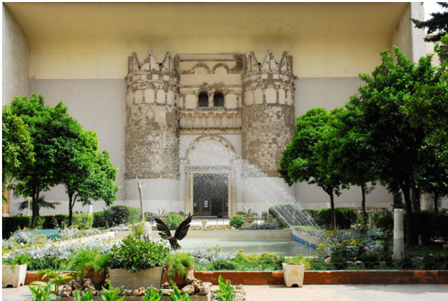
Fig. 8.3 Front entrance of the National Museum of Damascus with the façade of the Qasr al-Hayr al Gharbi. (Photo: Kari Zabler)
