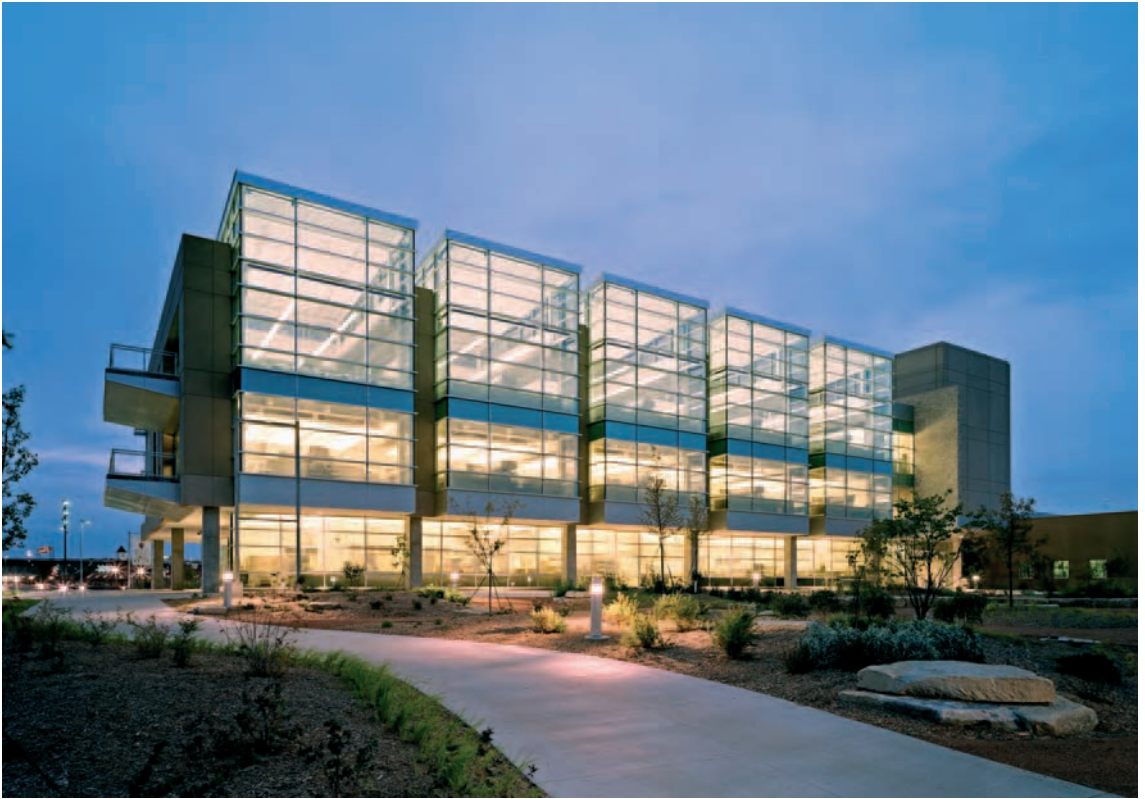
▲ 8.1 Developed under the GSA Design Excellence program, the National Park Service's Carl T. Curtis Midwest Regional Headquarters Building was designed by Leo A Daly to LEED-NC Gold-certification level. Photography by Tom Kessler. Courtesy of Leo A Daly.
