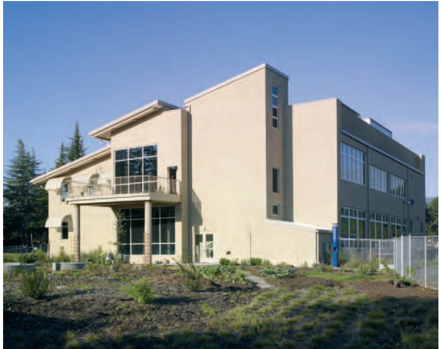
▲ 13.2 Kirsch Center for Environmental Studies, designed by VBN Architects in association with Van der Ryn Architects, is a virtual laboratory for DeAnza College's environmental curriculum. Its LEED Platinum features include natural ventilation, extensive daylighting and native landscaping.
