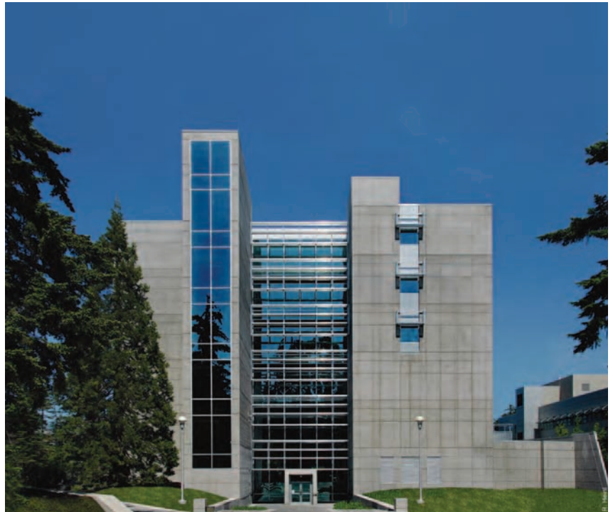
► 5.5 The ECS Building on the University of Victoria campus operates at 51 percent below Canada's National Energy Code. Courtesy of Busby Perkins+Will.
