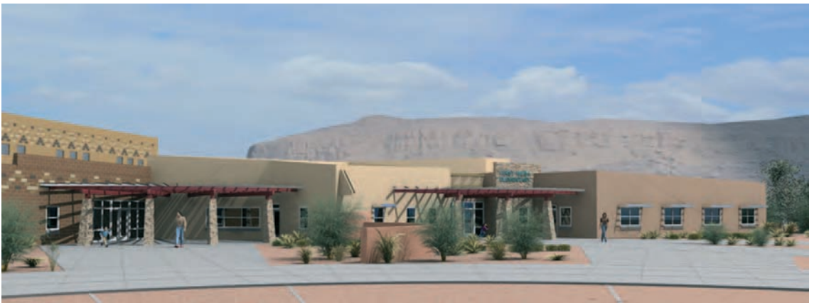
▲ 5.4 Replacing a 50-year-old school, First Mesa Elementary serves 220 children from the Hopi Tribe in Polacca. Designed by Dryon Murphy Architects, a Native American-owned firm, the school is LEED-NC certified. Courtesy of Dyron Murphy Architects, PC.
