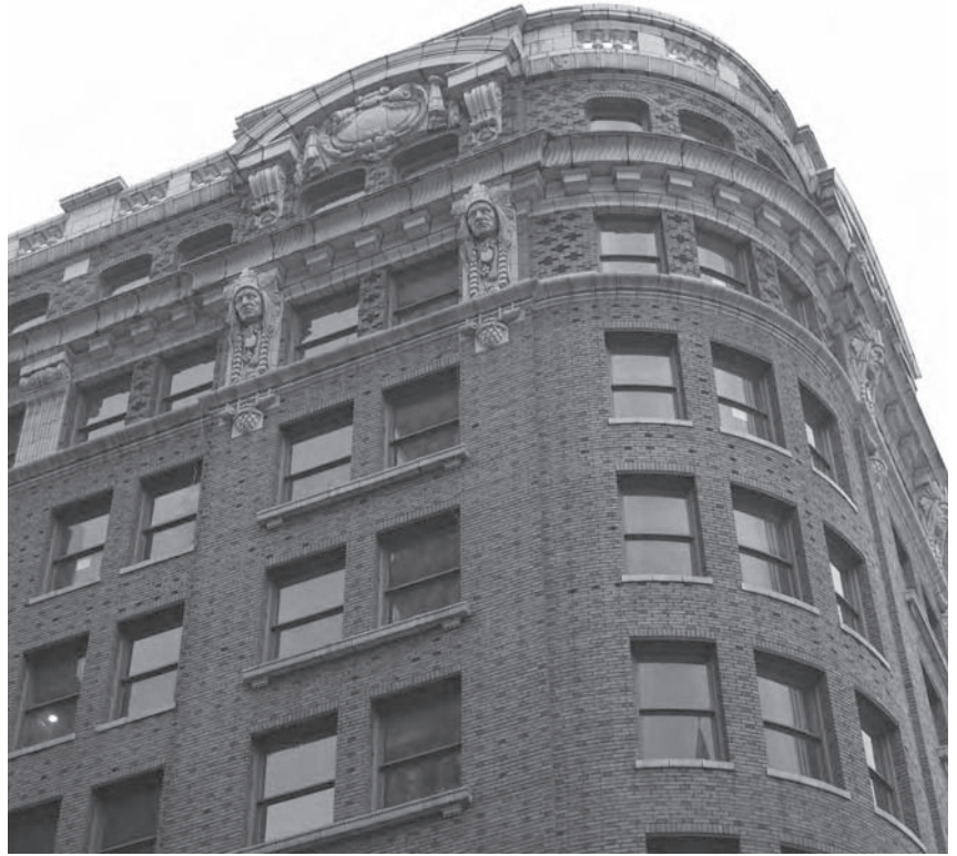
► 5.9 Unico's Cobb Building in Seattle, built in 1910, demonstrates that sustainable features can be incorporated in a historic renovation project. The building is aiming for LEED-NC certification. Photography by Young Lee Courtesy of Unico.
