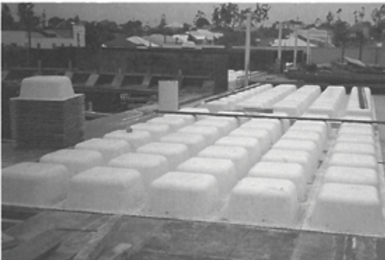
GRP Waffle Forms on Flat Soffit Form
