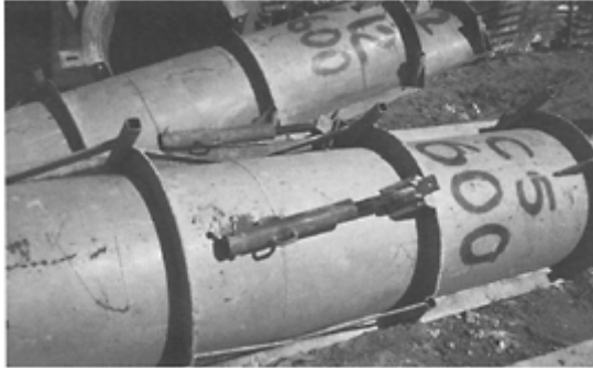
Steel Column Formwork with Bracing Attached.
