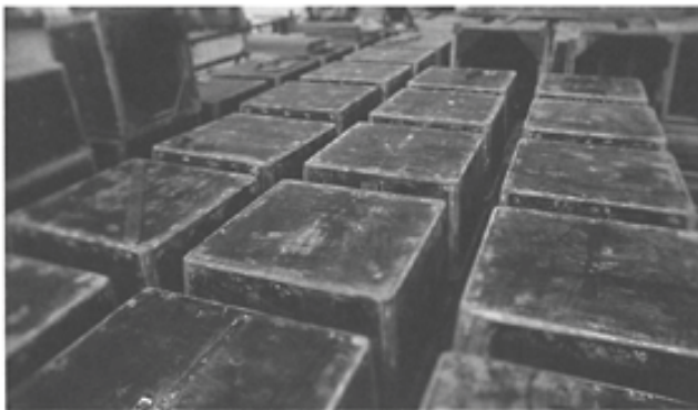
Timber and Plywood Waffle Forms
