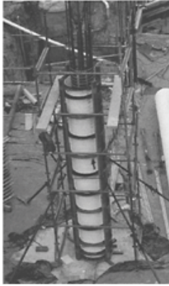
Proprietary Plastic Column Form
