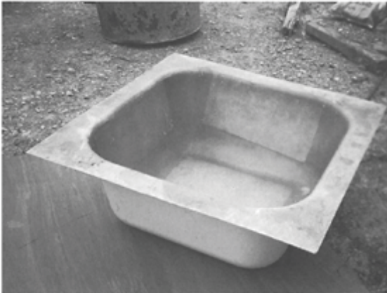
The Underside of a GRP Waffle Form
