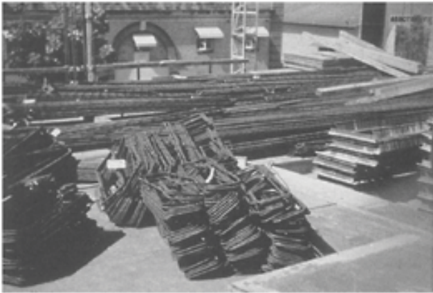
Reinforcement Stacked on the Formwork
