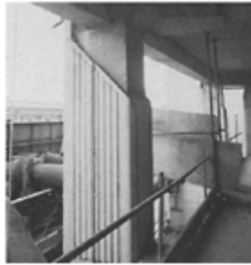
Precast Forms to all Column Faces
