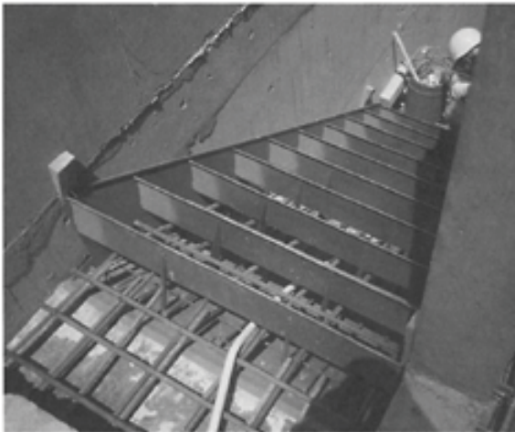
Sheet Metal Stair Form in Place
