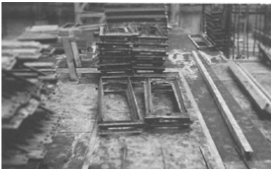
Components Stacked on the Formwork
