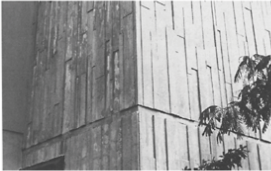
Wall from Timber Formface Varying in Thickness
