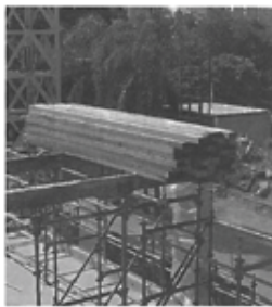
Material Stacked on the Formwork
