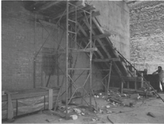
Strutting to the Sloping Soffit Form
