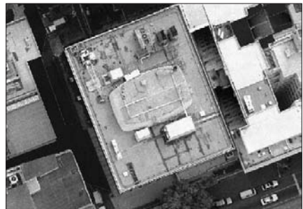
Fig. 24.2. Building roof top has been ortho-rectified although some minor rooftop structures have not been rectified.
