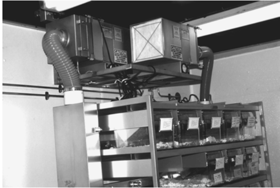
Figure 8.18 Upper portion of an individually ventilated microisolation cage rack showing the cage supply and exhaust filter and blower units sitting on a wall-mounted shelf. This arrangement facilitates rack changes by eliminating the need to transfer the filter and blower units from rack to rack.
