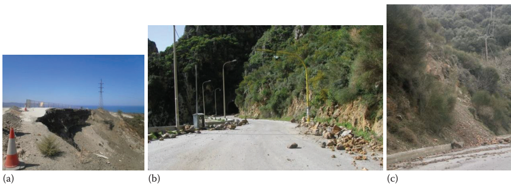
FIGURE 23.6 Different types of earth displacement affect transportation networks: (a) embankment failure in Cyprus; (b) rockfall events interrupting traffic at Topolia Gorge, Crete, Greece; and (c) small-scale landslide may be as destructive as large ones.
