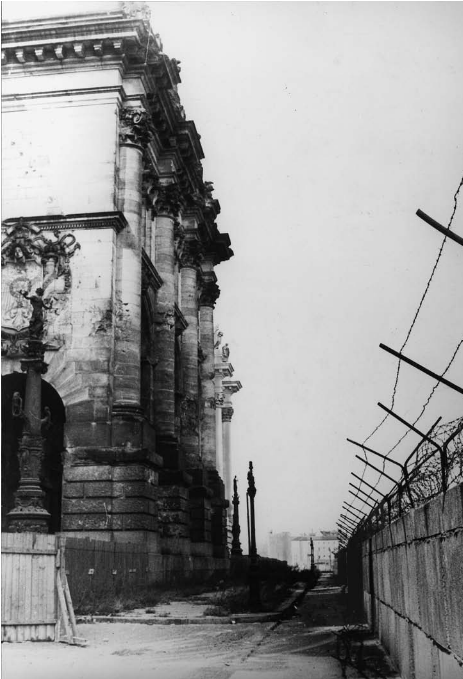
Figure 2.7 The Reichstag and the Berlin Wall during the Cold War. In the later years of a divided Berlin, the Reichstag (left) was a few metres into West Berlin. This photograph dates from the first era of the Berlin Wall, 1961–1964, when it was a structure of rough-cast concrete blocks topped with barbed wire
