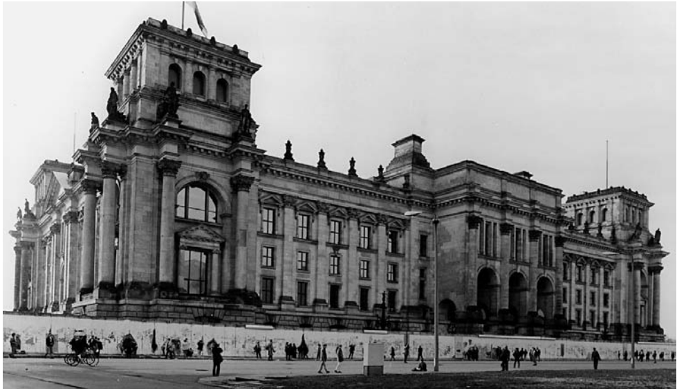
Figure 2.8 The Reichstag and the Berlin Wall soon after German reunification in 1989. In its final form, the Berlin Wall was a smooth-faced wall of cast-concrete segments topped with a curved asbestos–cement pipe. The West German side was famously covered with spray-painted graffiti, the East German side kept in neat order by the border police. As this photograph taken from the east soon after German reunification shows, the east side of the wall was immediately also covered in graffiti. Segments of the pipe topping to the wall have been removed, and there are holes hacked through it
