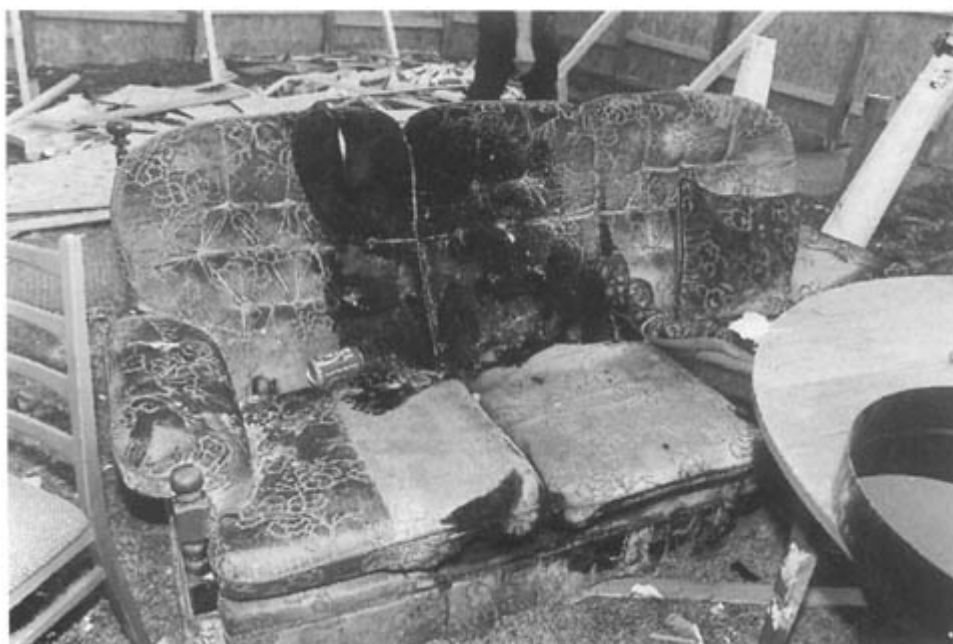
Figure 7.14 Secondary fire initiated by the deflagration of a gas/air mixture.
