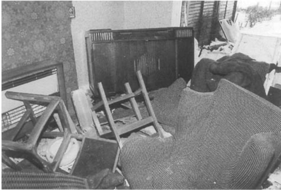
Figure 7.15 Chairs overturned by the upwards displacement of the floor.
