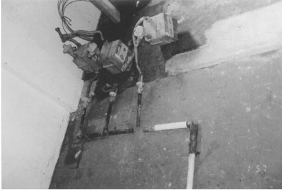
Figure 7.23 Reconstruction of new service pipe manifold and three gas meters.
