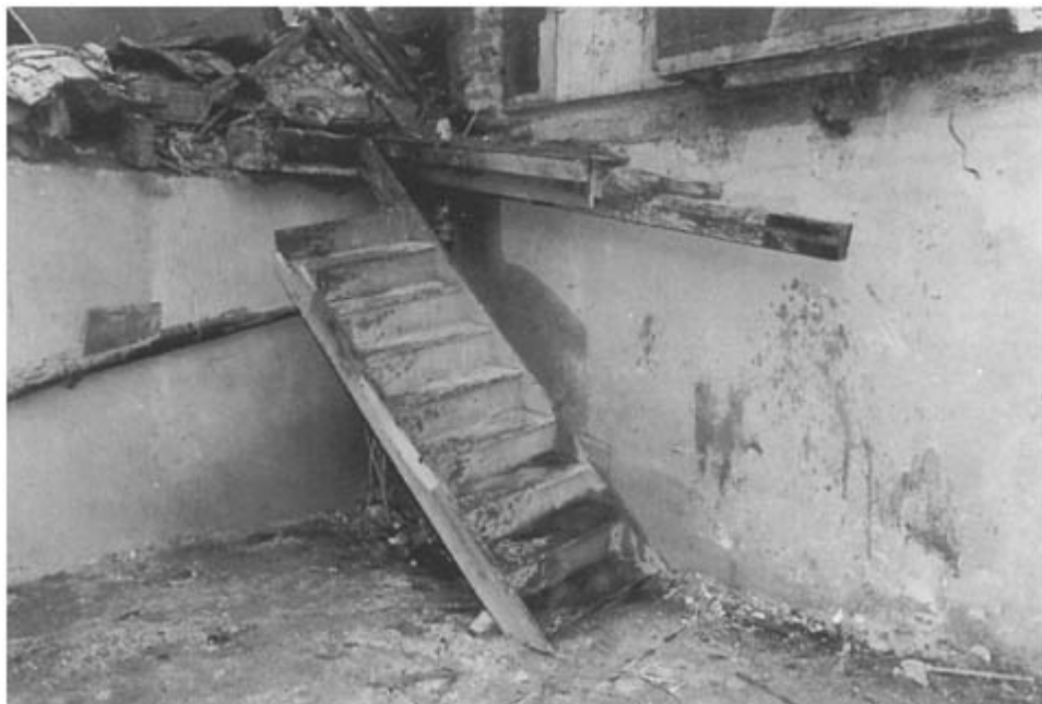
Figure 7.20 Reconstruction of basement stairs.
